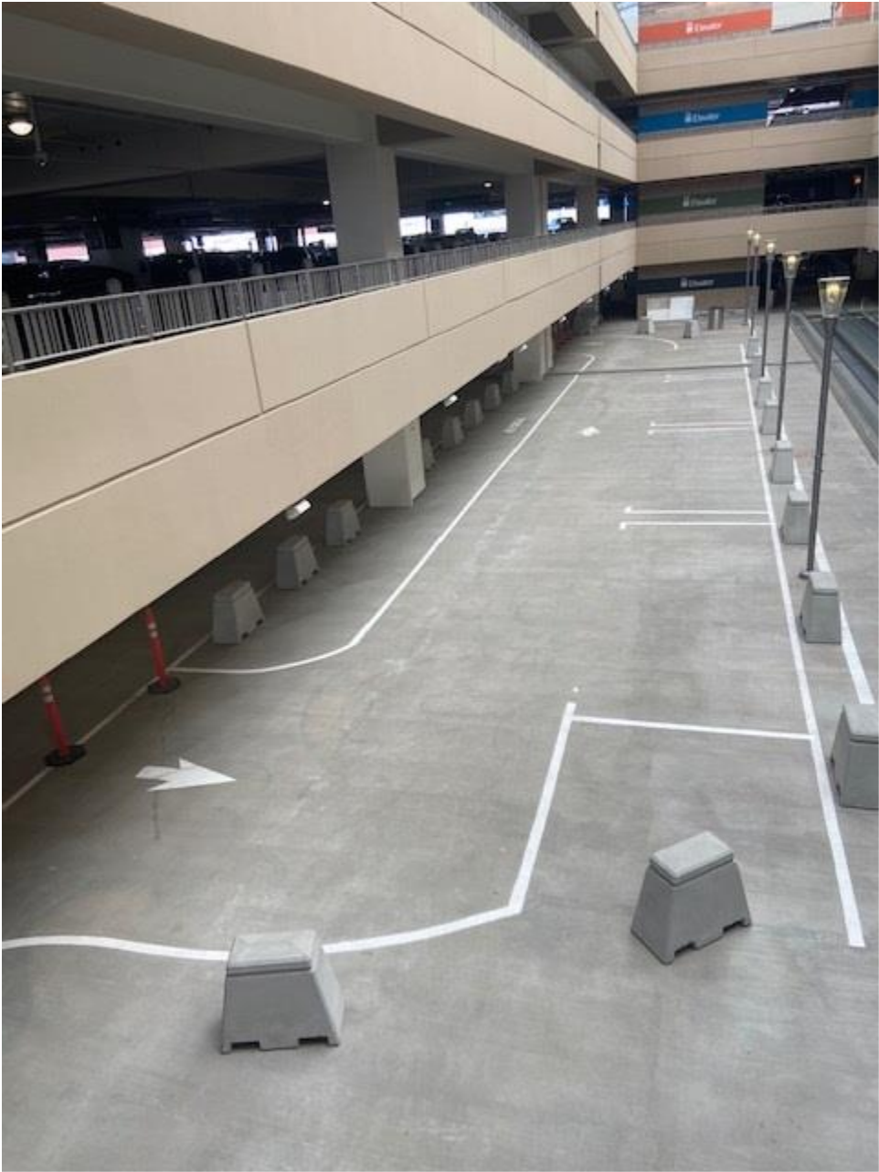
Images 5: Overhead view showing drive thru lane and drop off areas.
