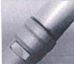
3. Before inserting a spigot end into the socket, it is recommended to mark the insertion depth on the spigot. See insertion Depth 'A' from chart on page 6.
