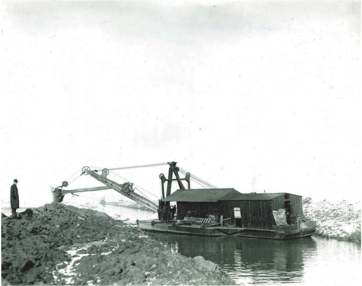
Figure 6. Dredging of the Surplus Canal. Believed to be the City Dredger (Utah State Historical Society, Photo 24676, dated 1913-06-13). While the photo is dated June of 1913, the snow seen in the photo clearly indicates the photo was taken in winter and was most likely taken during the 1910-1911 construction season.
