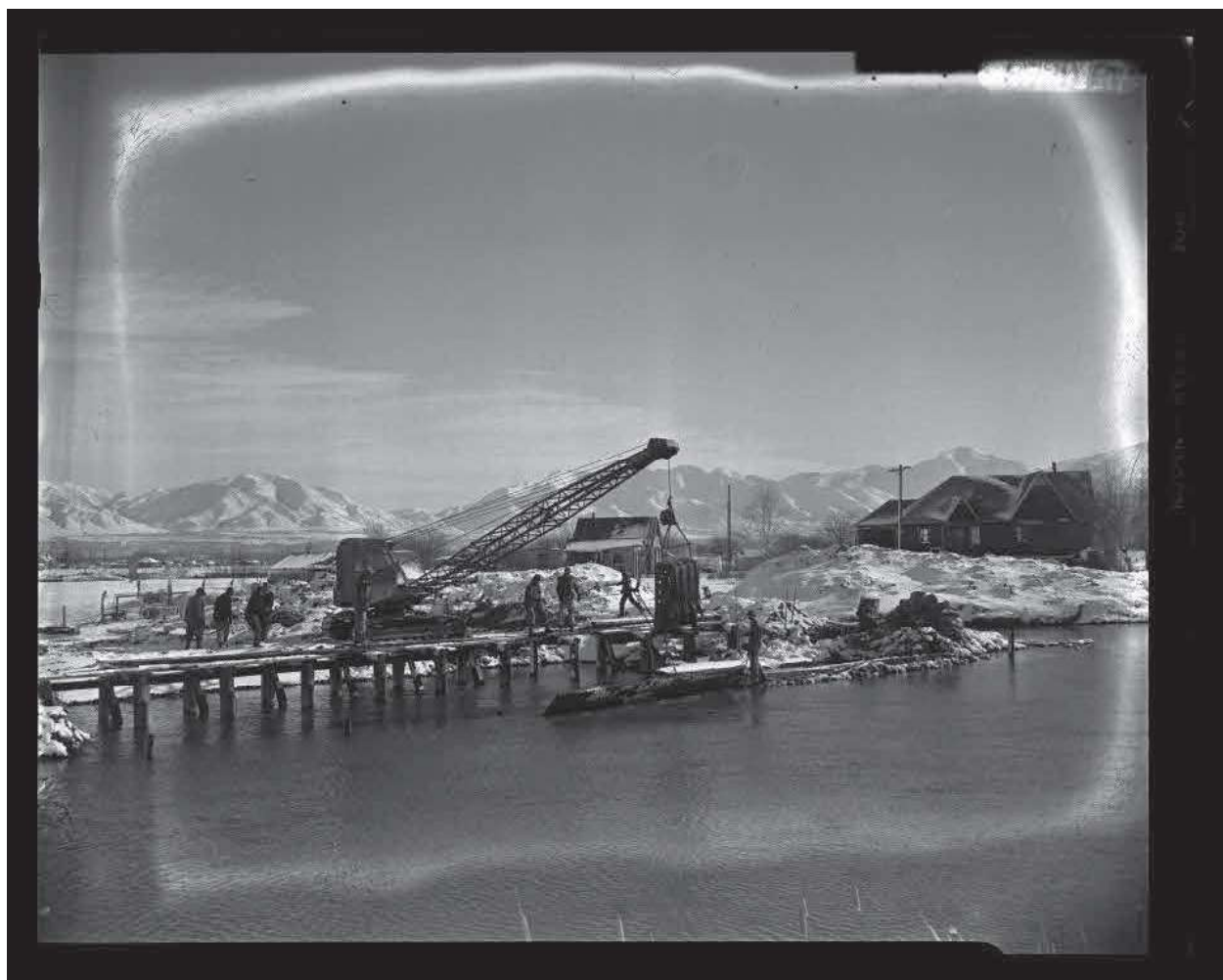
Figure 8. Construction of a new diversion structure for the Jordan River Surplus Canal, 1952-01-14 (Utah State Historical Society Photo 10547).
