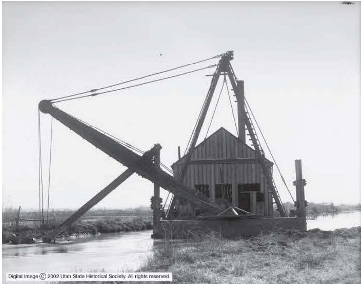
Figure 5. Dredge working on the Jordan Surplus Canal in 1910. Believed to be the Utah Sand, Dredging, & Construction Co. dredger that first started work (Utah State Historical Society, City Engineers Photo 01537).
