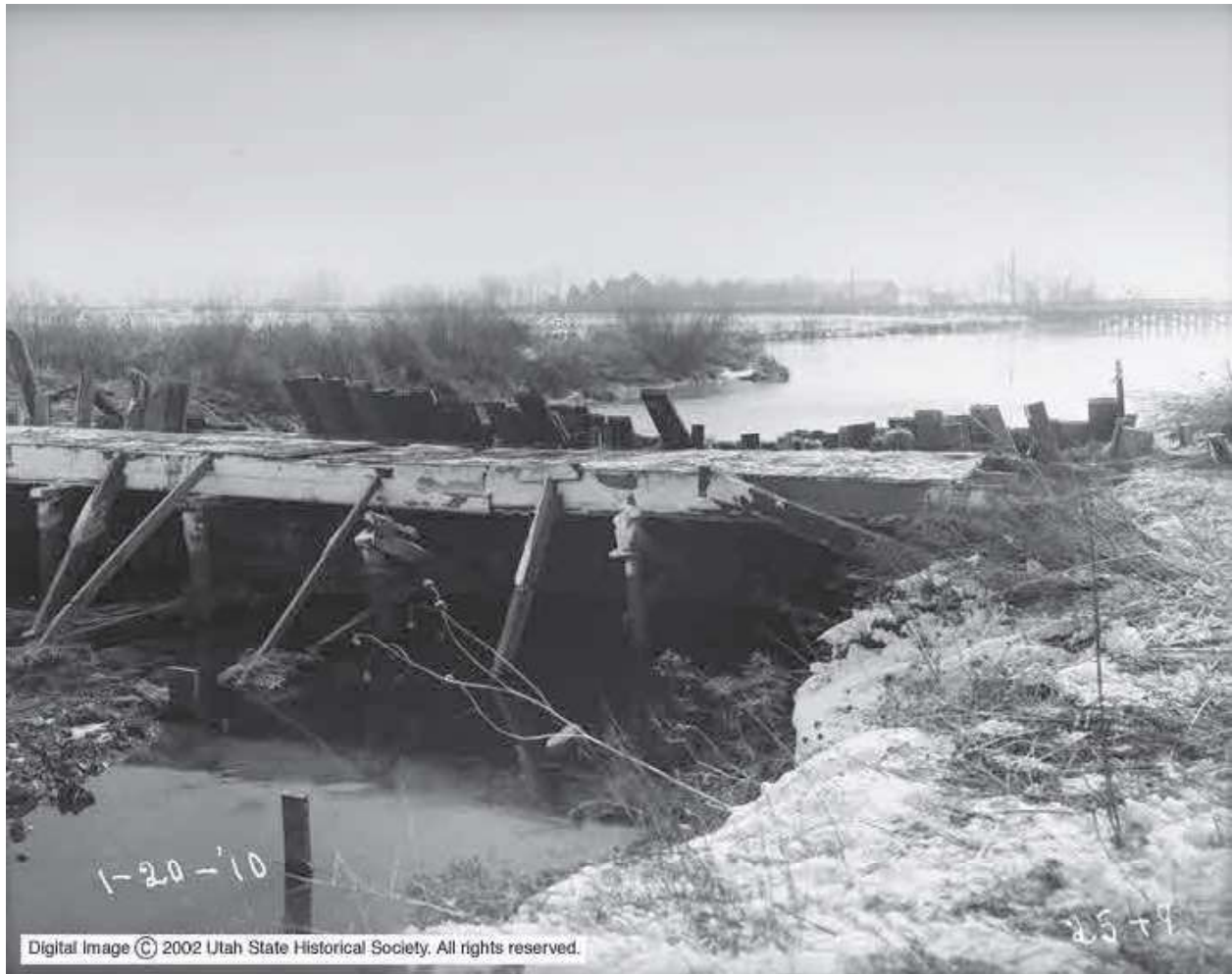
Figure 3. Dam at the head of the Surplus Canal at its junction with the Jordan River (1910-01-20; Utah State Historical Society, City Engineers Photo 01531).
