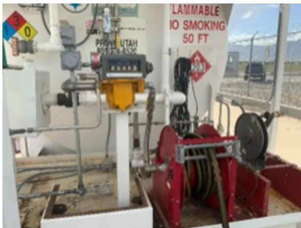
Completion of the new meter at the KTVY 100LL self-serve tank
