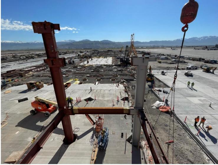
The first steel beam has been raised on Phase 4 of The New SLC. This phase will add 16 gates--for a total of 94 gates--to Concourse B-east by 2026.
