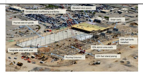
The focus of TRP construction remains the car rental area Quick-Turn-Around (QTA) facility. To date, 55% of the foundation and shear walls have been cast, 93% of the structural columns have been cast (192 of 206) and 60% of the concrete slab has been poured. Work continues on the administrative area, mechanical rooms, foundation walls and sump installations. In addition, site utilities are being developed, parking and roads are being formed and the elevated deck is being erected.
