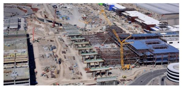
The Elevated Roadway is taking shape as the concrete girders are put in place.
