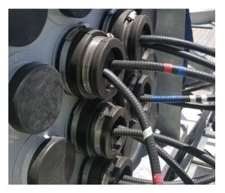
c. Boot assemblies shall be Commscope 4" Boot Assembly (p/n 294573) with the appropriate Commscope boot insert for the required number and size of holes to match the number and size of cables.
