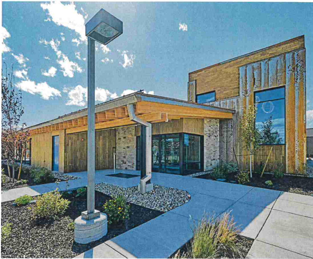
Big-D led work on the National Ability Center's Equestrian Center expansion in Park City.
