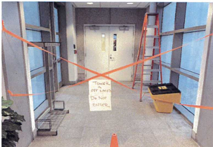
The tower closed off for damage assessment
