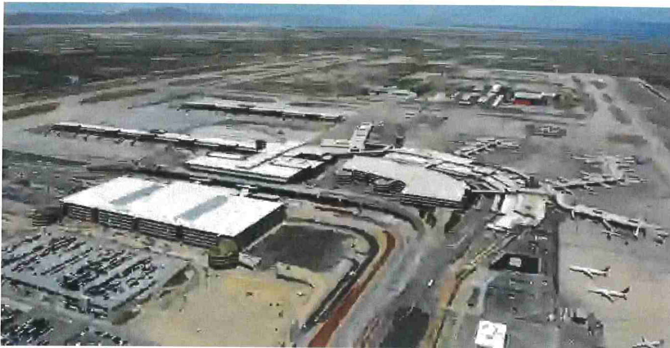
An aerial view of the Salt Lake City airport with the new terminal and satellite concourses on the left, and the old terminal complex on the right. (Photo courtesy of the Salt Lake City International Airport)
