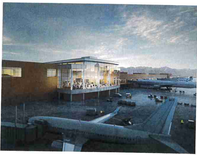
The new terminal opens to the public Sept. 15. (Photo courtesy of Salt Lake City Airport)
