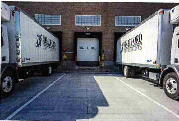
(Trent Nelson | The Salt Lake Tribune) The Salt Lake City Airport's new Central Receiving and Distribution Center (CRDC) on Tuesday, Aug. 11, 2020.
