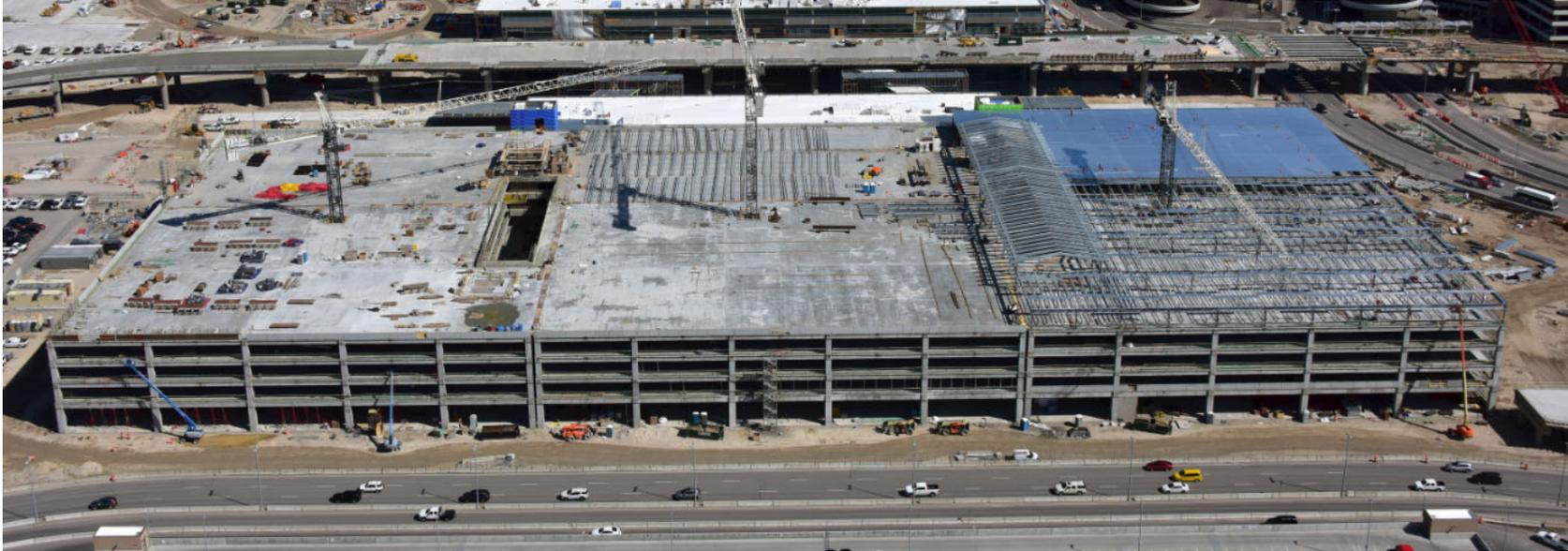
Parking Garage looking north – Steel Erection Progressing East to West
