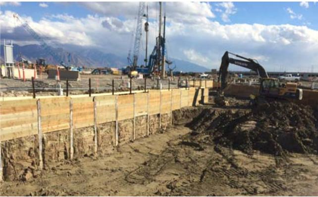
Tunnel Excavation and Lagging Wall
