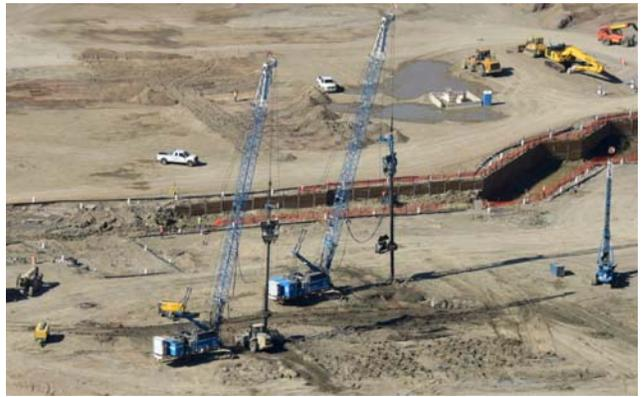
Last of the Stone Column foundation installation.
