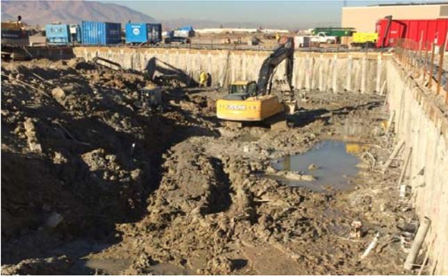
Excavation cutting back before digging down to the next depth.
