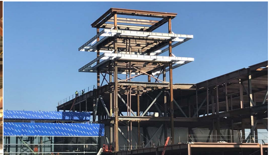
Ramp Tower Structural Steel Erected
