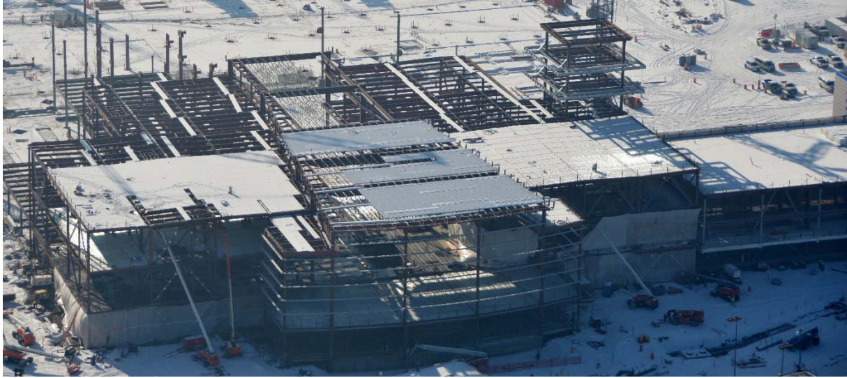
Terminal structural steel and metal decking, viewed from the north
