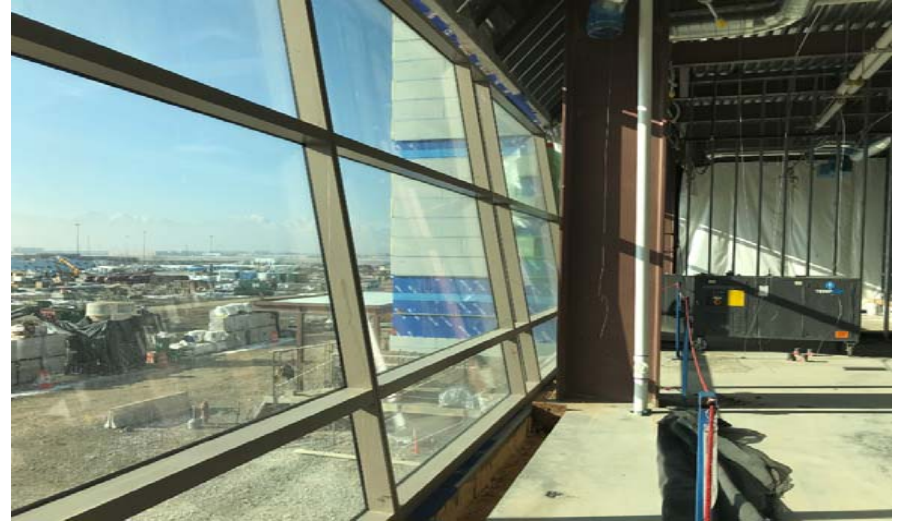
SCW south sloped curtain wall from the interior
