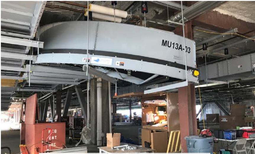
SCW baggage conveyor installation
