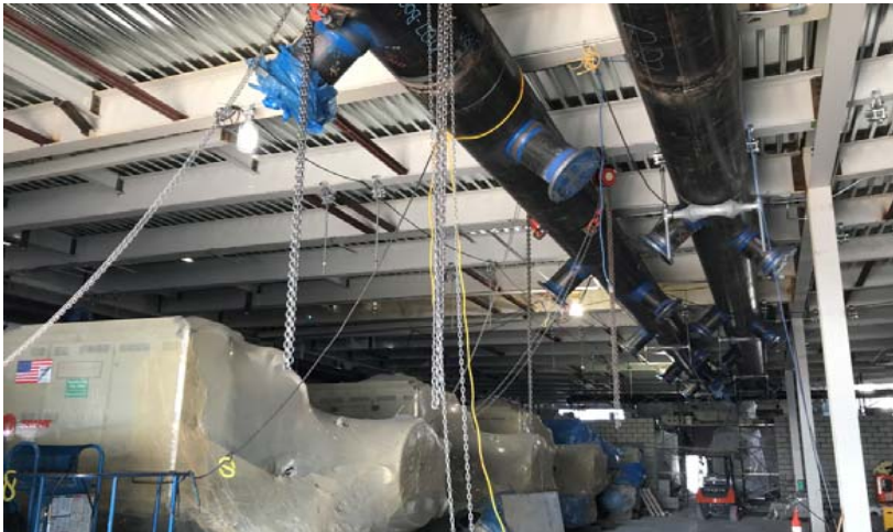
Large diameter Chiller piping installation progress (CUP)
