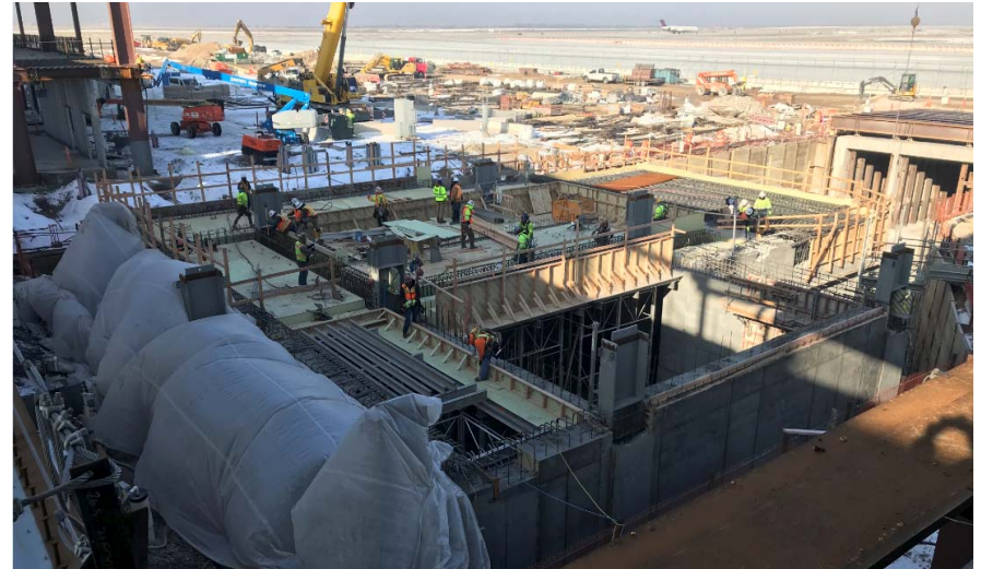
Construction at Mid-Concourse Tunnel
