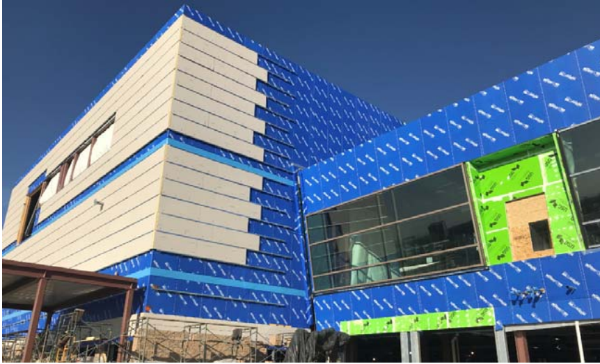
SCW curtain wall, sheathing, insulation and masonry
