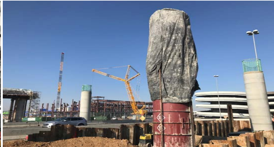
Roadway columns constructed between exit roads
