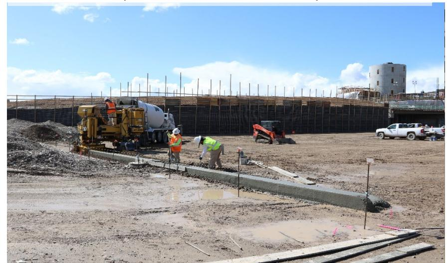
E Lot Curb & Gutter Concrete Placement
