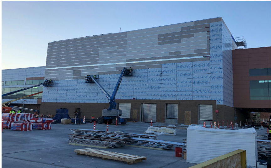
North Concourse Sector CN Metal Panel Installation
