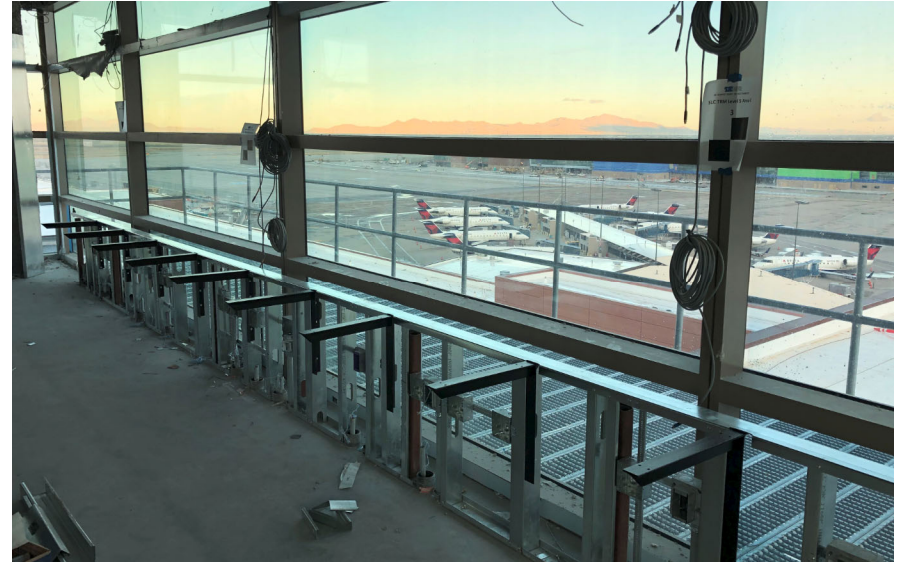
Terminal Ramp Tower Counter Framing
