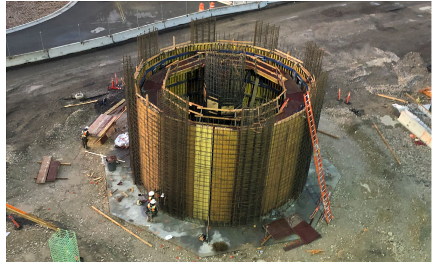
Parking Garage West Helix Formwork
