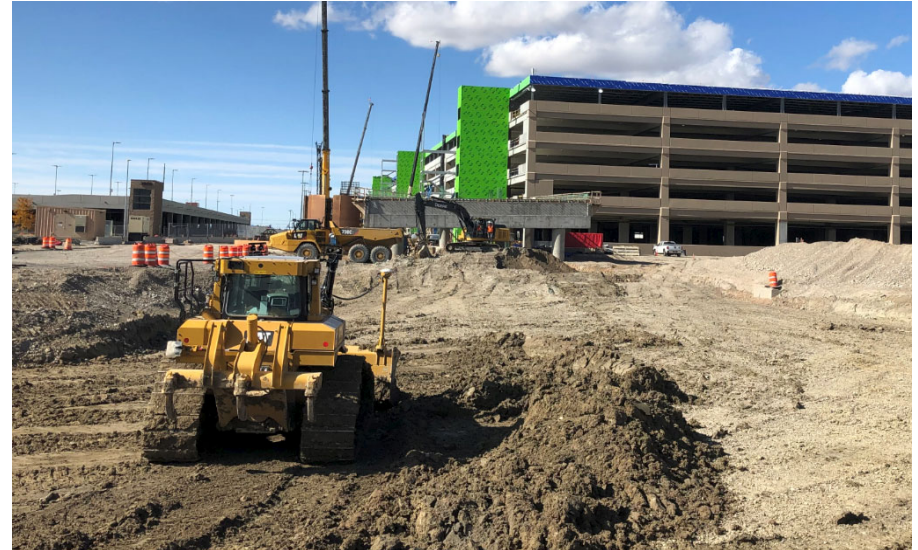
Parking Garage Entrance Road and Plaza Excavation & Grading
