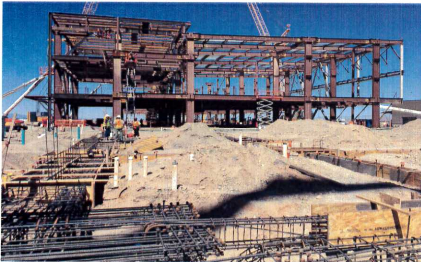
South Concourse West steel erection (background) and east area foundations (foreground)
