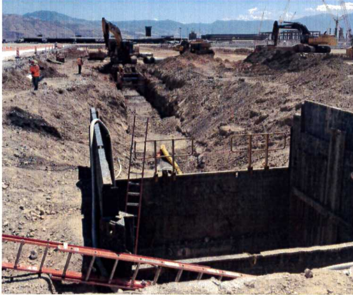
Storm sewer installation under Taxiway 20
