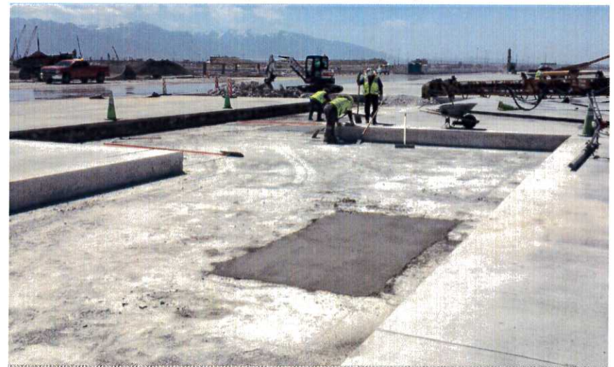
Repair to the soil cement base under Taxiway B
