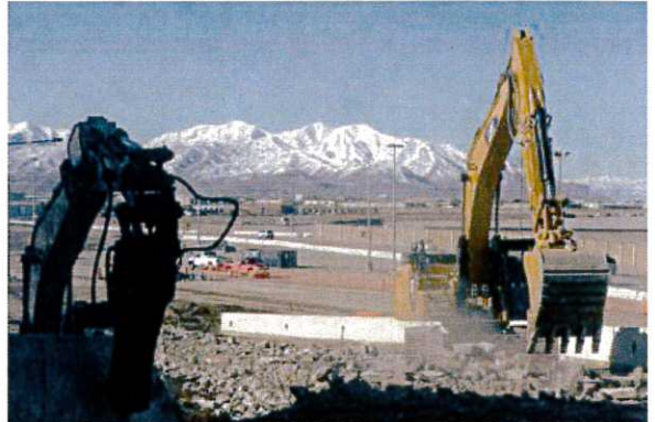
(Rick Egan | The Salt Lake Tribune) Excavators demolish the exit ramp to what was previously the drive-through lane of the Salt Lake International Airport's short-term parking garage. The exit ramp area, as well as what formerly housed car rental canopies will become a new roadway exiting the airport the summer of 2016 to prepare for future construction projects at the airport, Monday, February 22, 2016.
