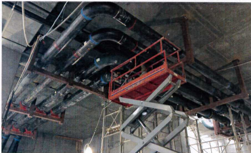
Terminal Tunnel installation of hydronic piping
