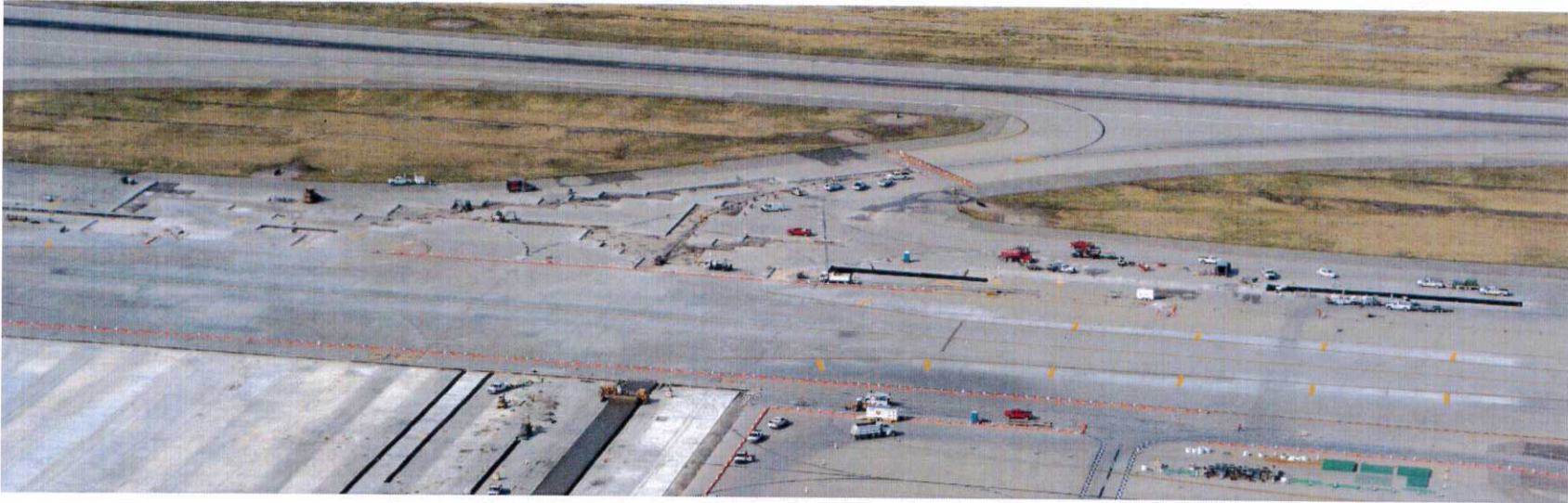
Taxiway 'A' paving and lighting reconfiguration in progress.
