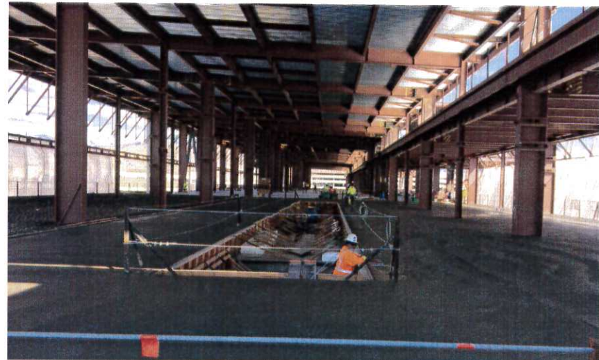
SCW Level 2 elevated deck concrete finishing
