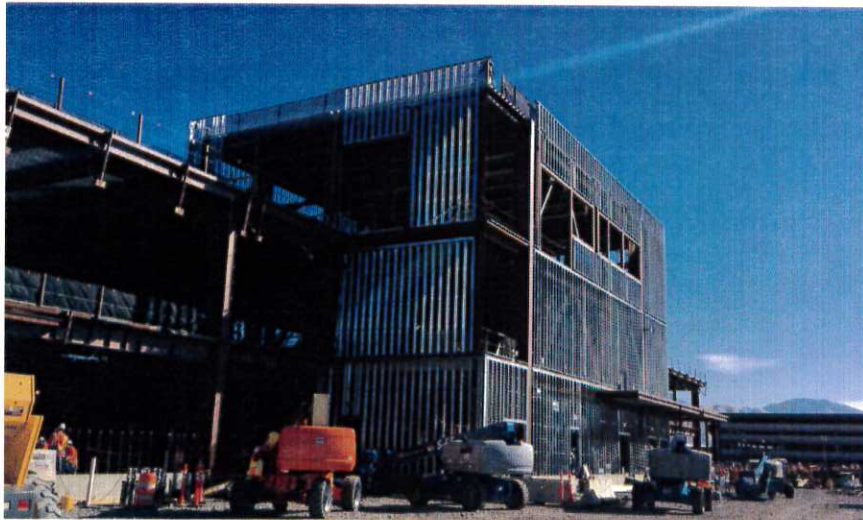
SCW exterior wall system installation in progress
