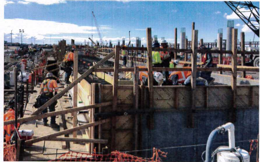
Preparations for the final Terminal Tunnel lid pour.
