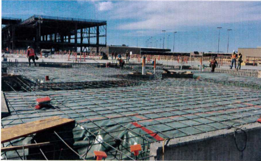
Installing rebar for critical Terminal Level 1 Area 'D' slab
