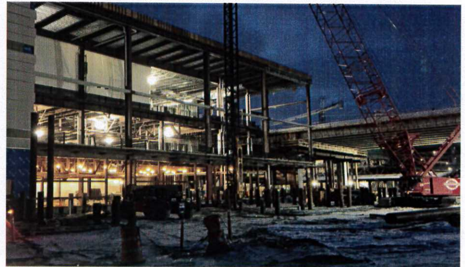
Terminal Expansion – Pile Installation
