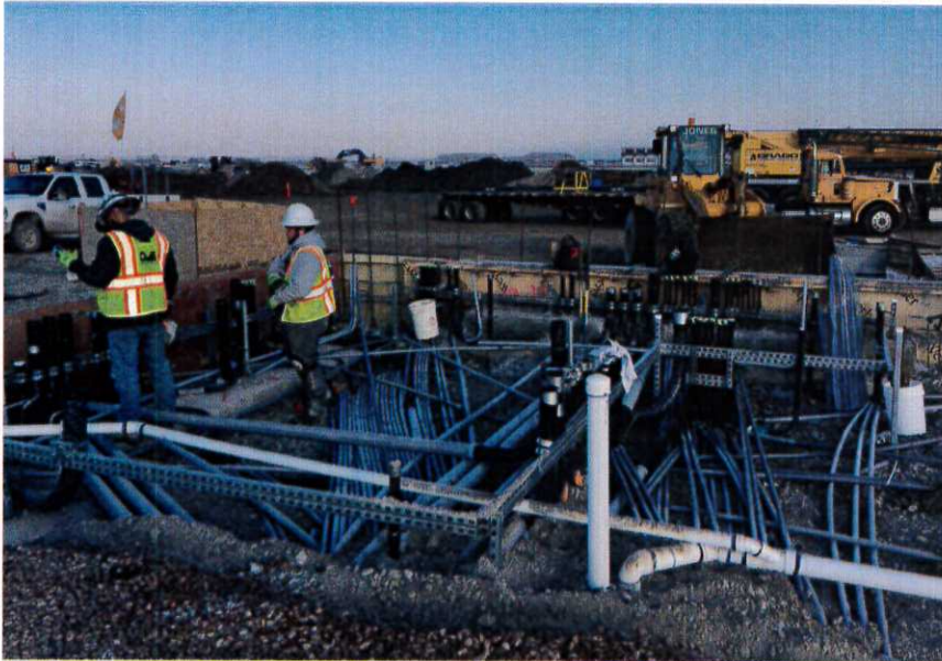
NCP Sector 'E' Electrical Room
