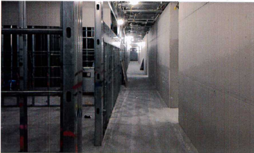
SLCDA Offices in Terminal Level L3
