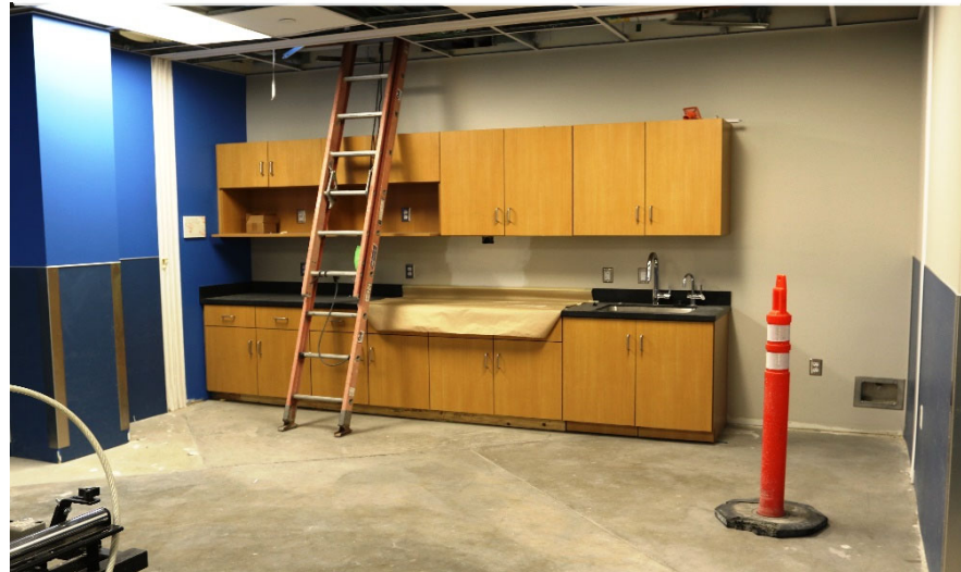
North Concourse Level 1 American Airlines Breakroom
