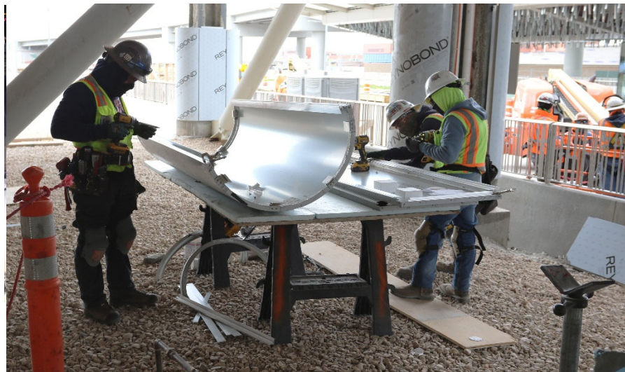
Gateway Level 1 Exterior Column Covers
