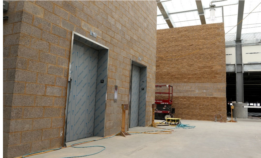
Parking Garage Passenger Elevators
