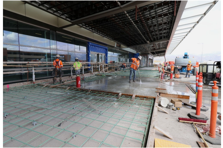
Roadway Departures Level Sidewalk
