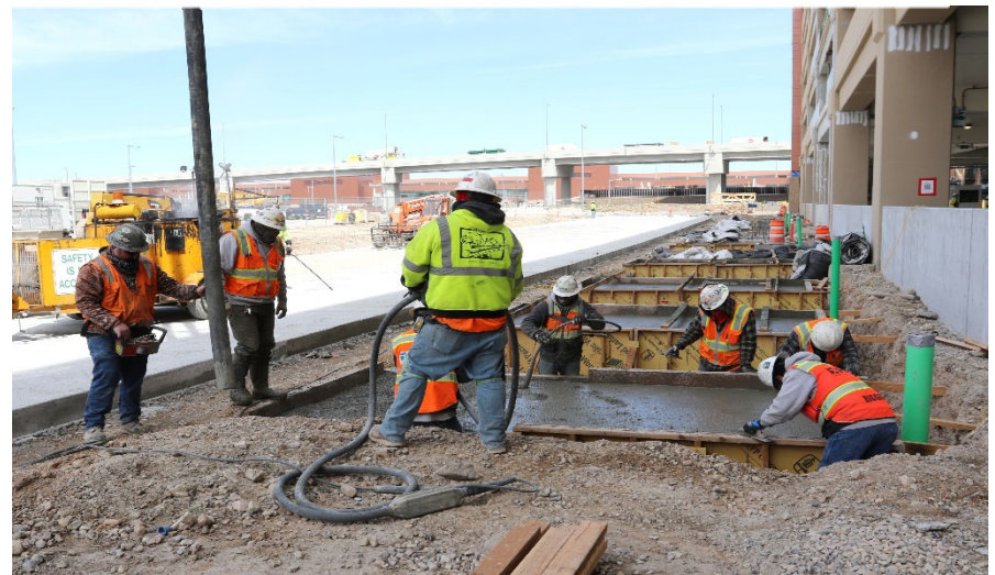
Off-site Rental Car Shuttle Area Canopy Foundations
