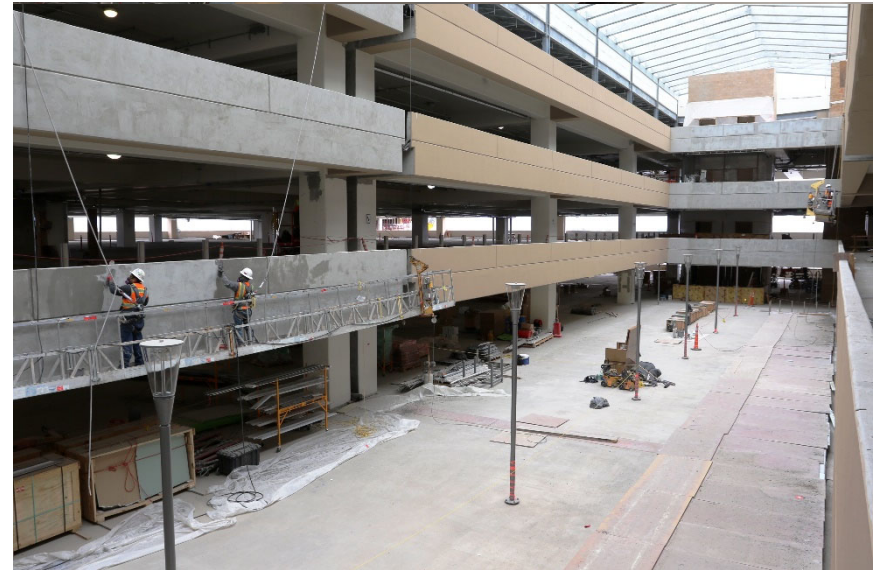
Parking Garage Pedestrian Corridor Patching & Painting
