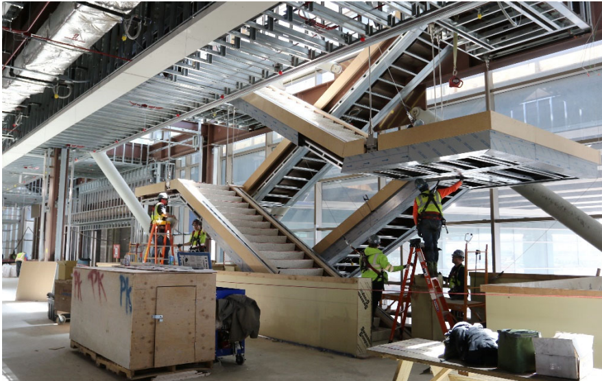
Terminal Entrance Level 2 Stairwell
