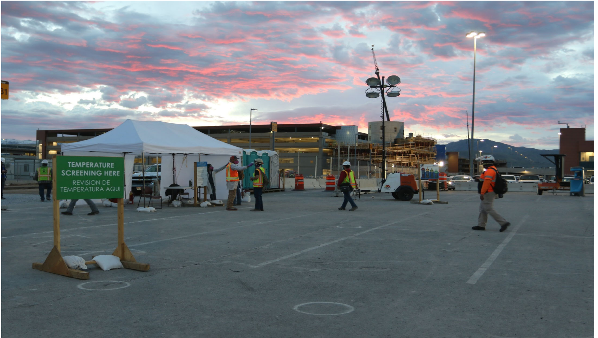
Trade Worker Site Entrance Temperature Check Station
