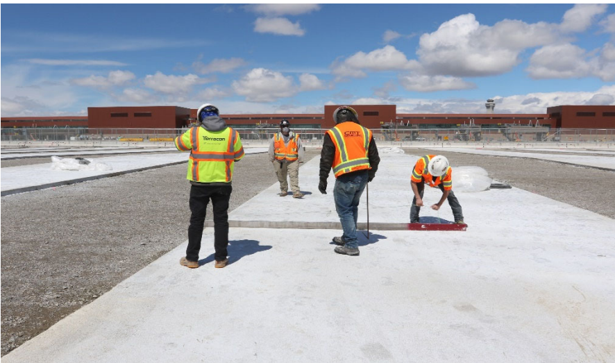
SCW North Apron Lean Concrete Straightness Testing
