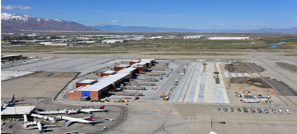
North Concourse & North Apron Looking west
