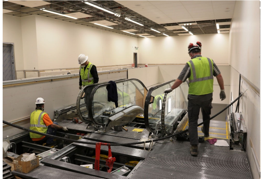
North Concourse Level 2 Mid-Point Escalators
