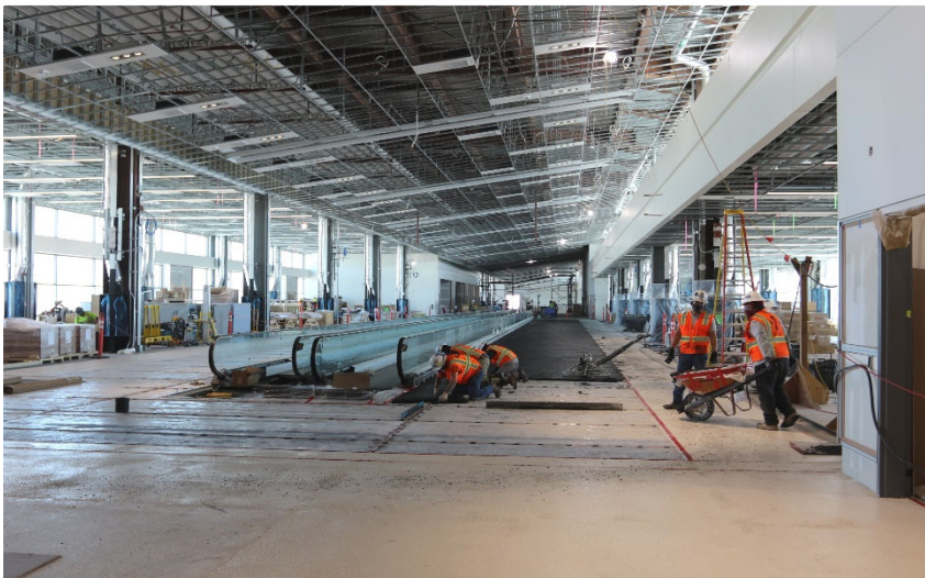
North Concourse Level 2 Terrazzo Installation
