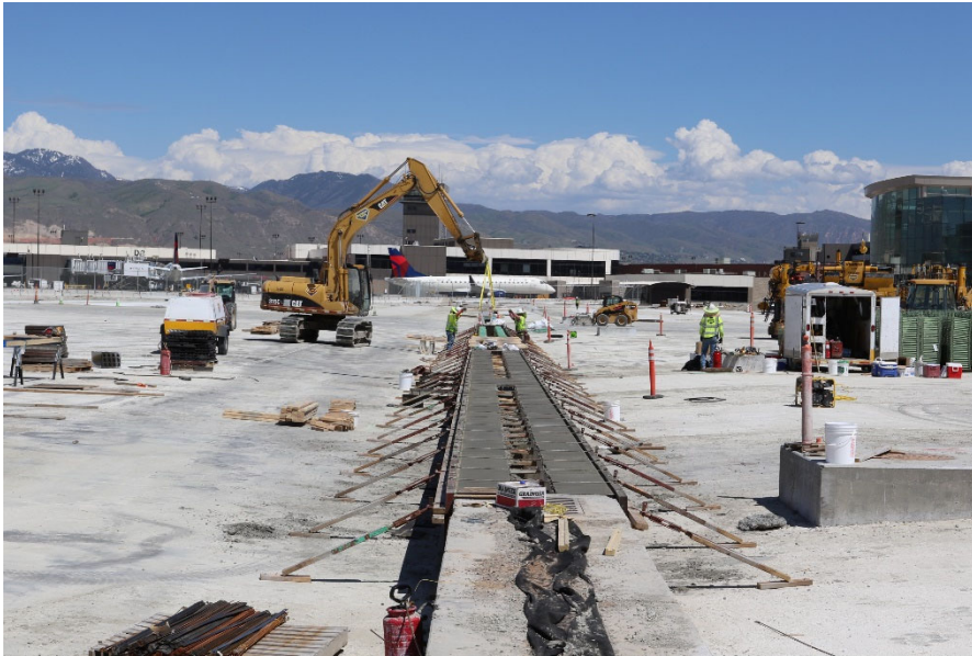
SCW North Apron Trench Drain installation
