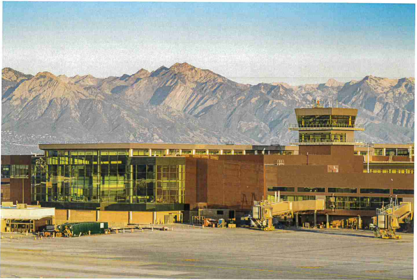
Photo: Salt Lake City International Airport
