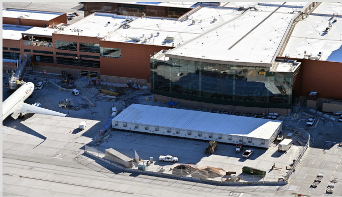
BHS Exp - TSA Temporary Trailer Complex
