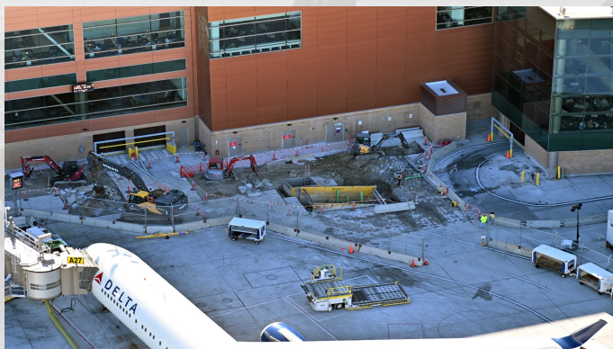
BHS Exp - Start of Building Expansion
