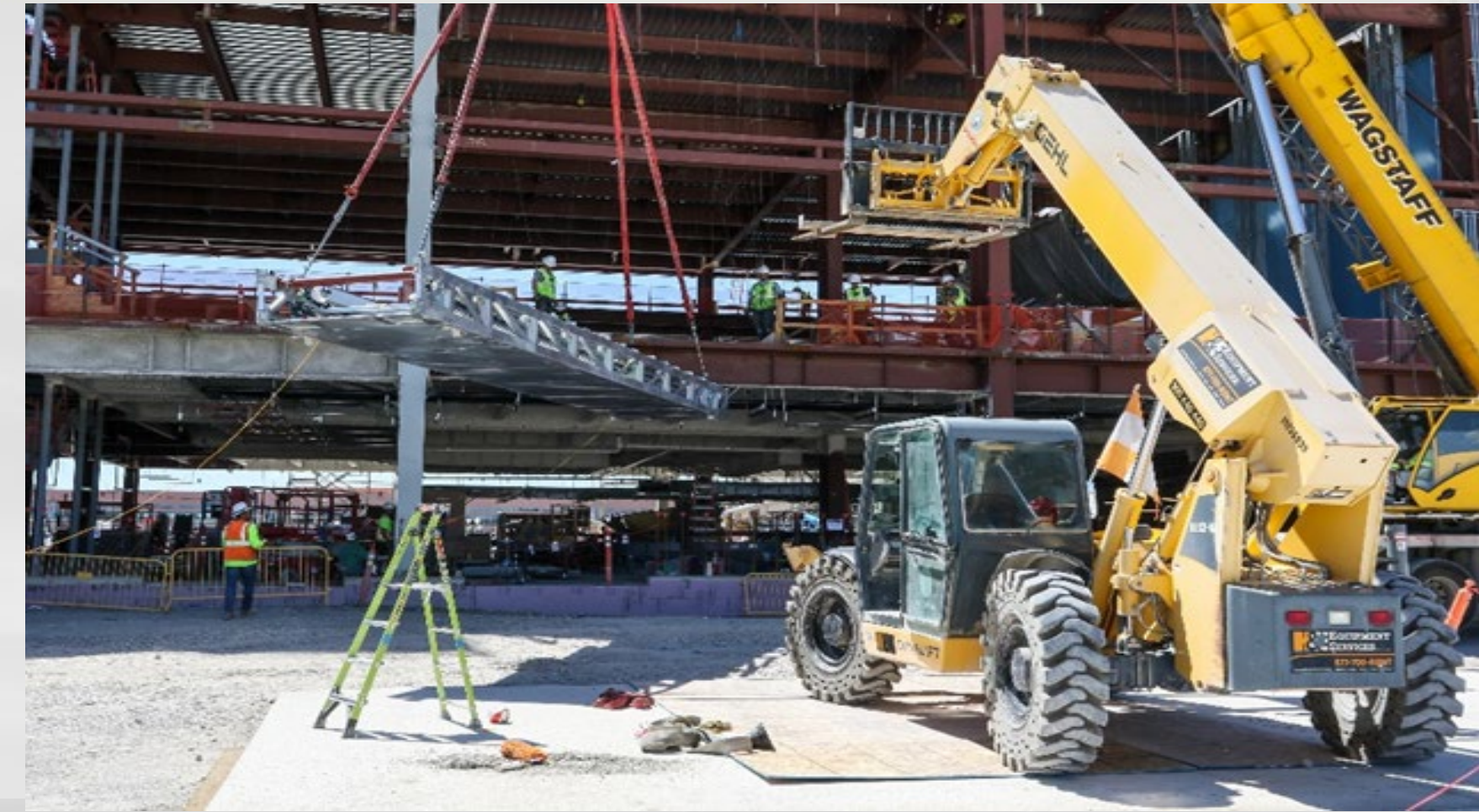
Hoisting Moving Walk into Phase 4
