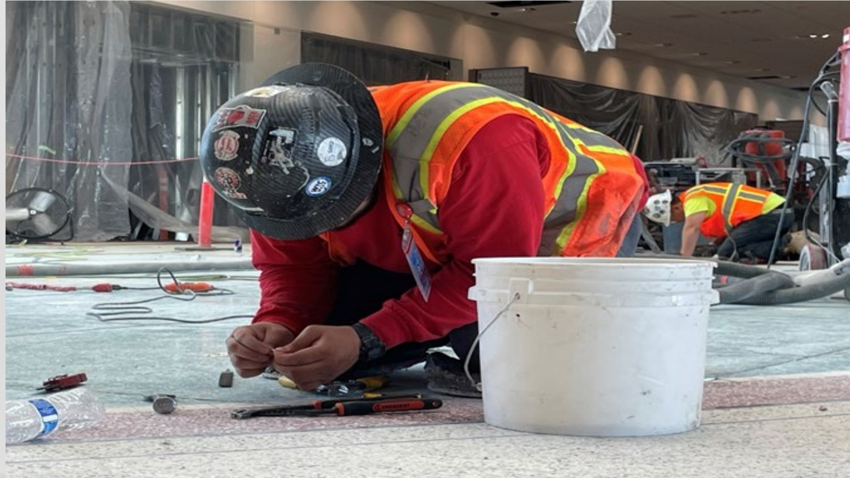
Repair of Metal Divider Strips
