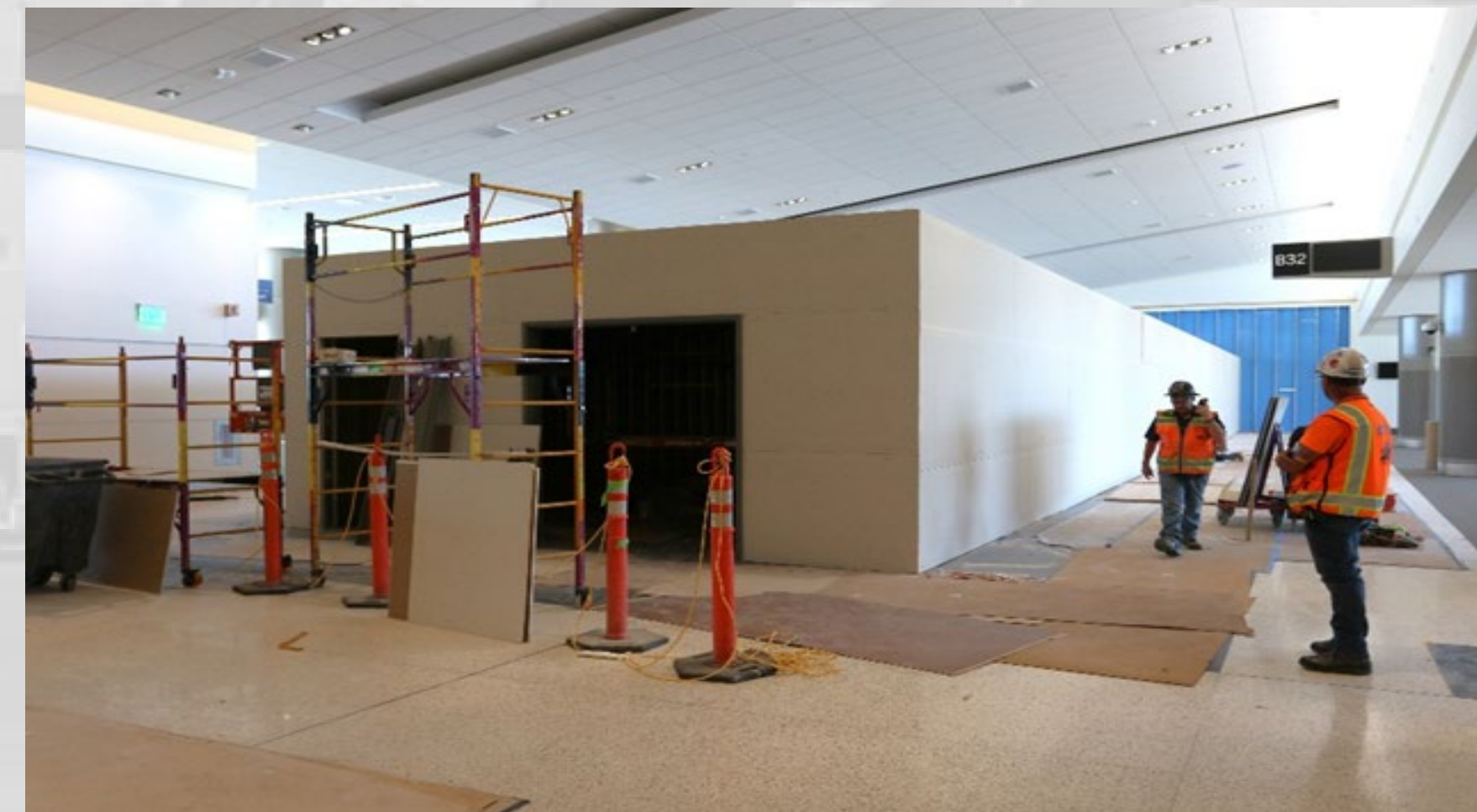
Completed Moving Walk Enclosure
