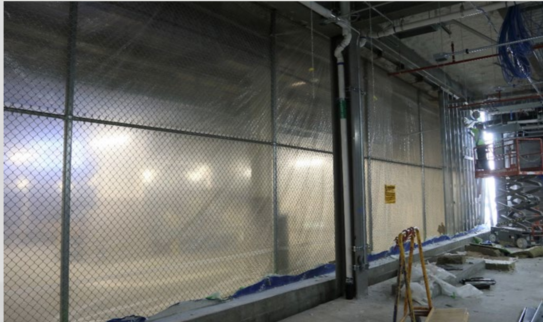
Lvl 1 Separation Bagroom and Construction
