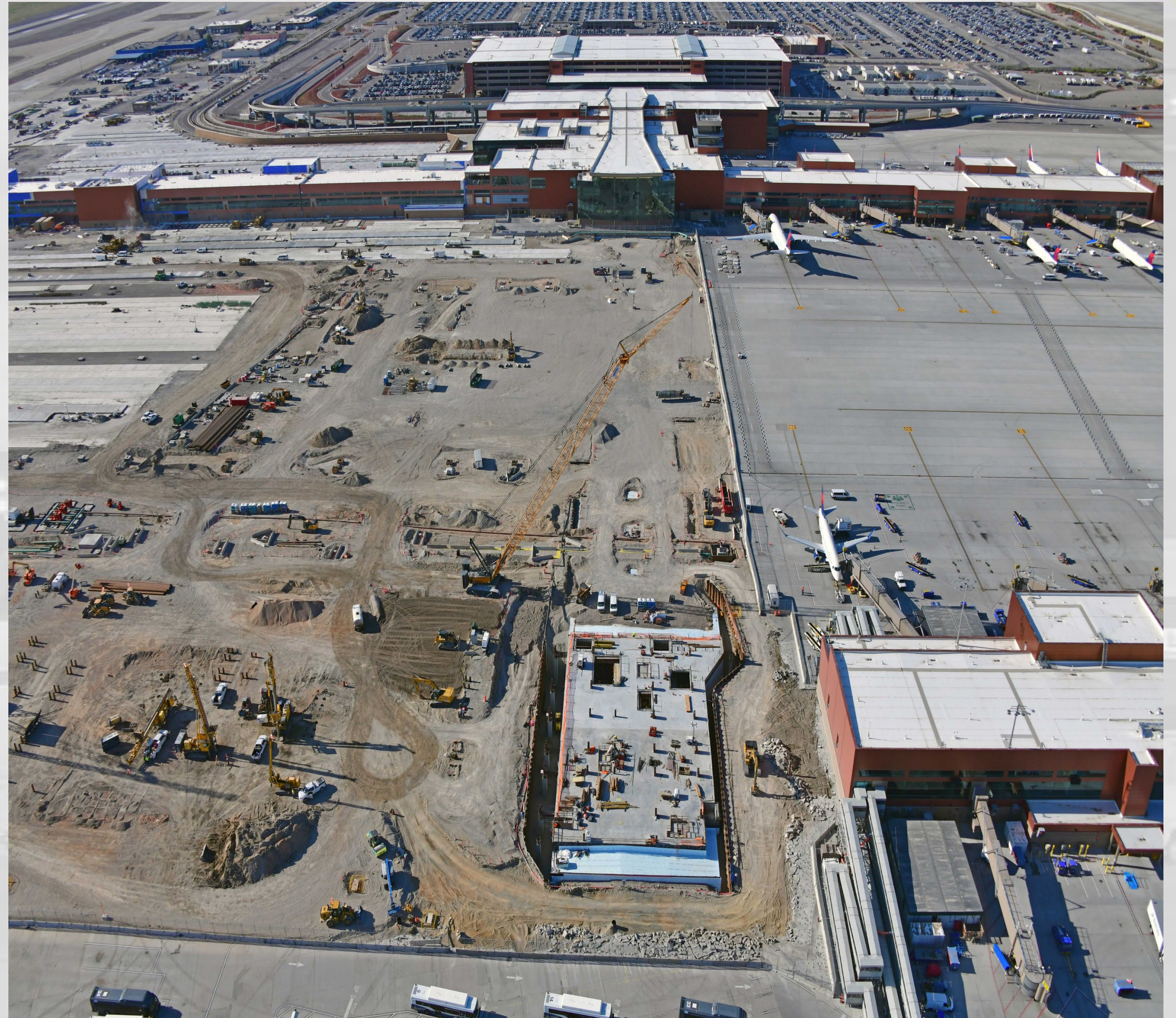
Central Tunnel Topside
