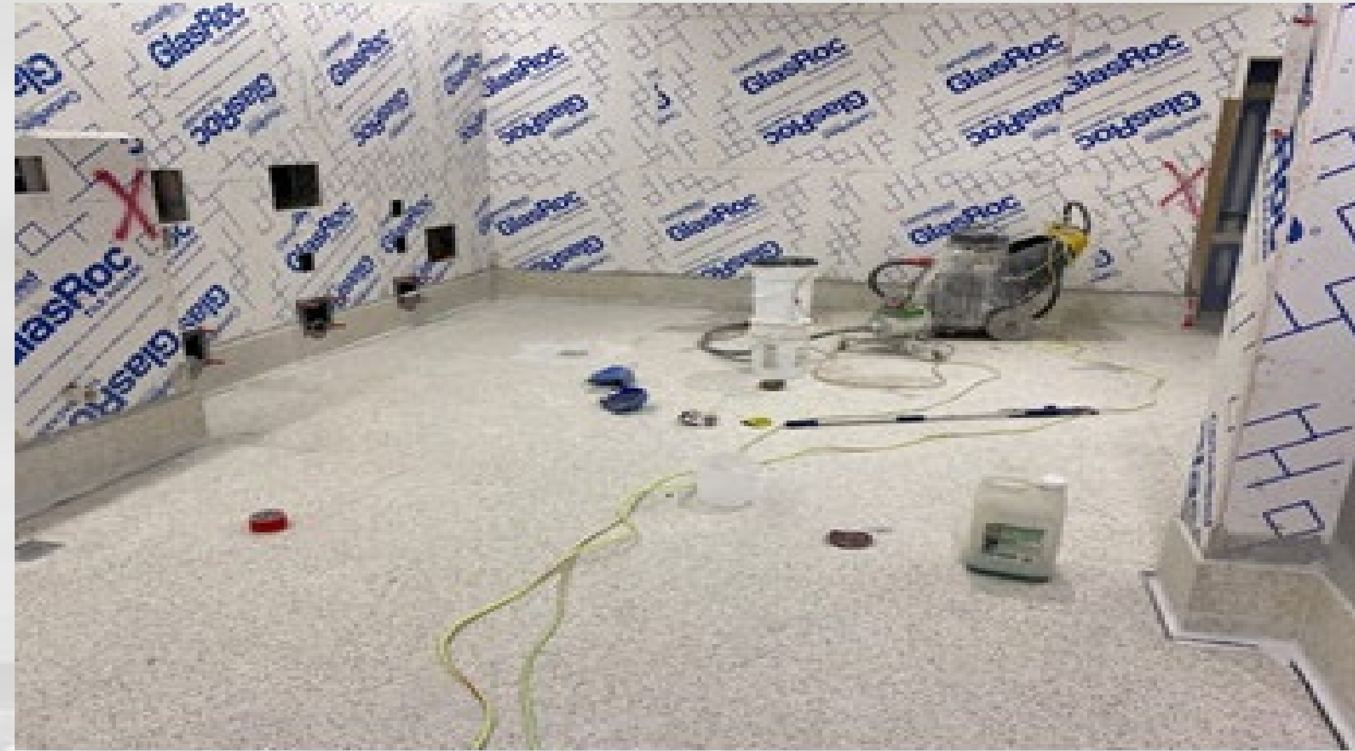
Level 2 Area A Restroom Terrazzo
