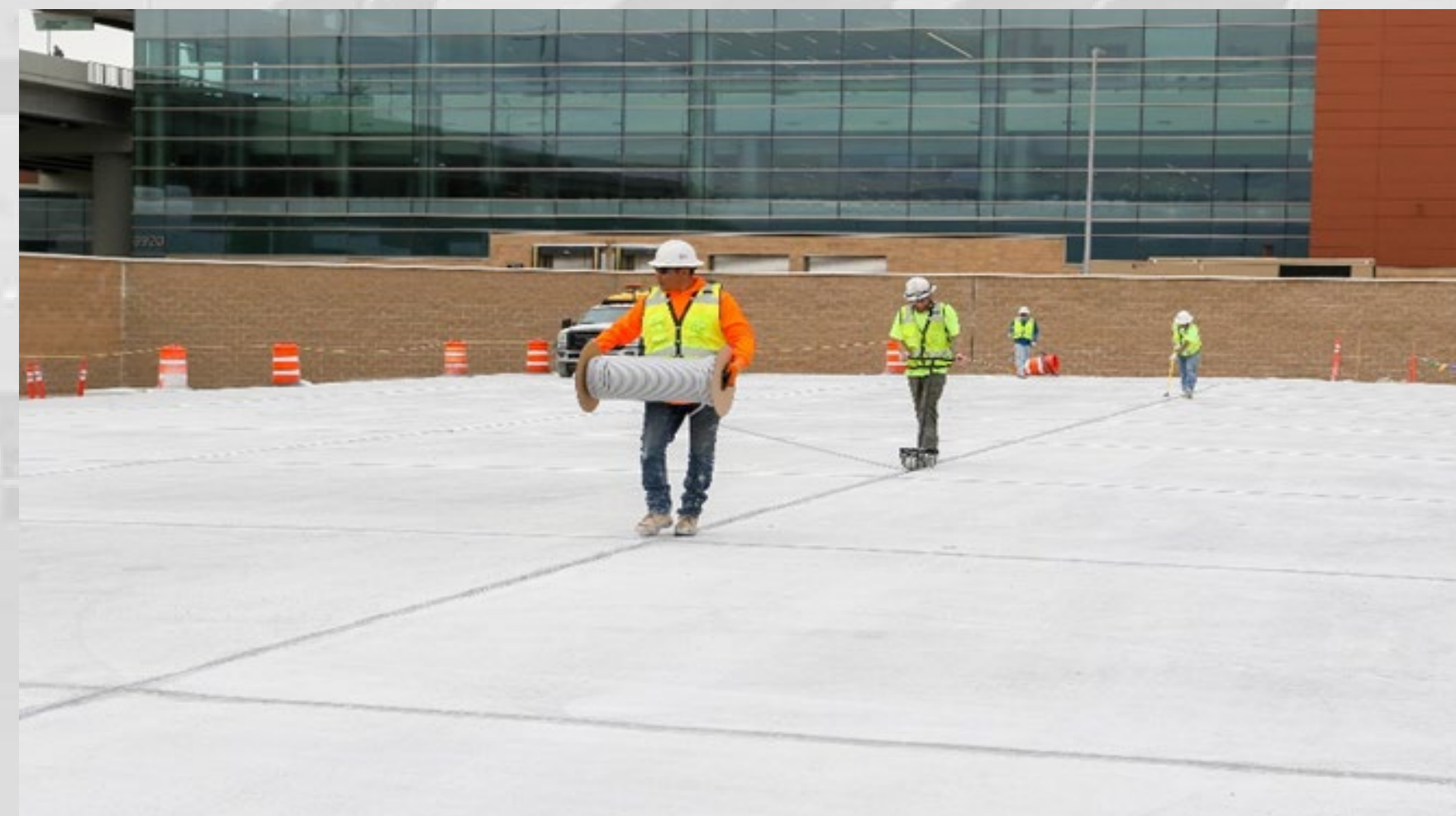
Apron Joint Sealing
