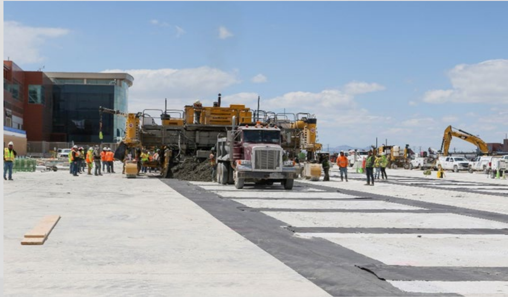
Paving North Side of Concourse 'A'
