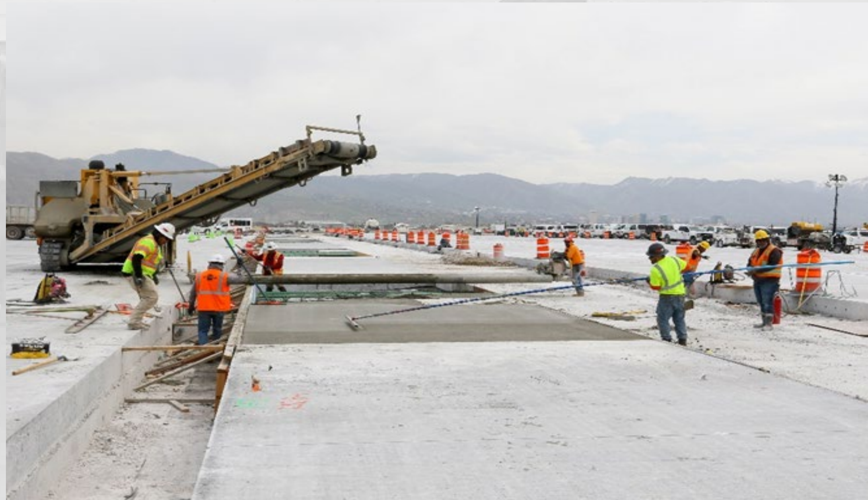
Paving South Side of Concourse 'A'
