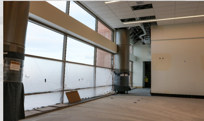
Gate A33 Vestibule – 5 th Early Gate
