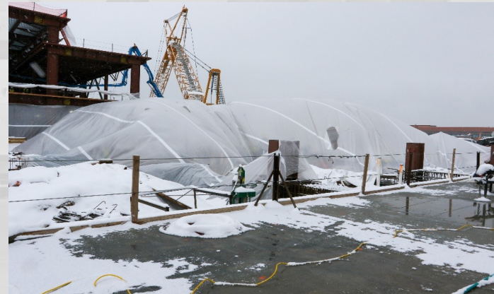
Area G East Shallow Fdns - Weather Protection
