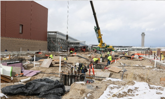
Area G Shallow Foundations
