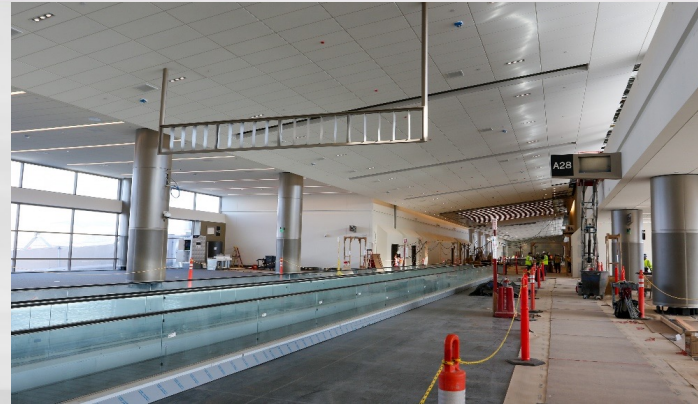
Overhead Sign Supports Area B
