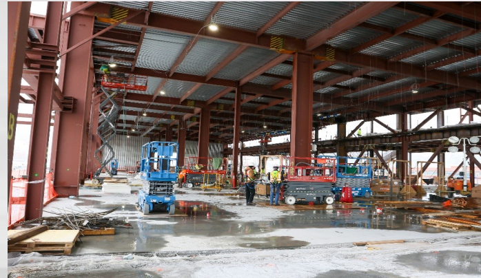
Level 2 Area J Framing
