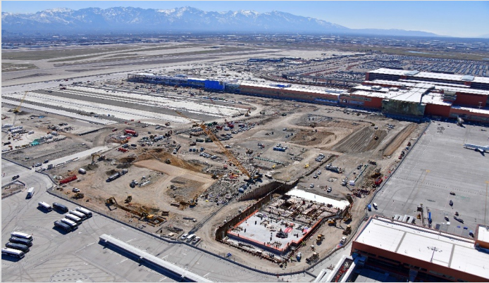
Site Grading Begins 03/2022
