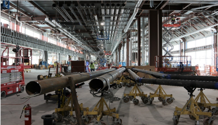
Level 2 Area B Looking West 04/2022
