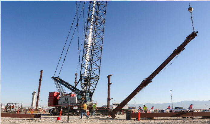
Steel Erection Day One 09/07/2022
