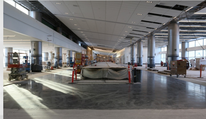
Level 2 Area B Looking West 12/2022
