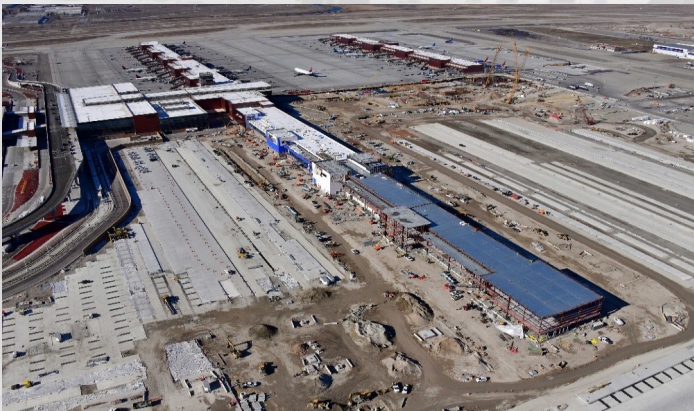
Concourse A East 01/27/2022
