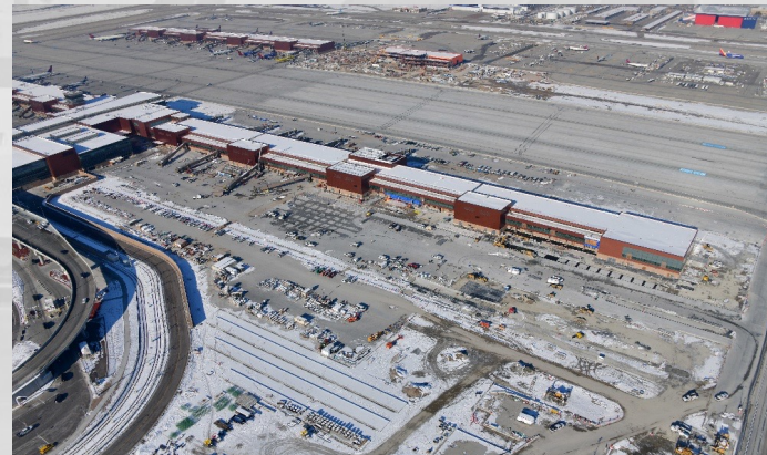
Concourse A East 12/19/2022
