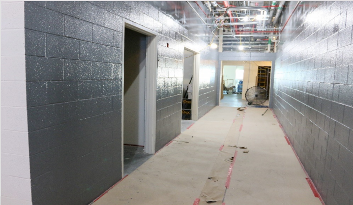
Loading Dock Corridor Epoxy Paint
