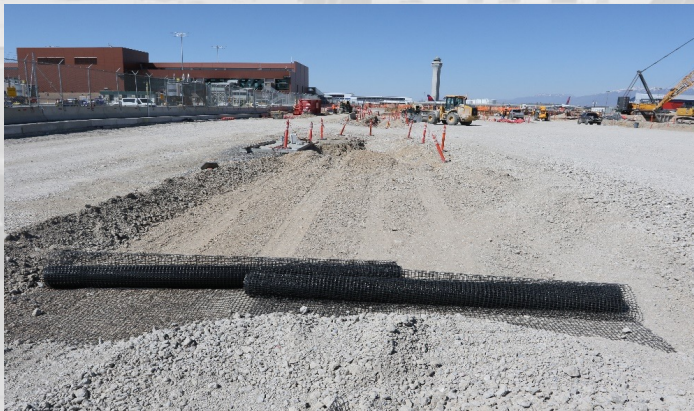
Backfill/Grading over Central Tunnel 04/2022
