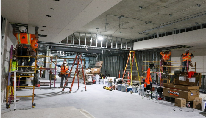
Passenger Cell Area C Framing & Drywall
