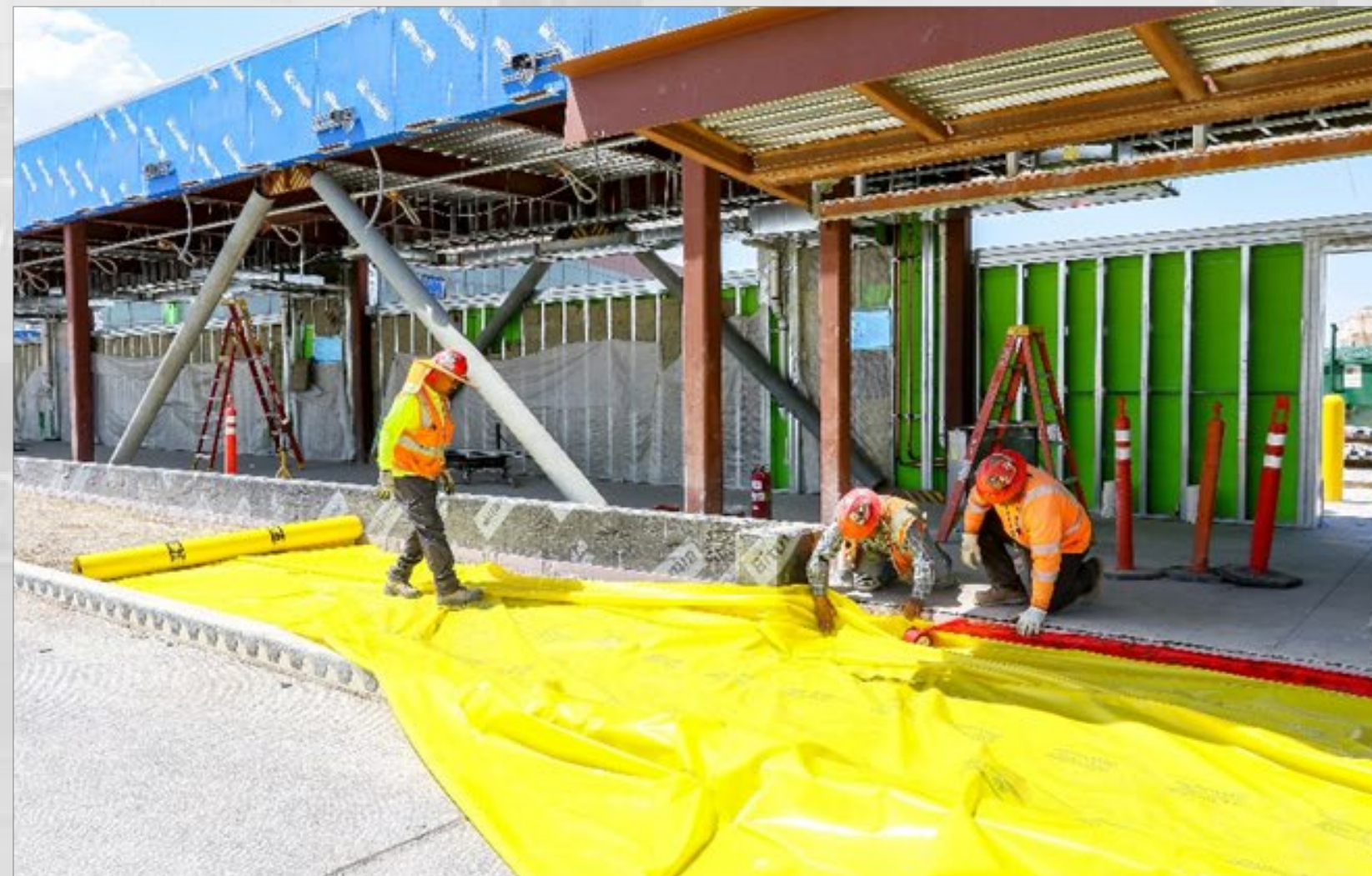
Area P Sidewalk Vapor Barrier
