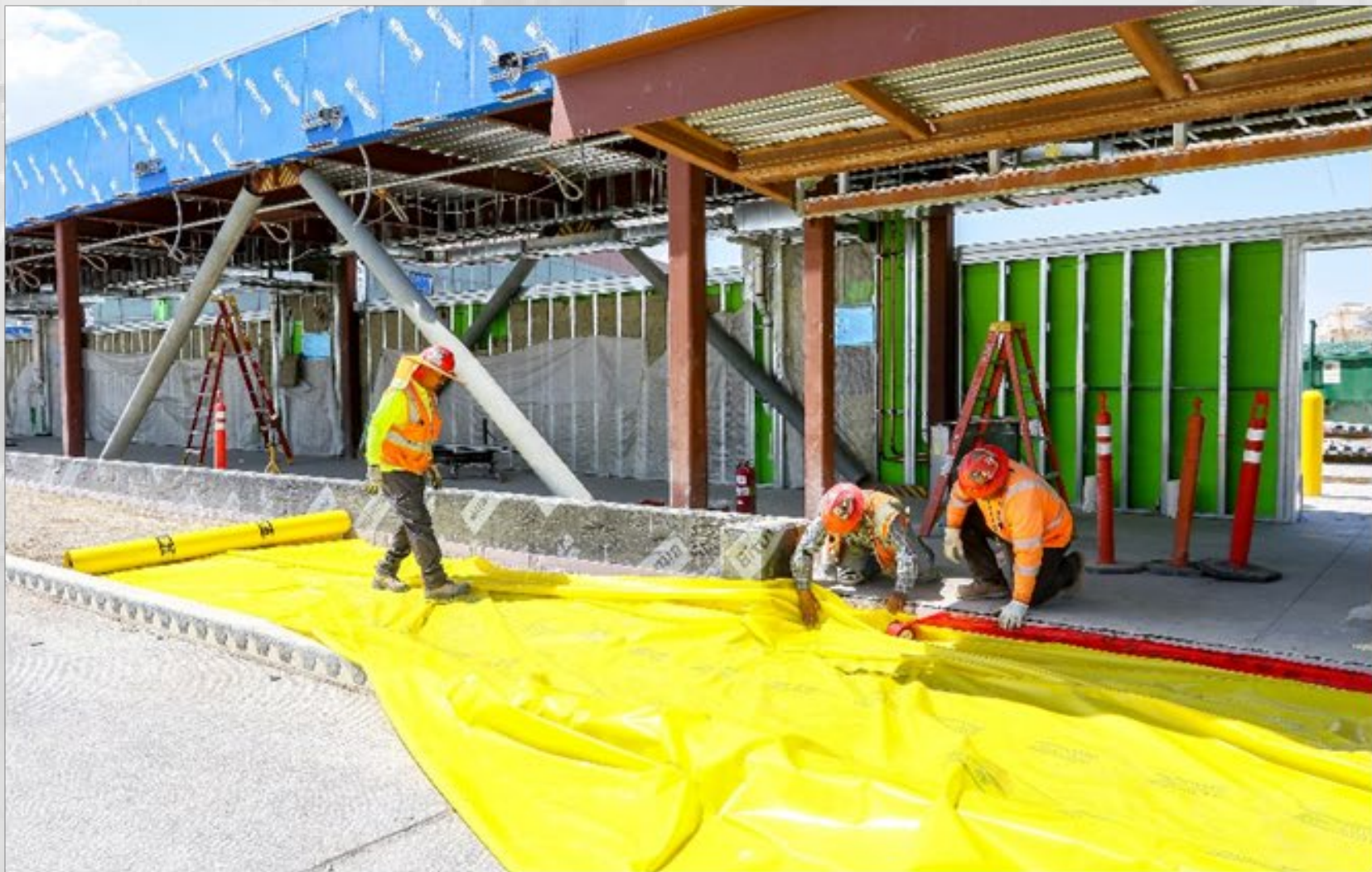
Area P Sidewalk Vapor Barrier
