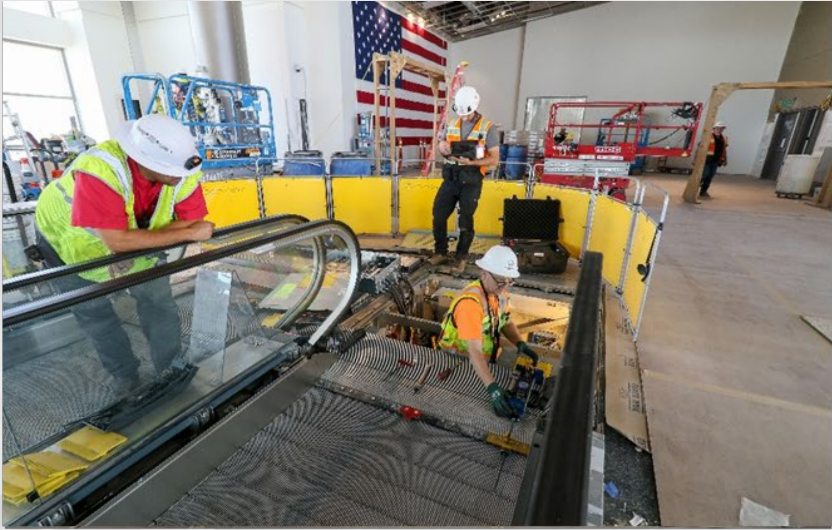
Moving Walkway Testing & Calibration
