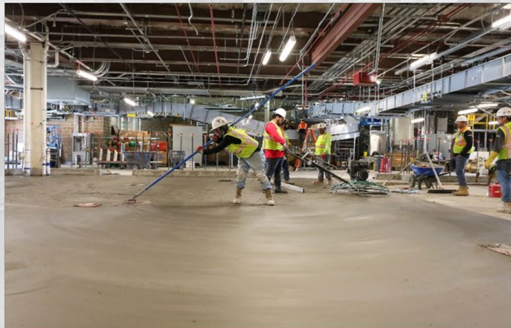
A-Nub New Slab Finishing
