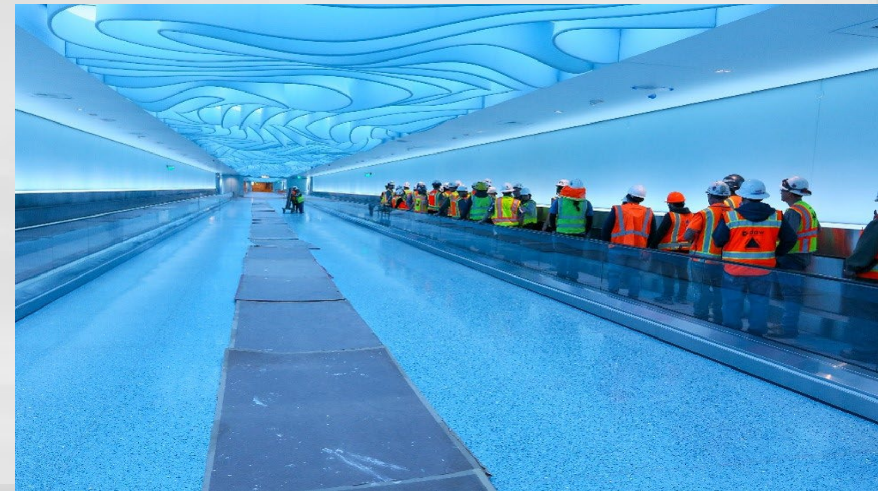
Tunnel Moving Walk Heat Load Testing
