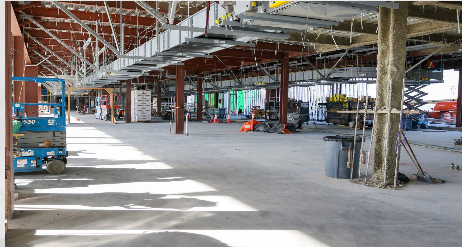
Level 1 Baggage Conveyor Installation
