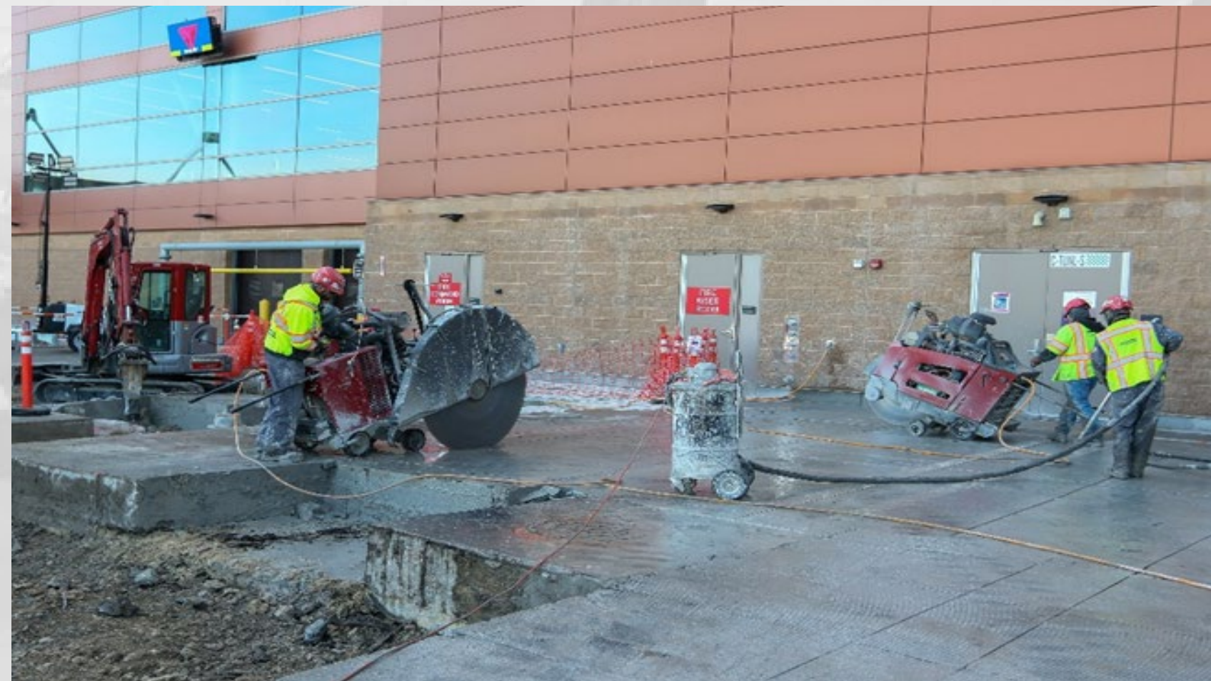
BHS Exp - Start of Building Expansion
