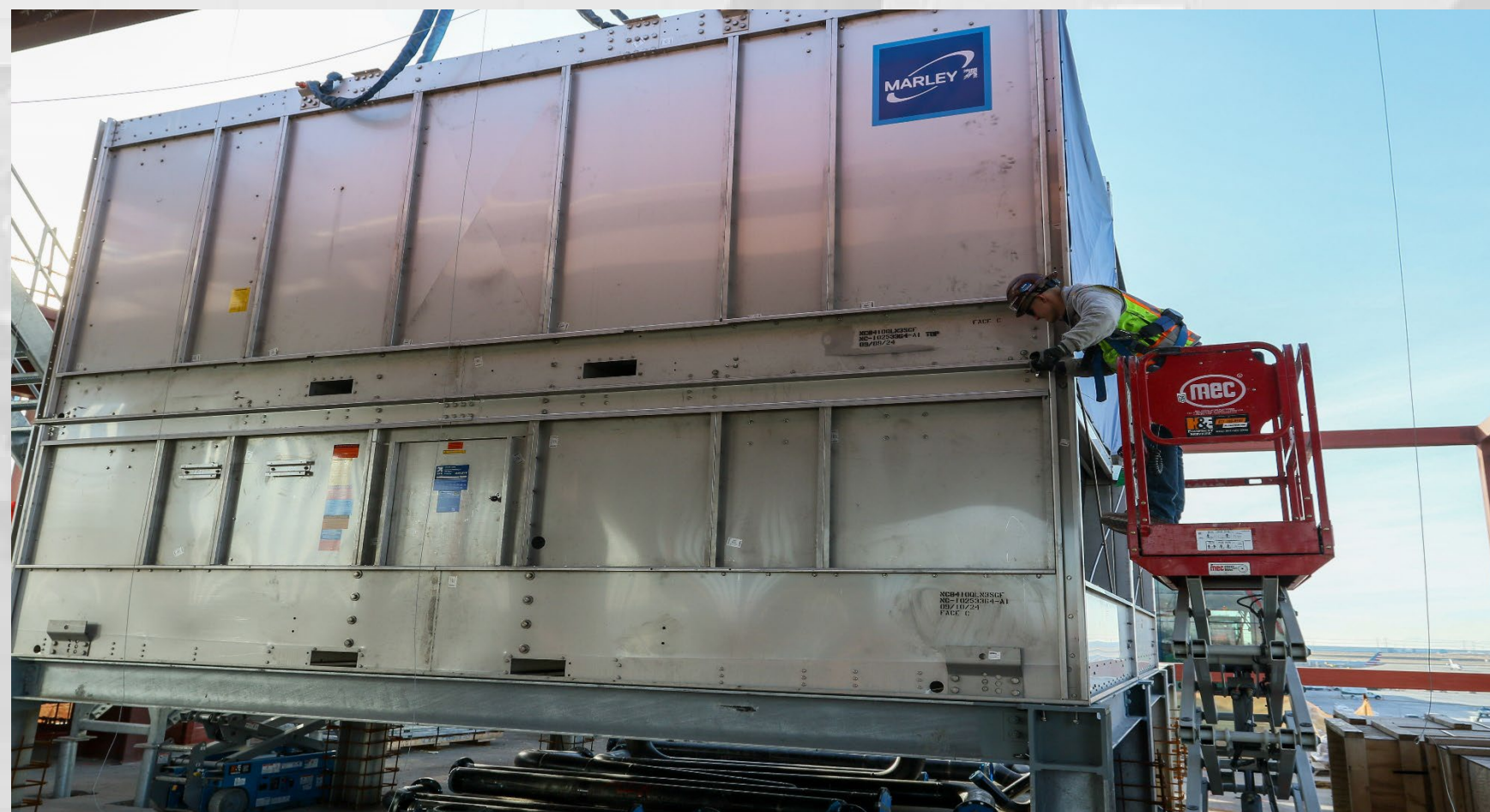
Cooling Tower Installation
