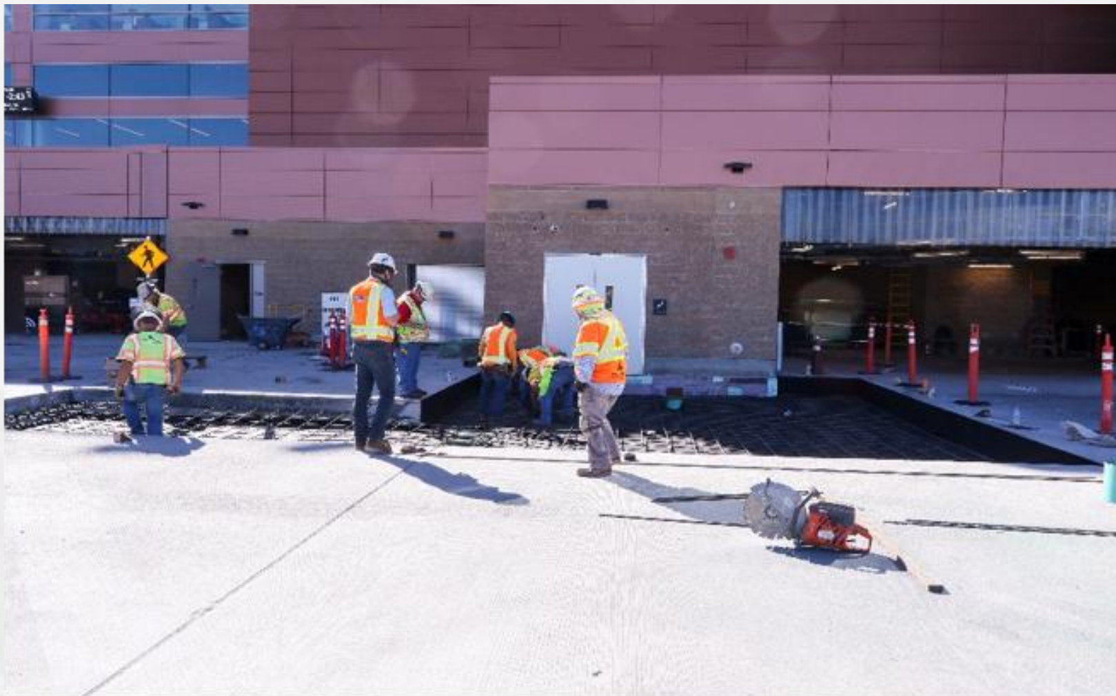
ASR Tug Lane Final Pavement Replacement
