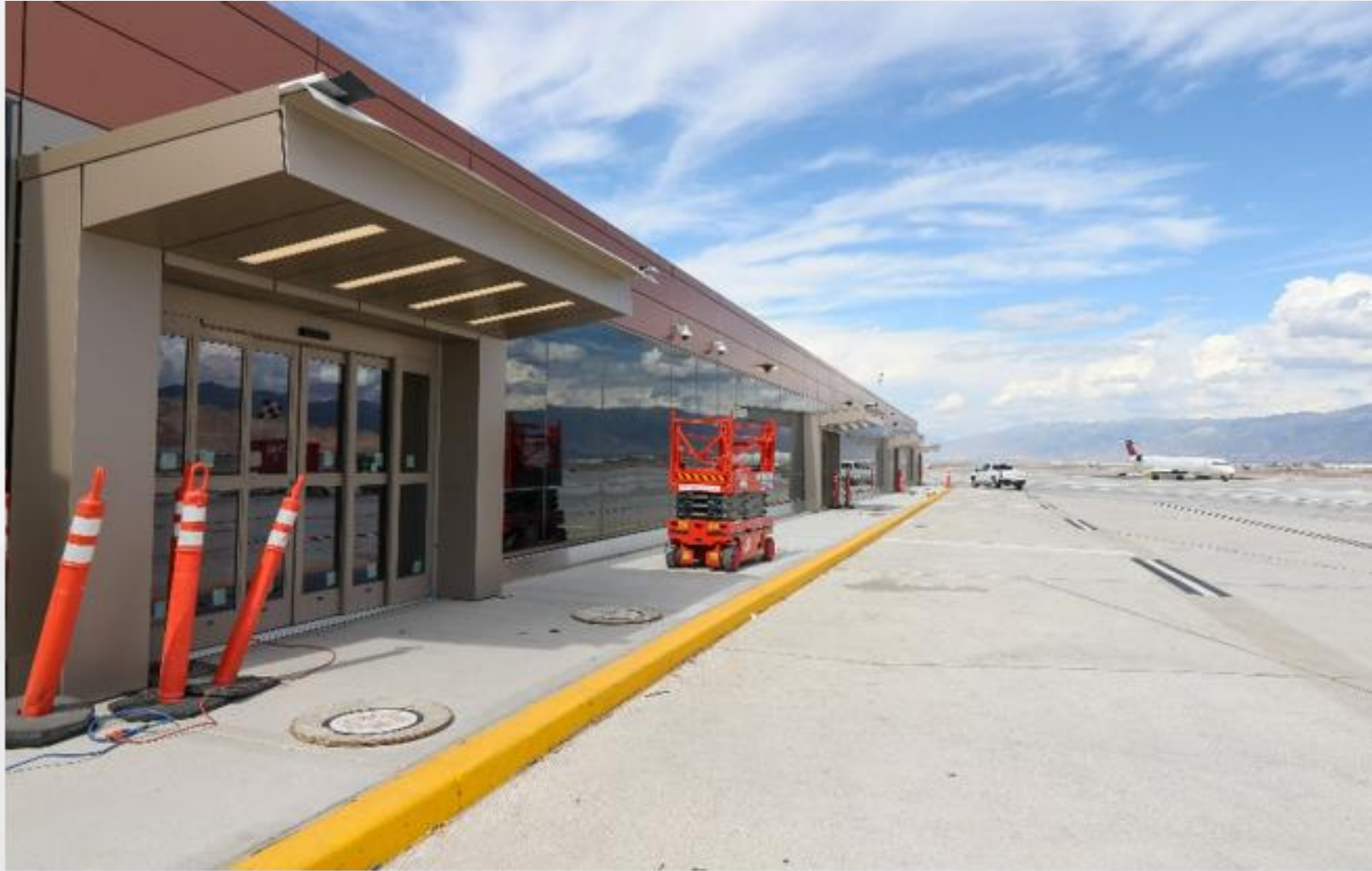
Area P Bus Shelter Looking North
