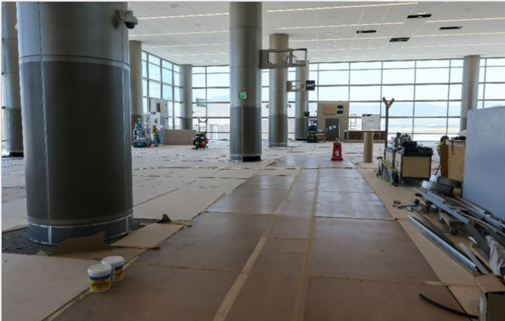
Area N Holdroom Column Covers Completed
