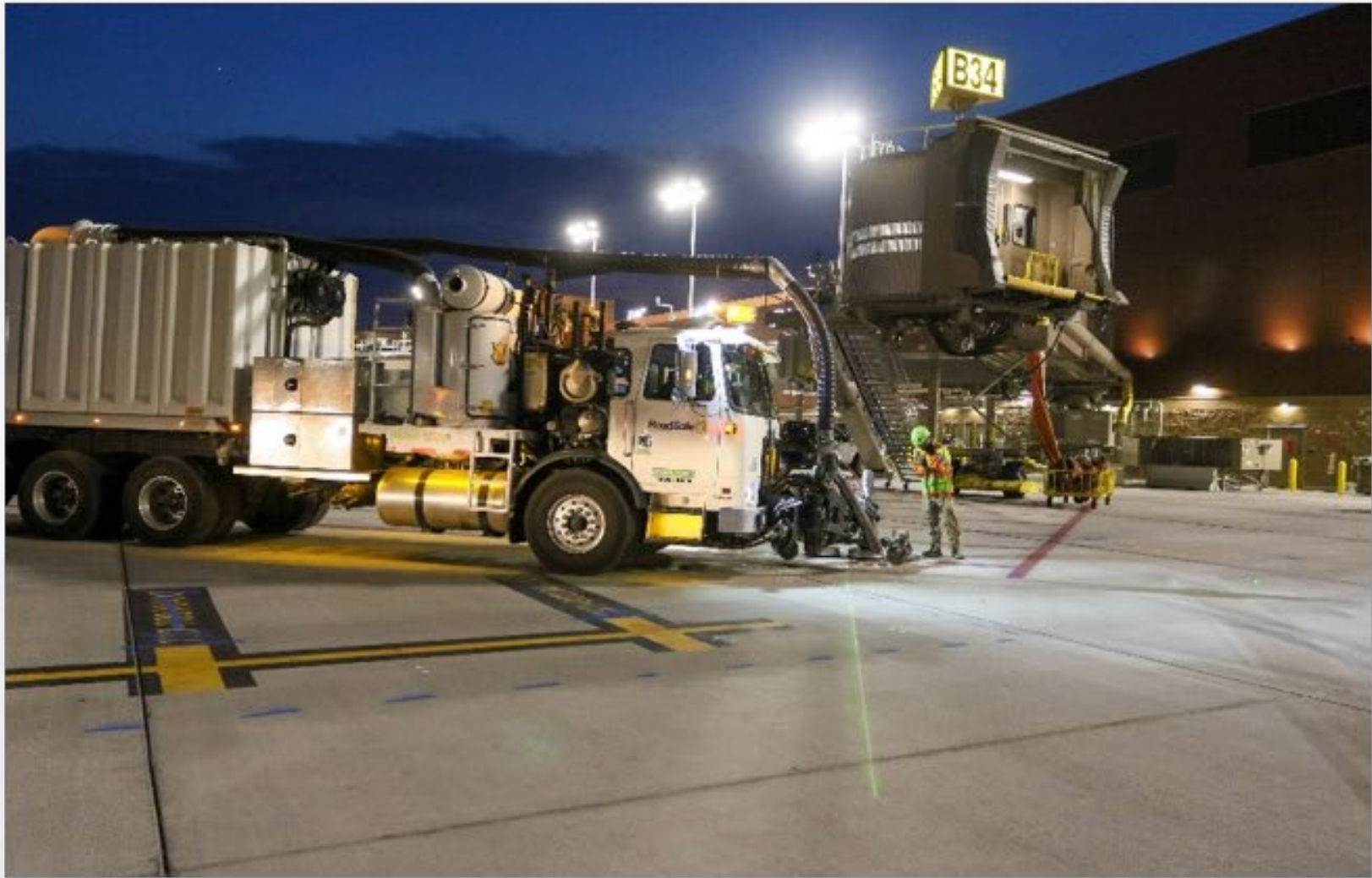
Gate B34 Apron Restriping
