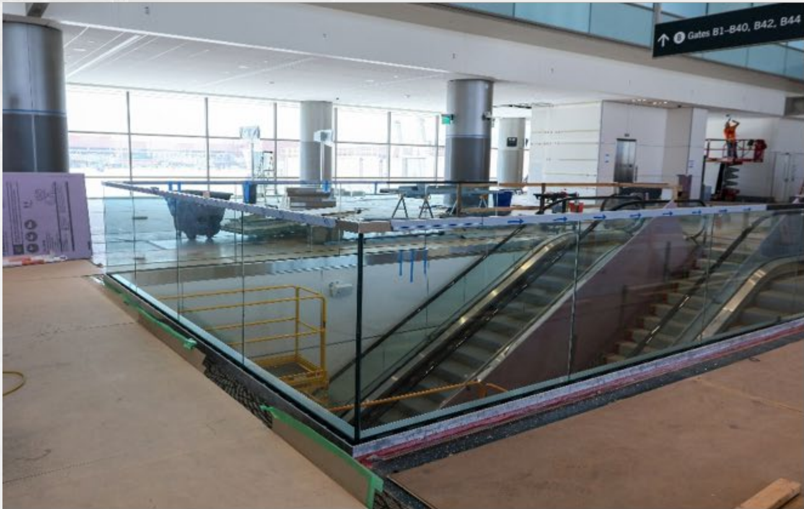
Area N Glass Handrails at Escalator
