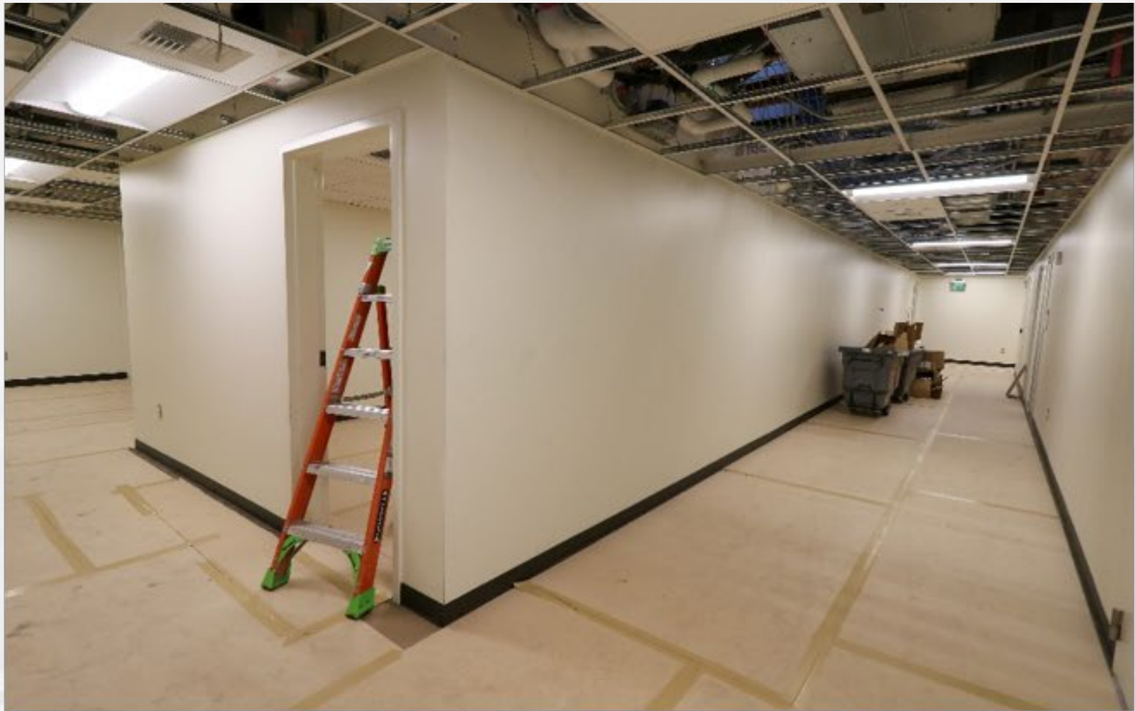
TSA Office Space Drywall & Painting
