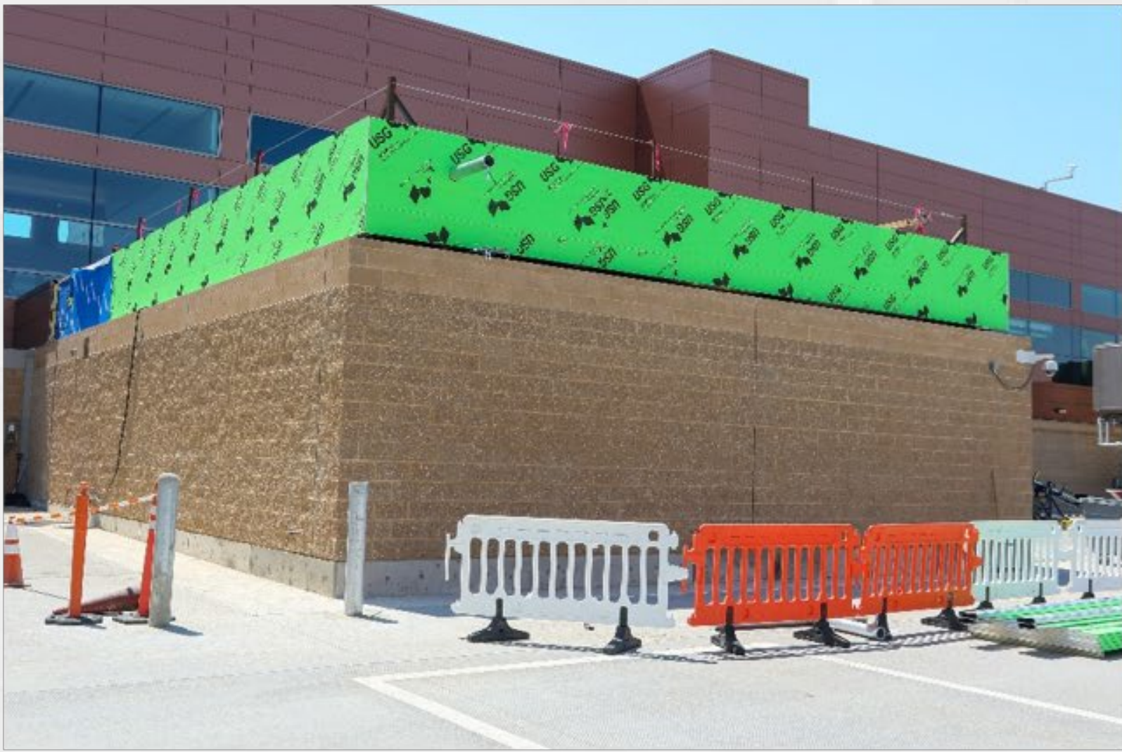
Bulletin 550 Delta Cargo Canopy Masonry & Framing
