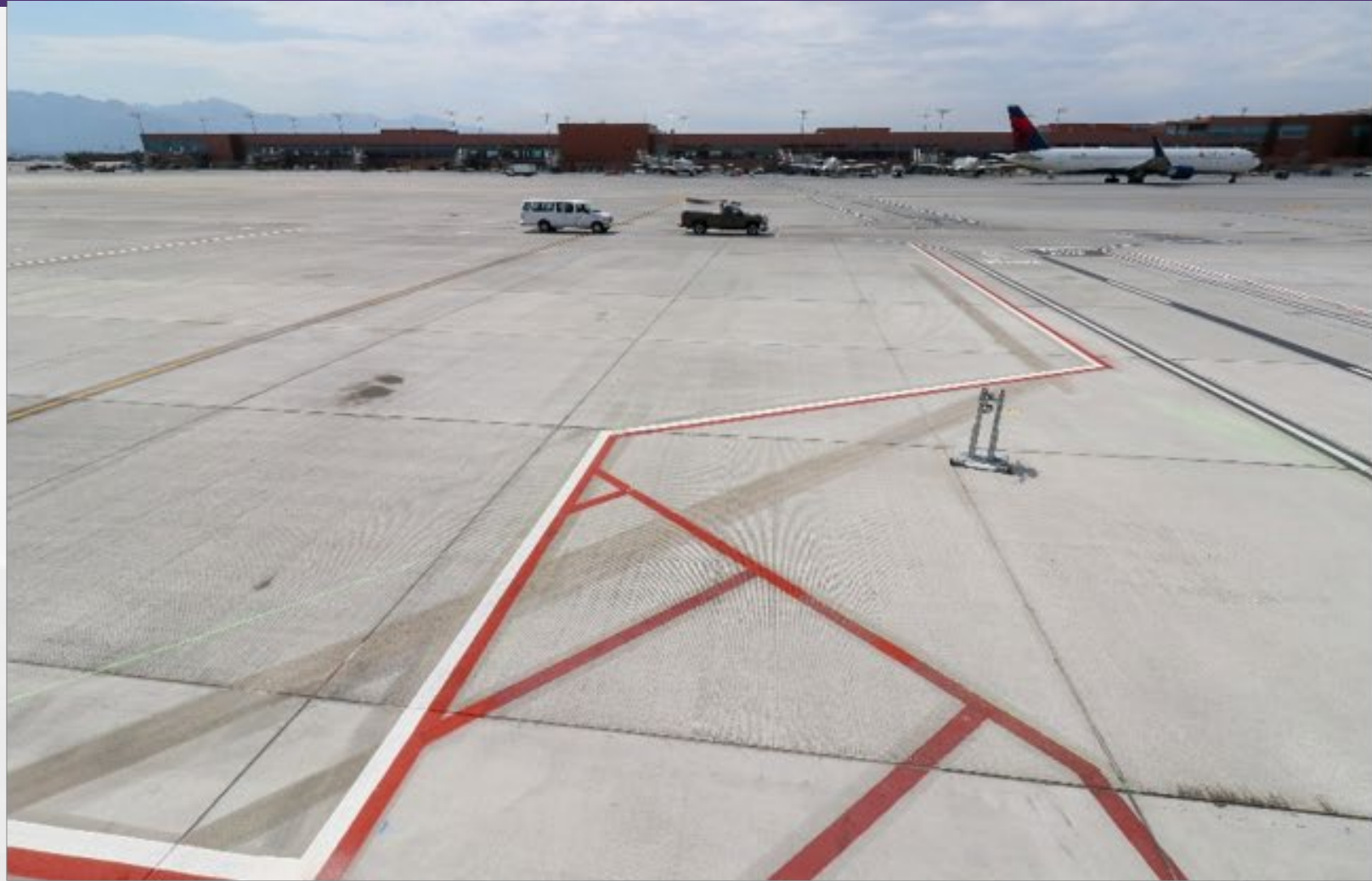
South Apron Restriped Gate B34
