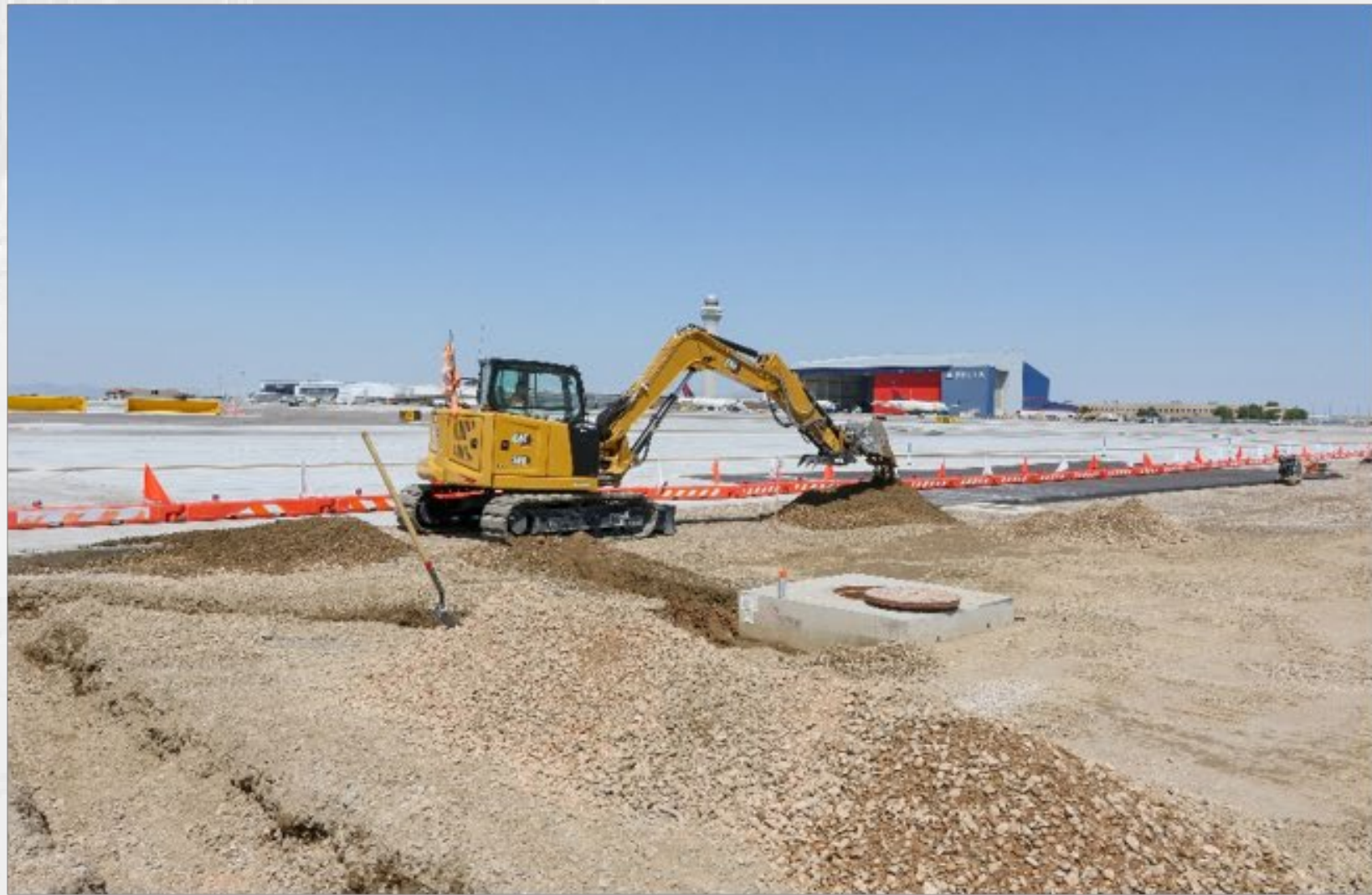
TW H Utility Ductbank Backfill
