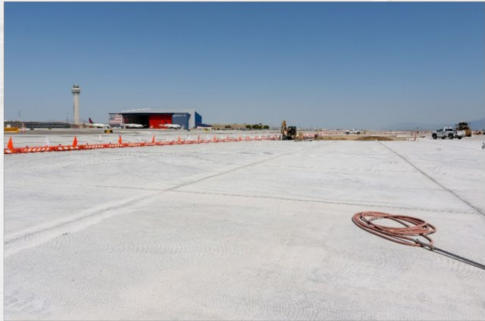
TW H P-501 Pavement Completed
