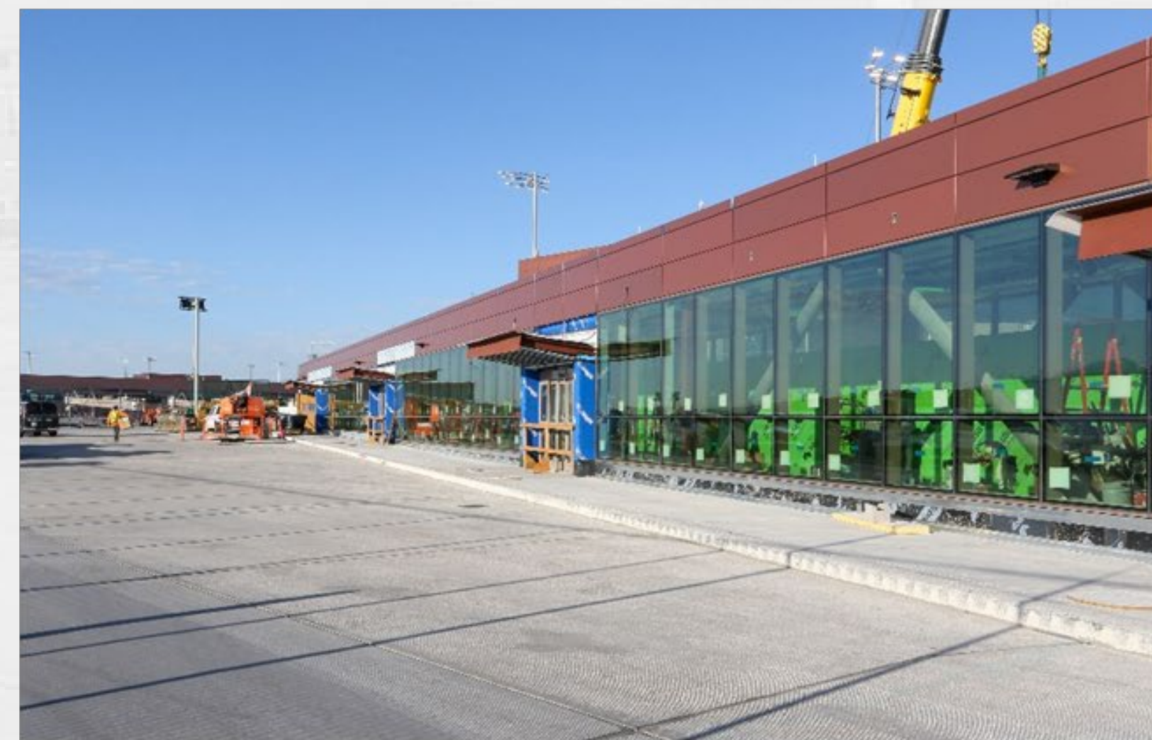
Area P Bus Shelter
