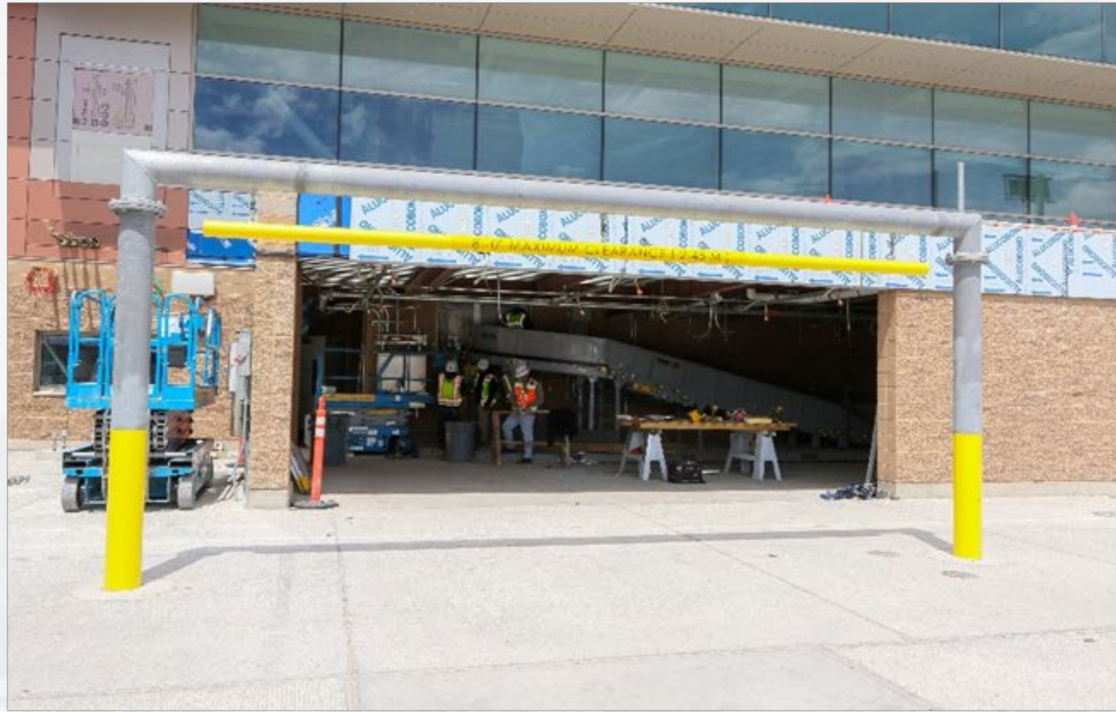
South Transfer Pier & Headache Bar
