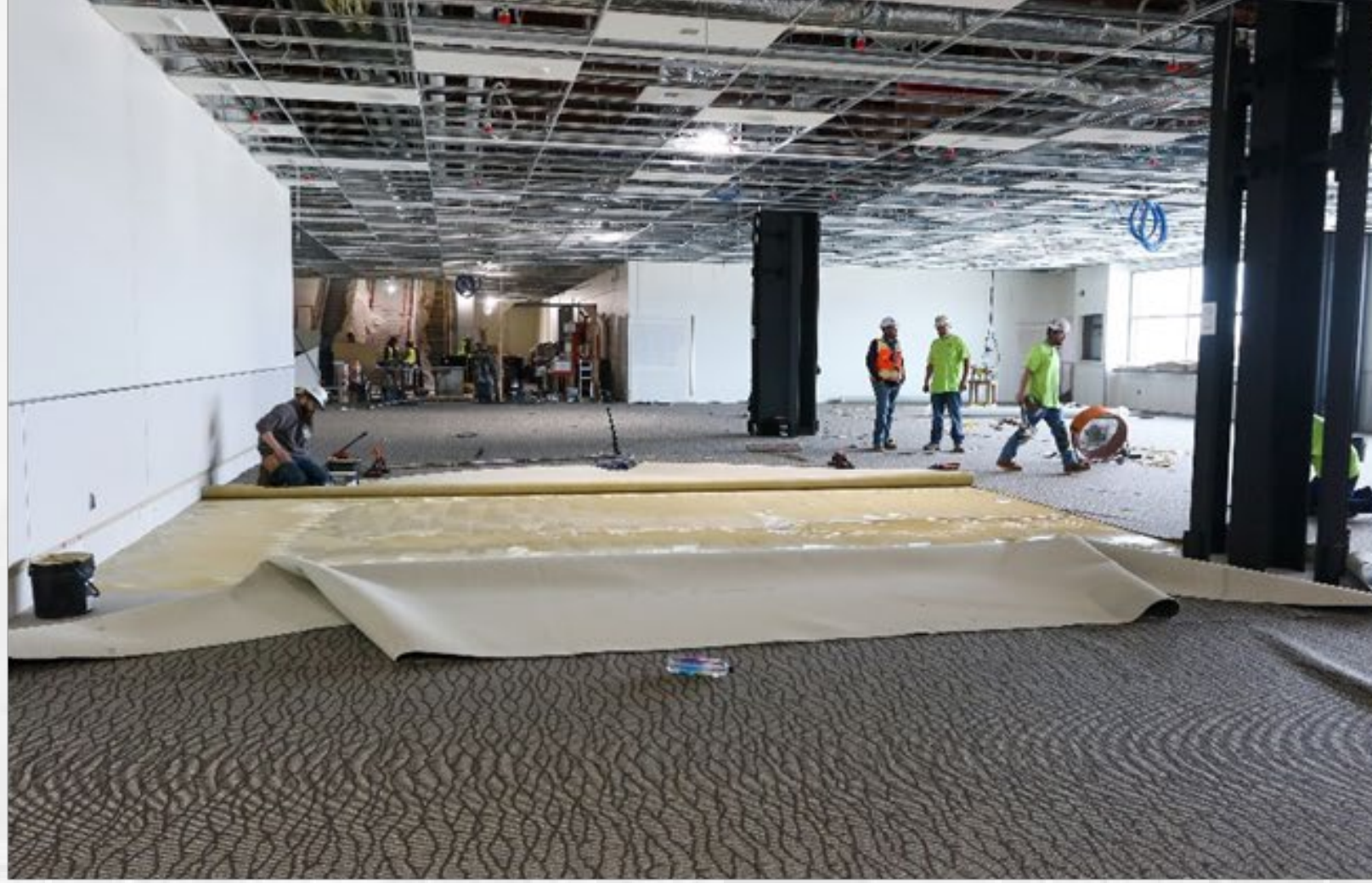
Area N Bus Shelter Holdroom Carpet
