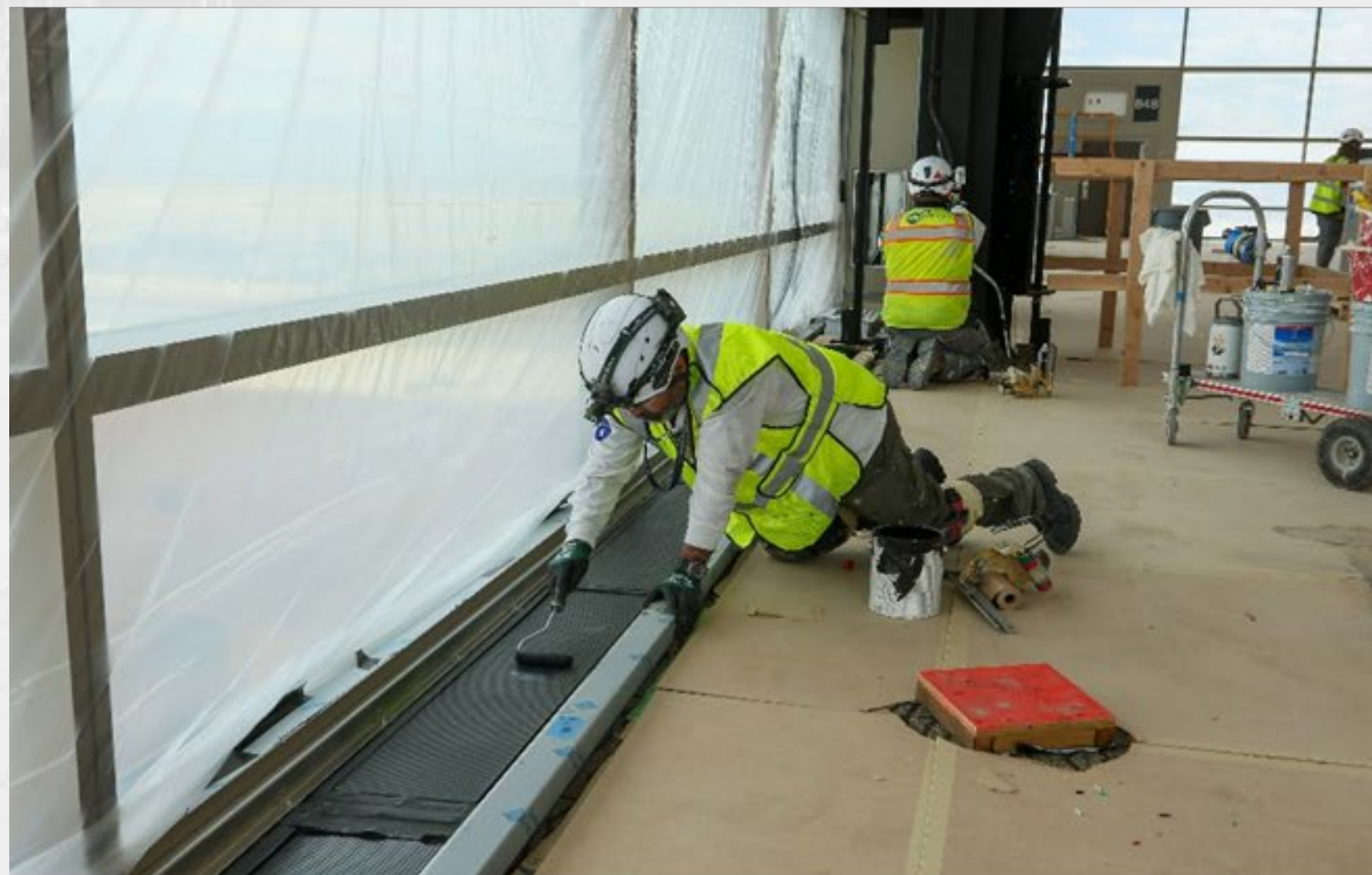
Area N Air Diffuser Painting
