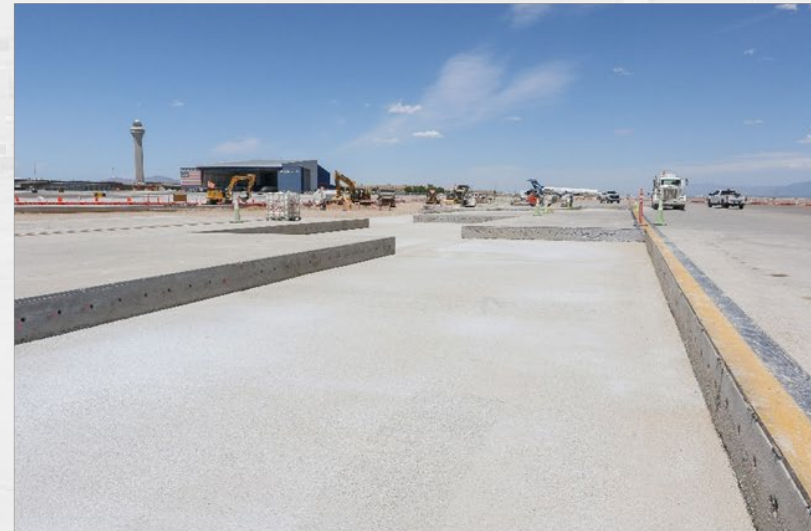
TW H P-306 Pavement
