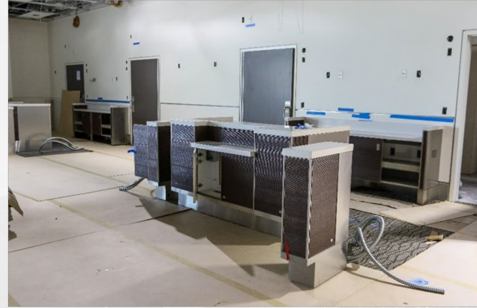
Area N Bus Shelter Holdroom Millwork
