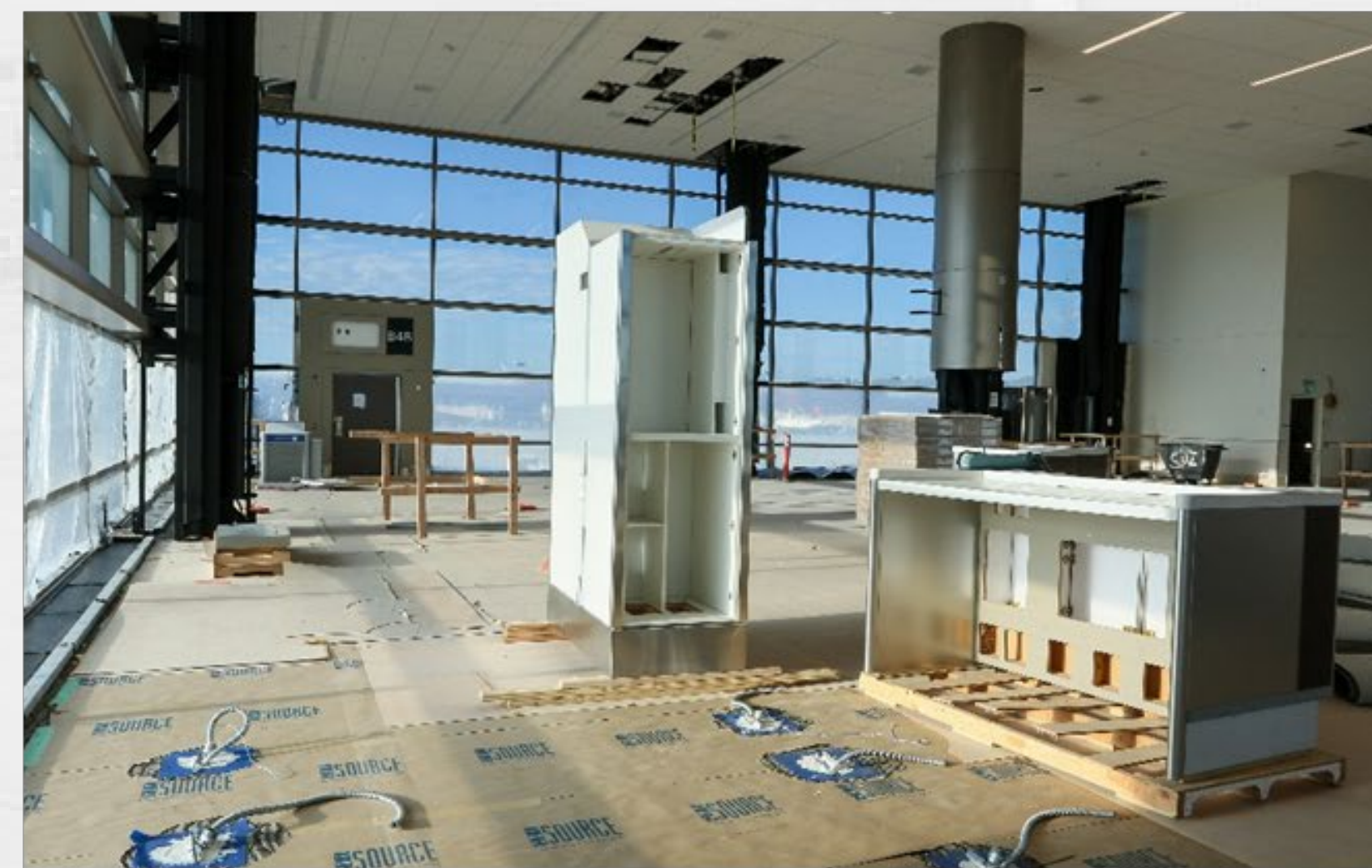
Area N Holdroom Millwork
