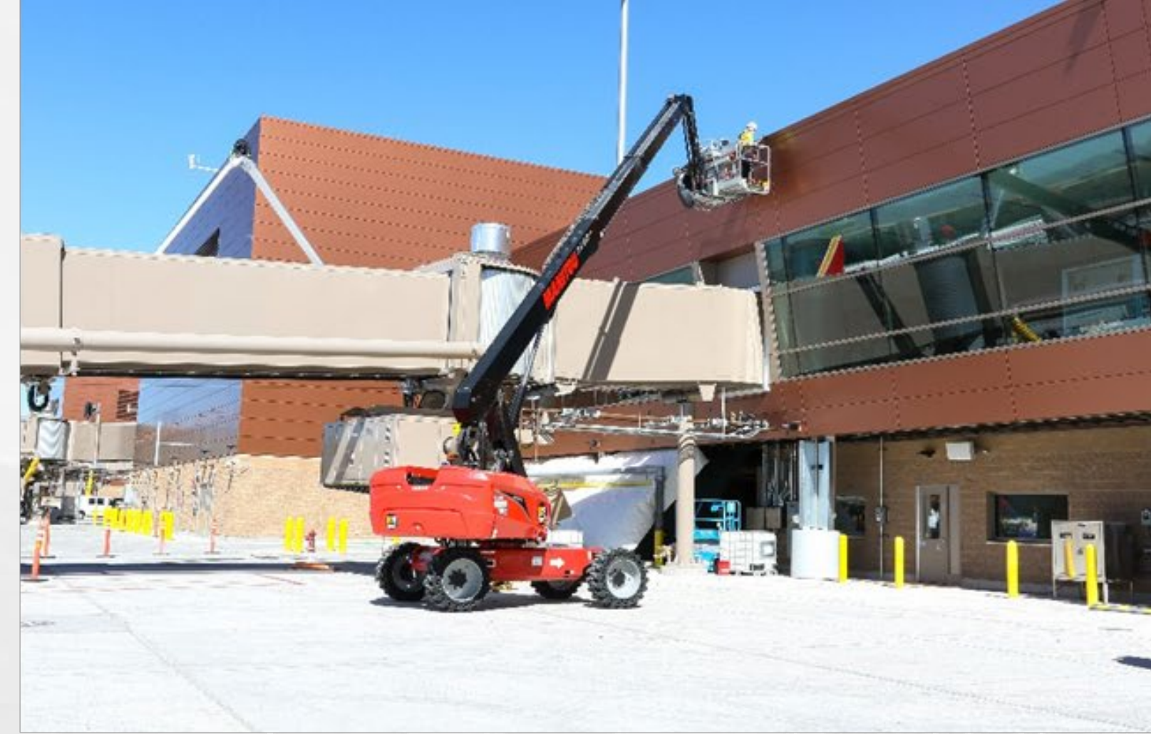
Area M Exterior Panel Punchlist
