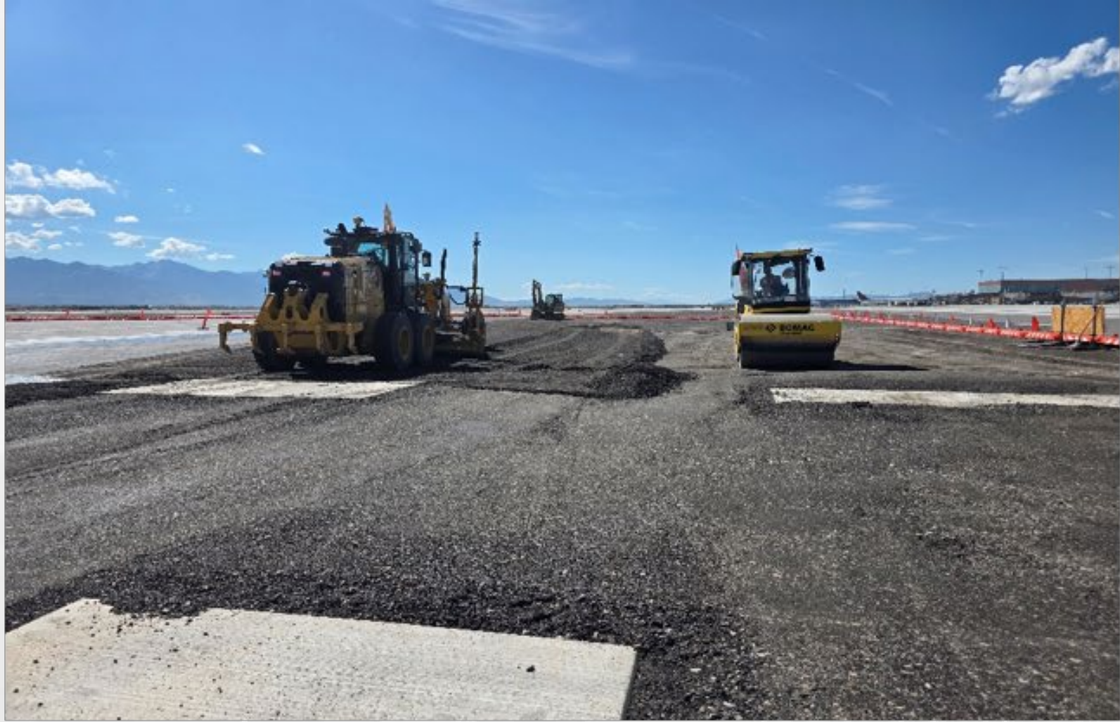
TW H Shoulder Millings Placement
