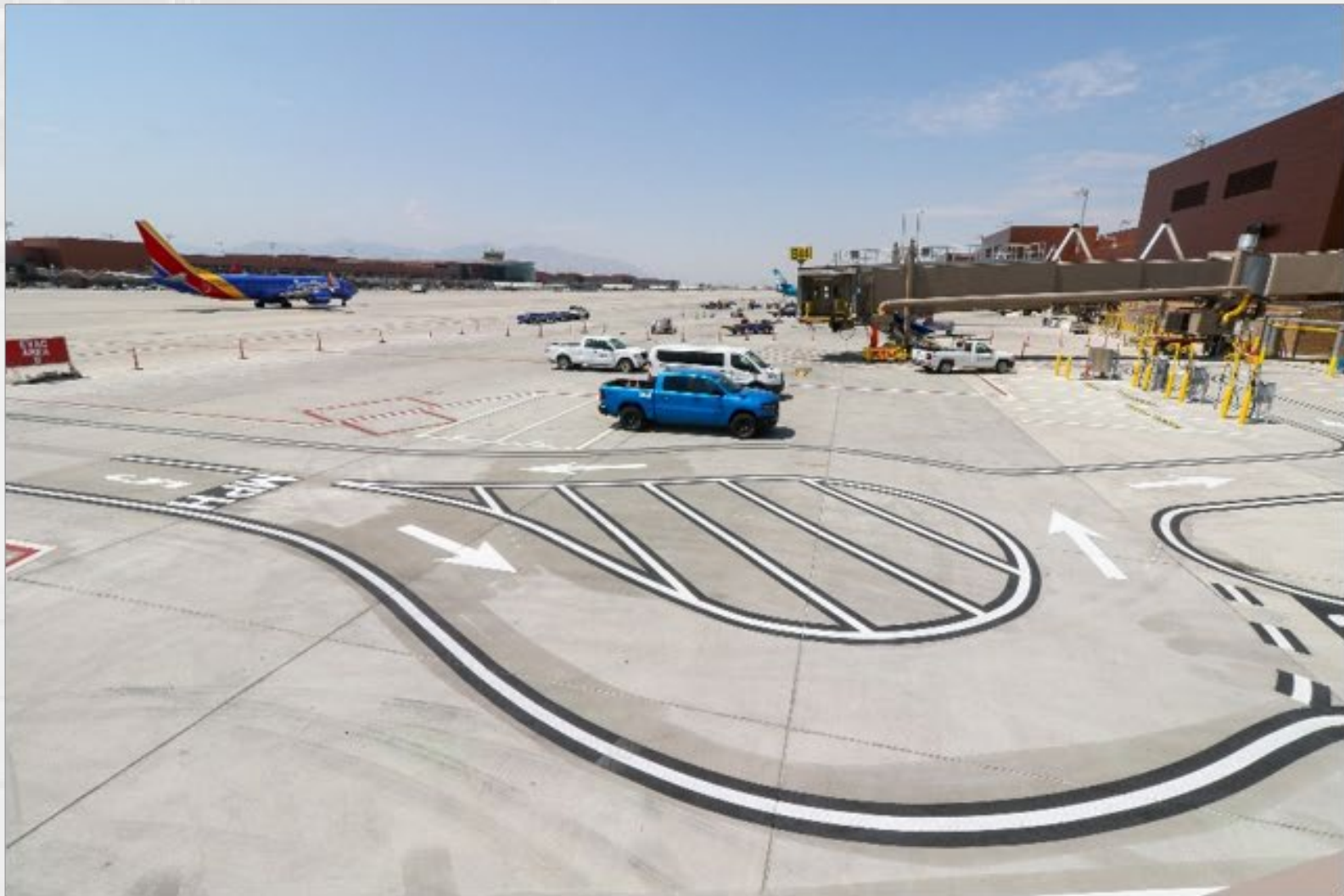
Area M South Apron Striping
