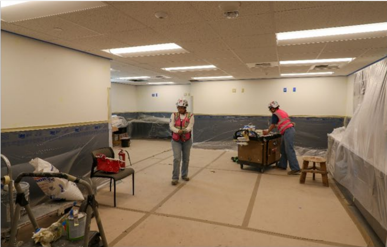
Area M Airline Ops Final Paint
