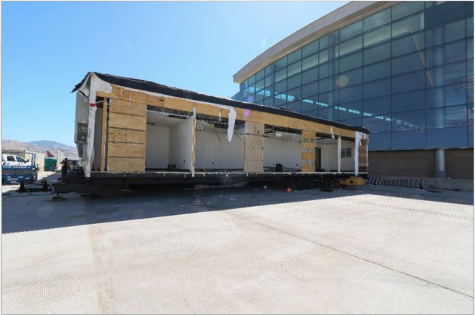
BHS Expansion TSA Temporary Trailer Demobilization
