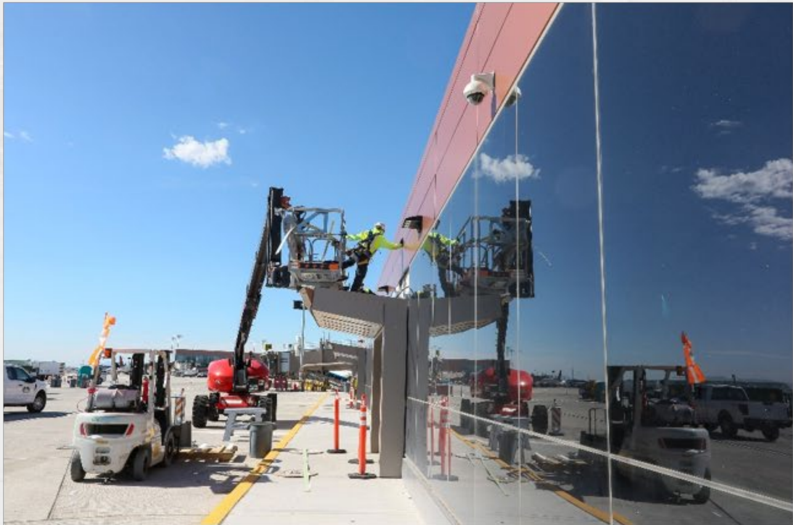
Area P Bus Shelter Canopy Roofing
