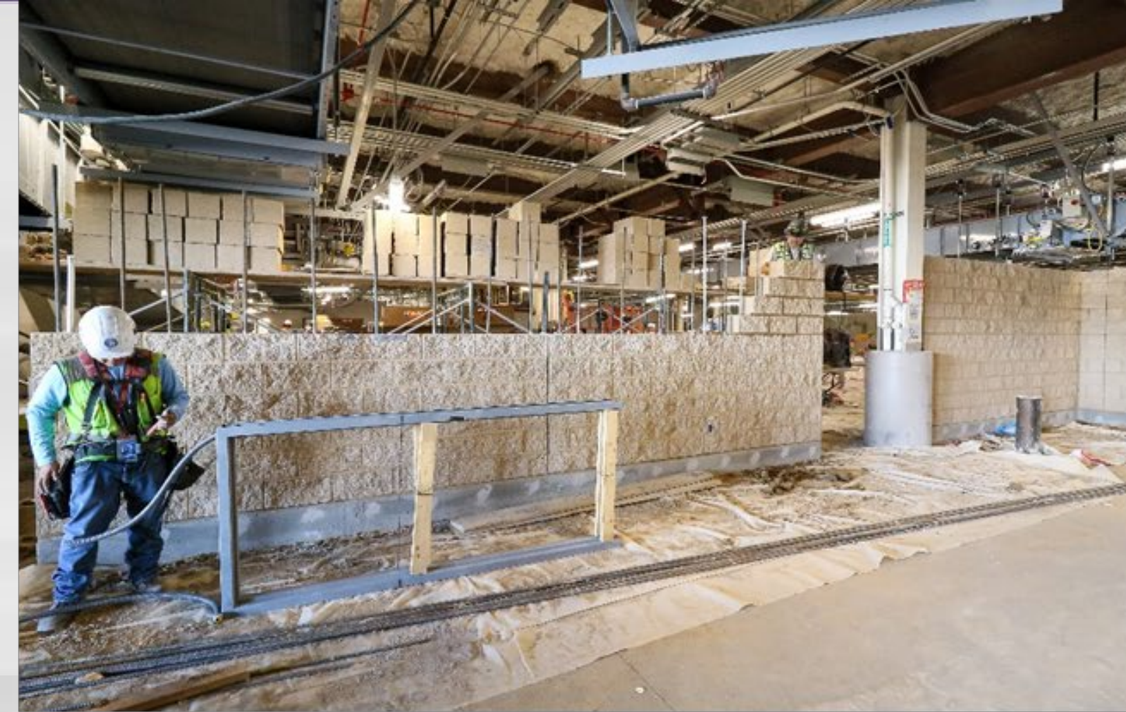
Interior Masonry for CBIS
