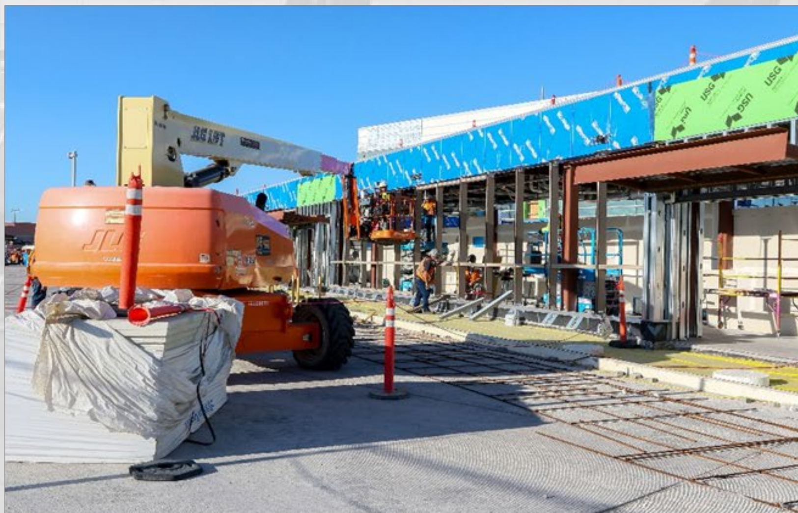
Area P Bus Shelter Glazing Framing – East Face
