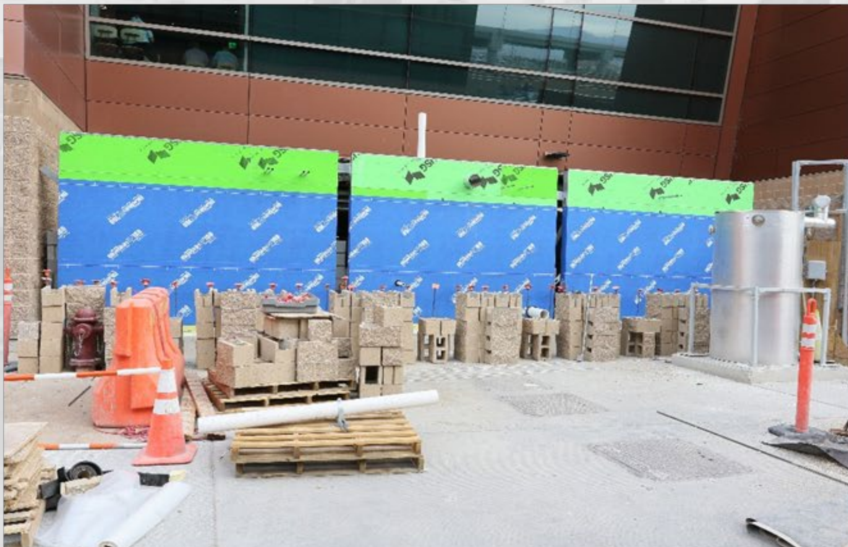
A-Nub Building Expansion Exterior Sheathing
