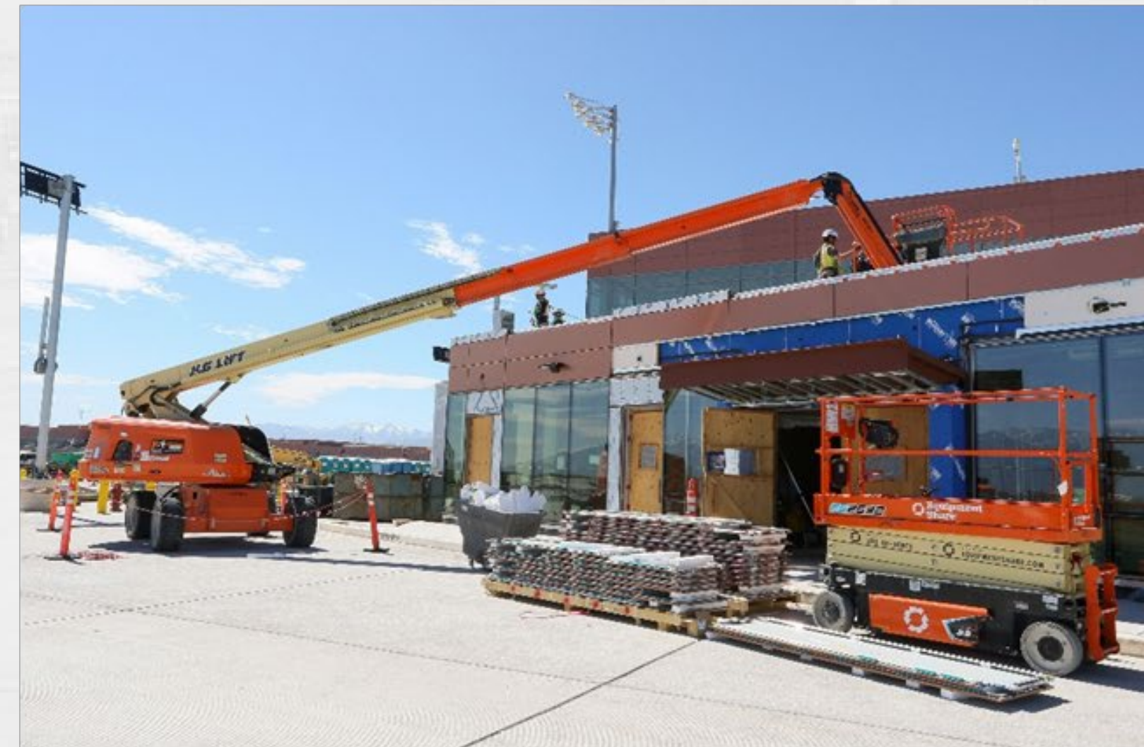
Area P Bus Shelter Roof Parapet Trim
