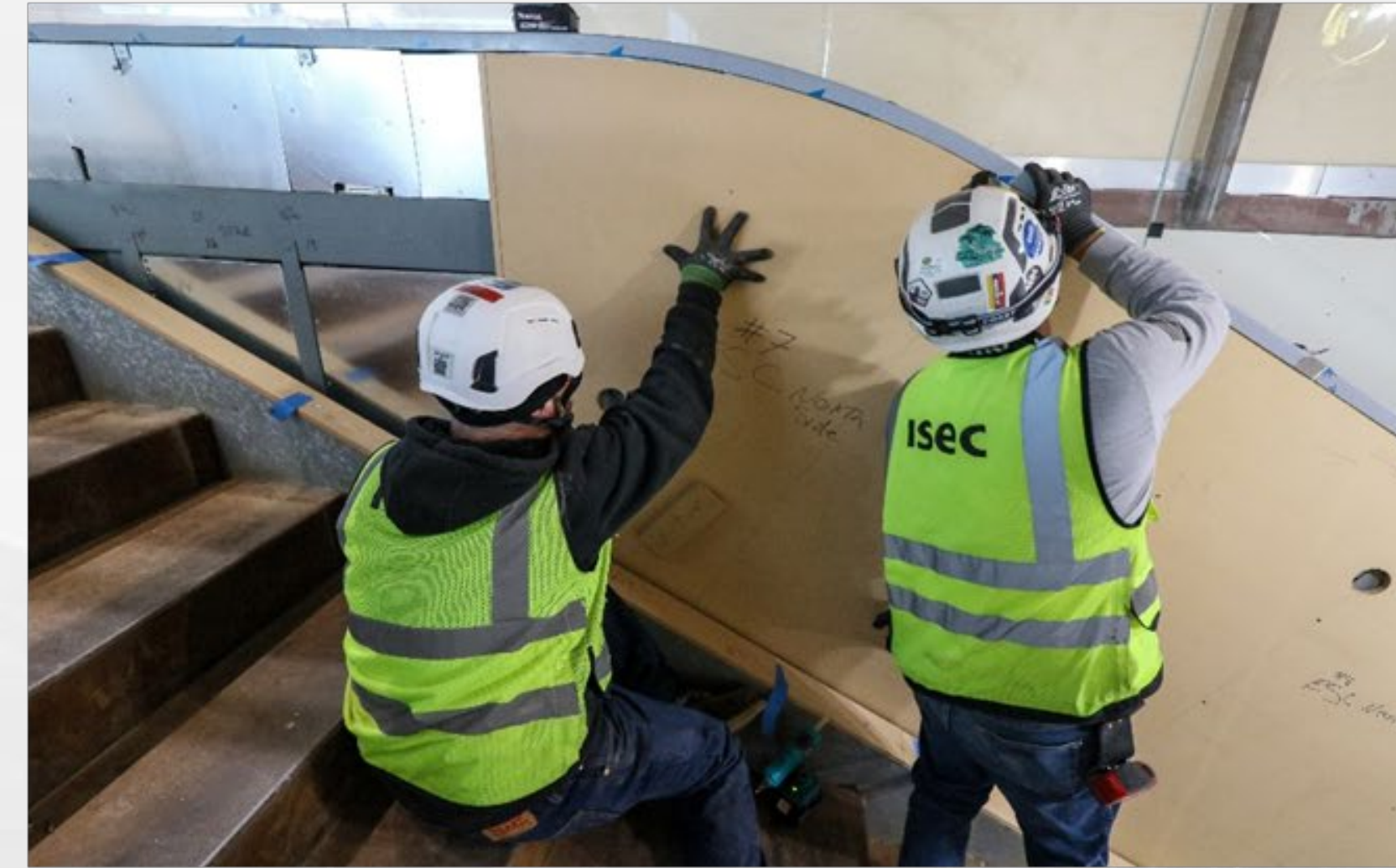
Area N Escalator Trim Underlayment
