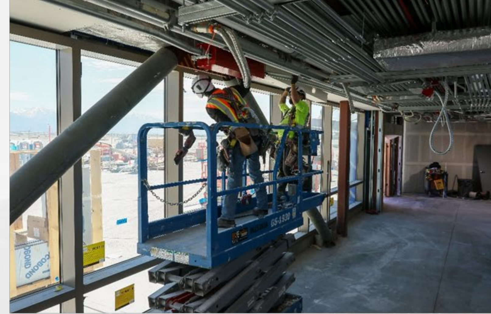
Area P Bus Shelter Soffit Drywall
