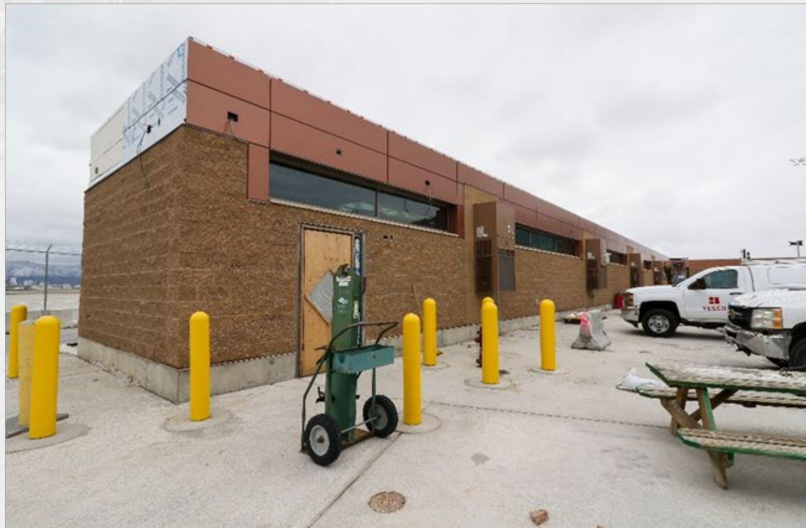
Area P Bus Shelter Metal Panels & BARD Units
