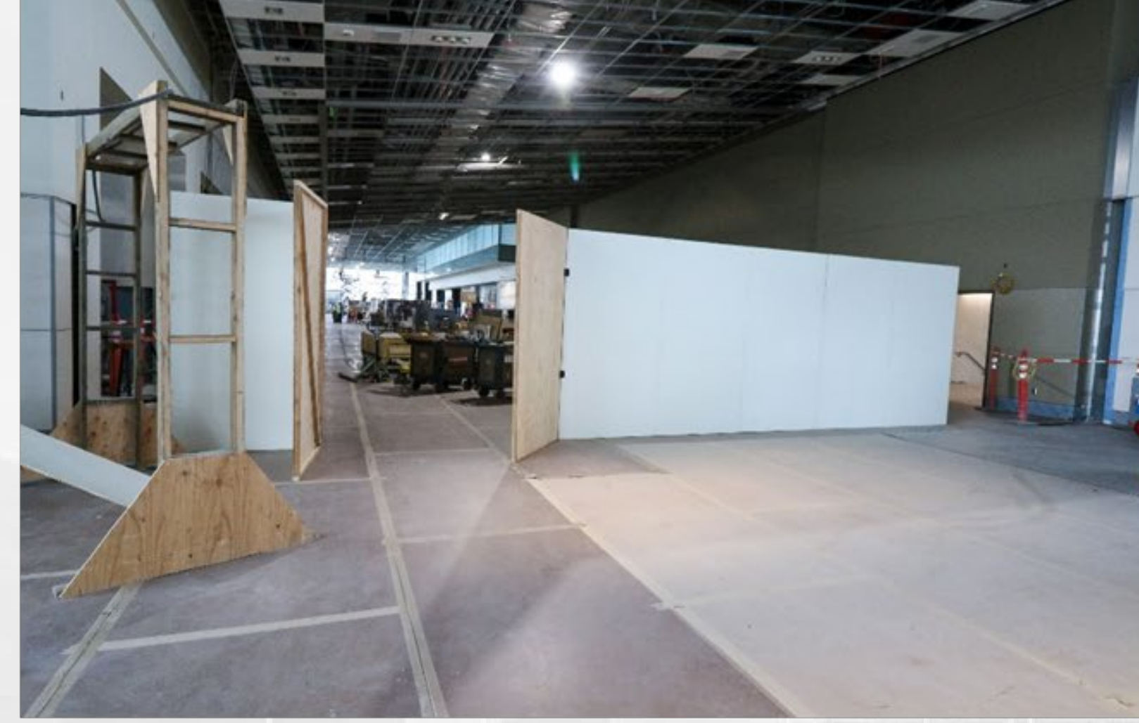
Area M New Separation Wall
