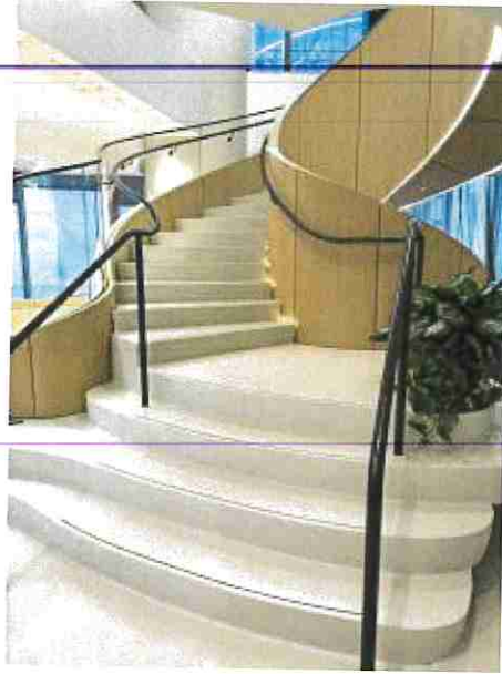
A CIRCULAR TERRAZZO staircase rises from a hand-poured, asymmetrical terraced platform in this installation by Zonca Terrazzo of Armonk, New York, at Clifford Chance in New York City. Courtesy of Zonca Terrazzo/Matt Holdsworth
