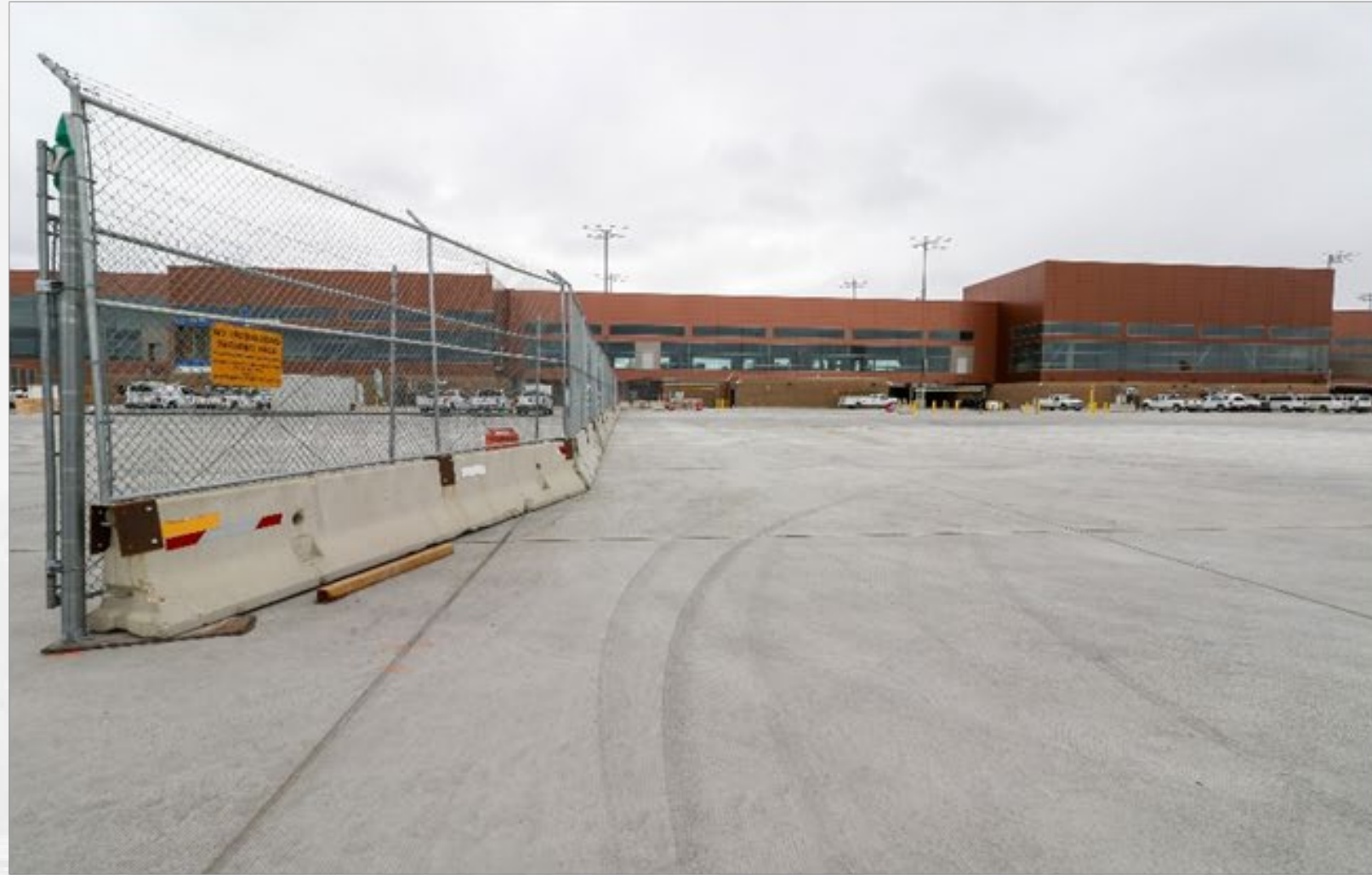
North Apron Fence Relocation
