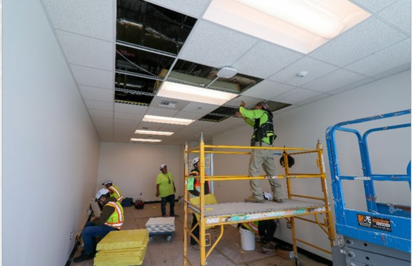
Bulletin 540 Concourse B Delta Above Wing Offices
