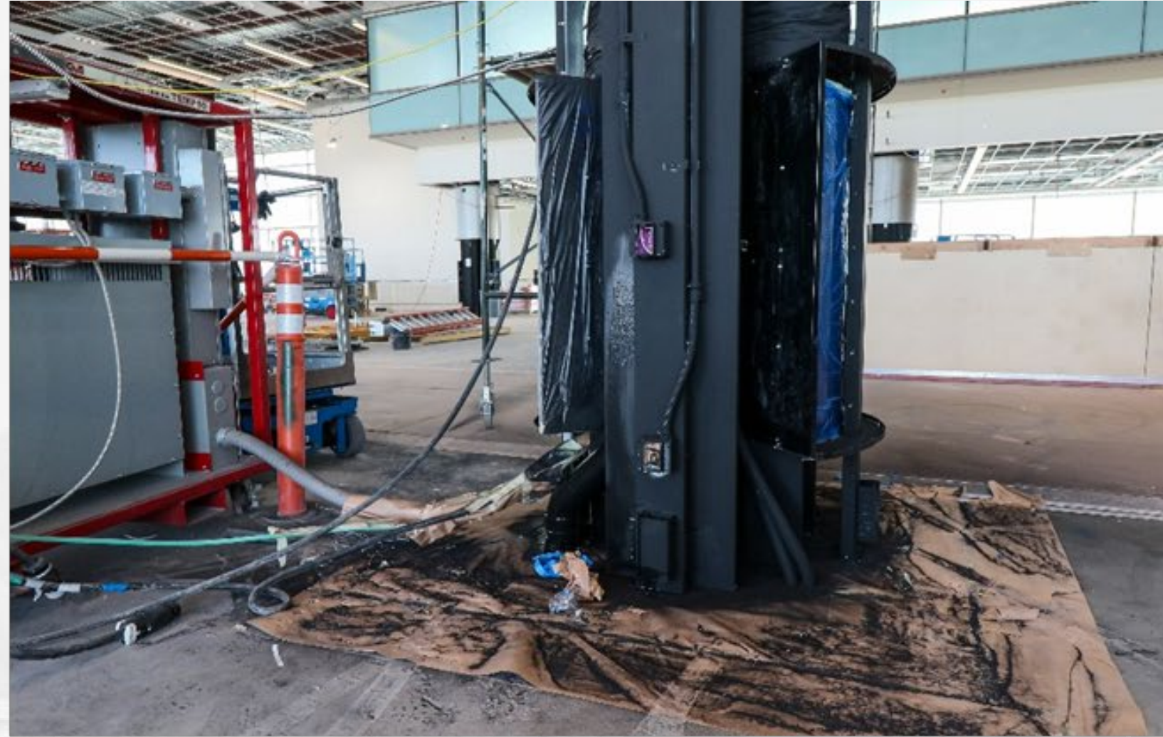
Area M Column Interior Devices & Painting
