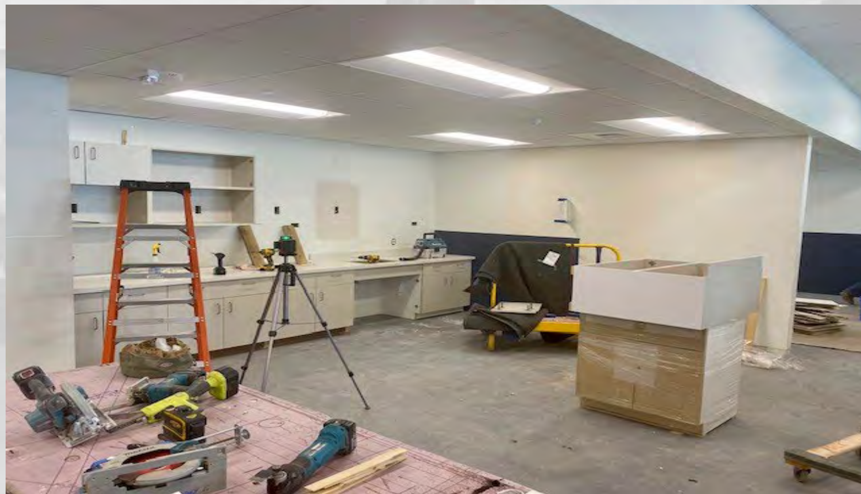
Setting Breakroom Millwork
