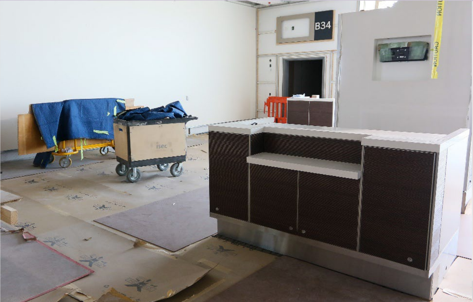
Gate B34 Millwork Installation
