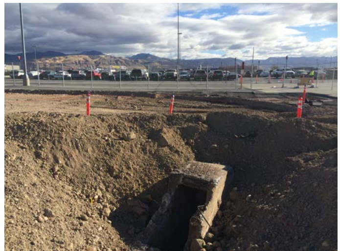
Break into box at 60" drainage line Monday, November 10 th , 2014 9:51 am
