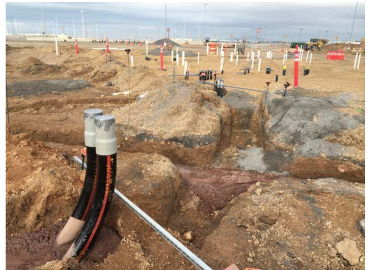
Electrical feeder lines for RSS A Wednesday, January 28 th , 2015 9:42 am
