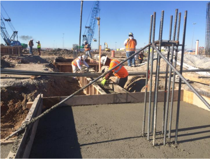
Placing concrete for footings and tie-beams Thursday, January 22 nd , 2015 12:04 pm
