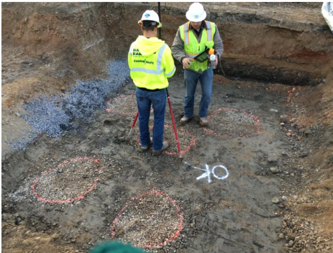
Accepting the stone columns and soil conditions in a spot footing Wednesday, December 17 th , 2014 8:52 am
