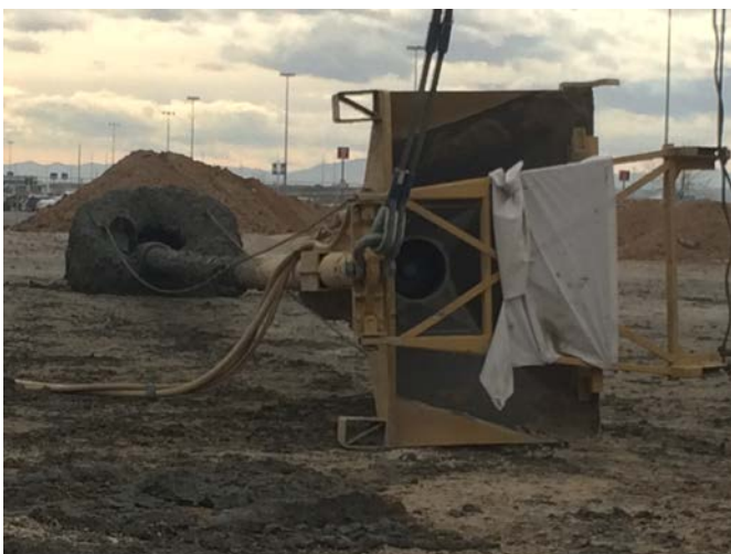
Hopper, vibrator column and tire Friday, November 14 th , 2014 11:27 am
