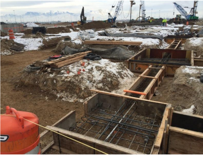
Formwork for footings at the east edge of the QTA Monday, January 5 th , 2015 11:29 am
