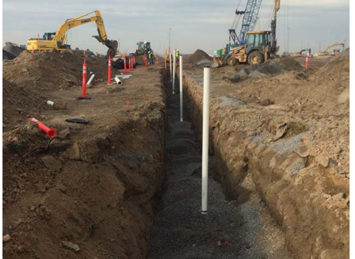
Storm drain line for trench drains at southmost bay of QTA Tuesday, January 27 th , 2015 9:37 am
