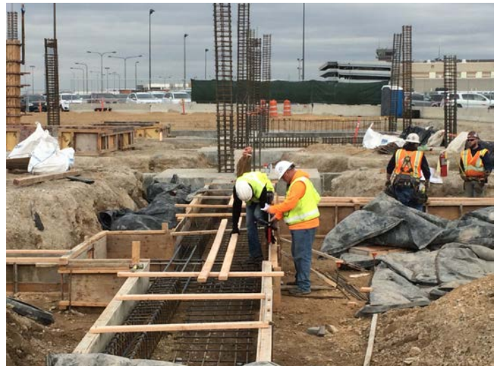
Formwork for base of east QTA ramp Wednesday, January 28 th , 2015 9:59 am
