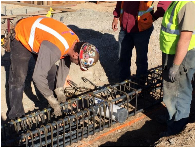
Sleeves for trench drains through grade beams Wednesday, December 10 th , 2014 1:52 pm
