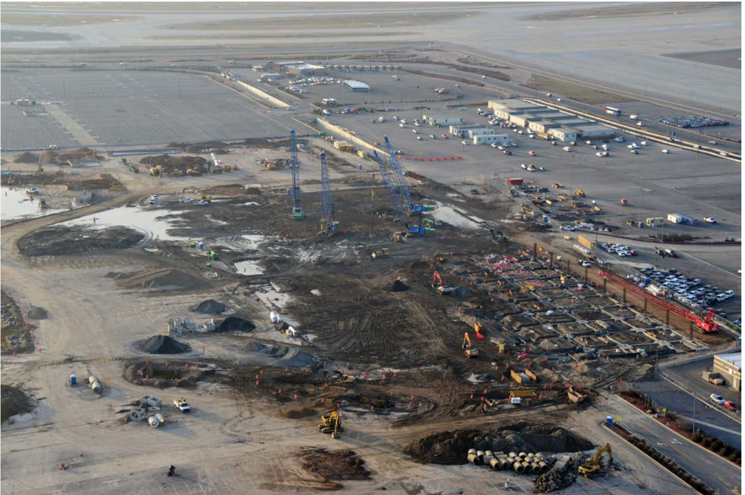
QTA overall site – Stone column cranes on the west half, footings and tie-beams starting from northeast corner Thursday, January 15 th , 2015
