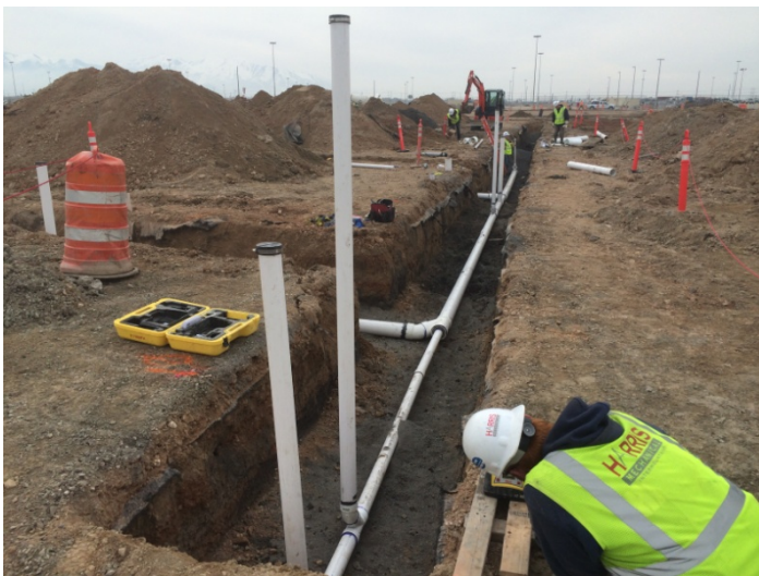
Storm drain and trench drain lines at northwest quadrant of QTA Thursday, January 29 th , 2015 3:36 pm
