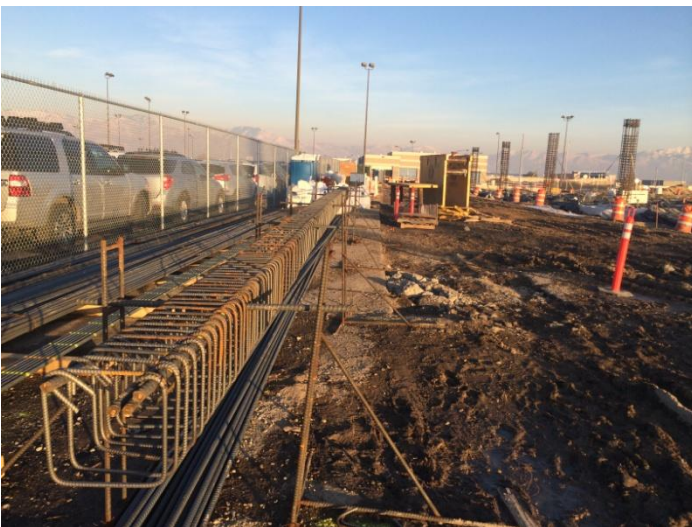
Staging area for tying re-bar for tie-beams Tuesday, January 6 th , 2015 4:36 pm
