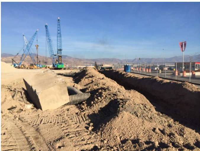
Removal of storm drain and catch basin – SW corner Friday, November 5 th , 2014 3:42 pm
