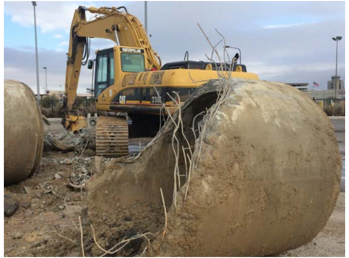
Old storm removed 60" storm drain line remnants Tuesday, January 13 th , 2015 11:46 am
