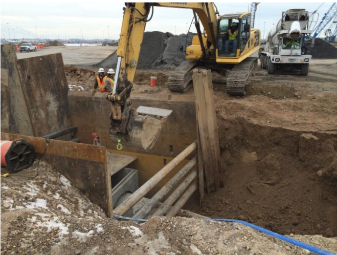
Placing concrete for collar at the box Monday, January 5 th , 2015 11:43 am
