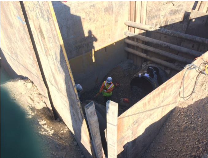
60" storm drain tie-in being prepared for new box Monday, December 15 th , 2014 10:26 am
