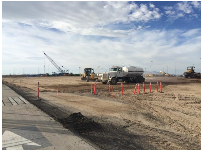
Center of QTA site graded and compacted – view from southeast corner - Friday, October 31 st , 3:45 pm
