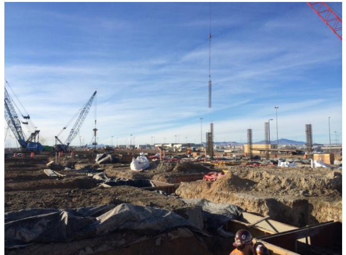
Column rebar cage being dropped in Tuesday, January 20 th , 2015 3:28 pm
