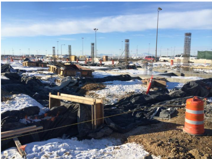
Column repair complete and footings ready to be re-formed Wednesday, December 31 st , 2014 3:14 pm
