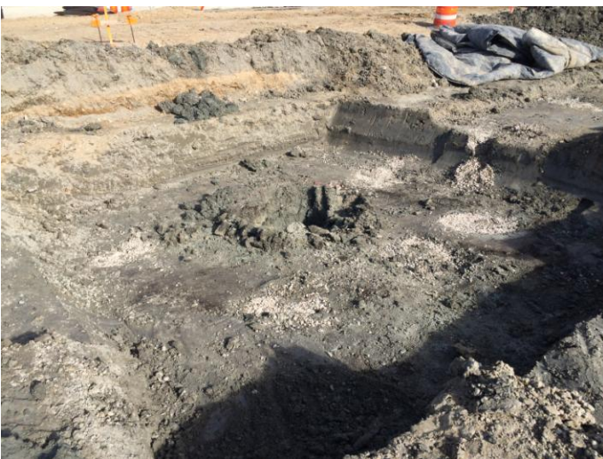
Example of small soft spot removal at top of stone columns in footing Thursday, December 4 th , 2014 11:42 am
