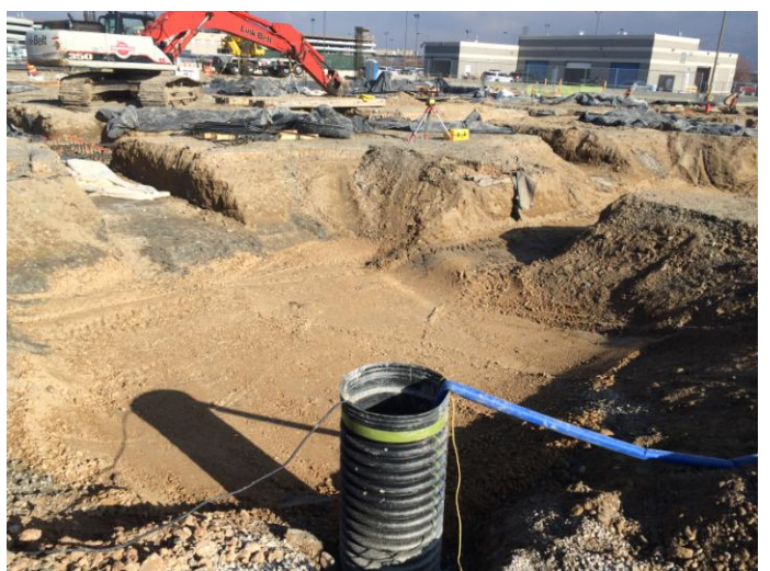
Flooded spot footing dewatered and filled with structural fill Thursday, December 10 th , 2014 12:01 pm
