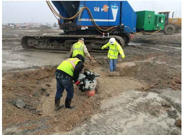
Preparing for a stone column "modulus" (load) test Monday, January 12 th , 2015 10:04 am
