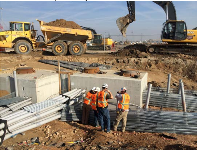
Power and communication vaults at northeast corner of QTA Friday, January 9 th , 2015 1:21 pm
