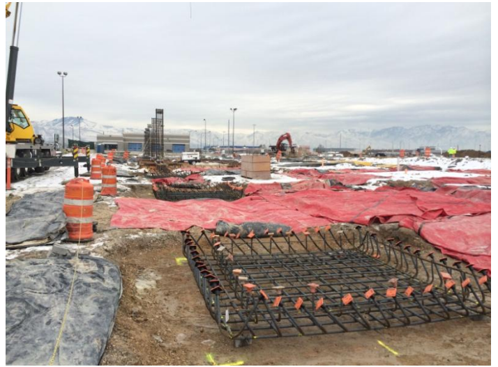
Rebar cages for footings near the north middle of the building Monday, January 5 th , 2015 11:26 am
