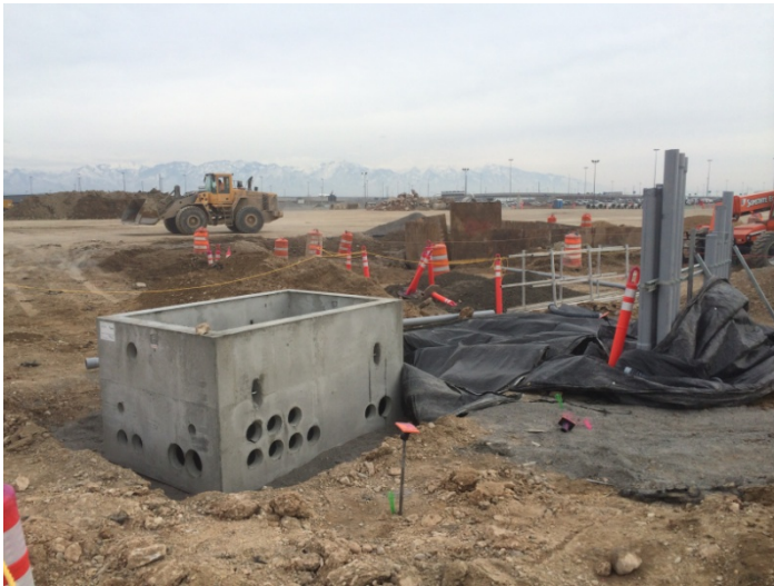
Electrical vault installed for QTA East Electrical Room Thursday, January 29 th , 2015 3:43 pm
