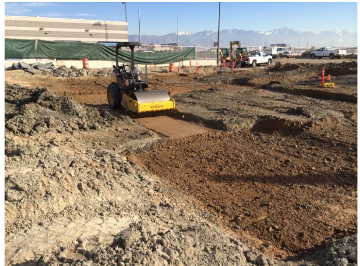
Compacting in spot footings & grade beams northeast corner Monday, December 8 th , 2014 2:07 pm
