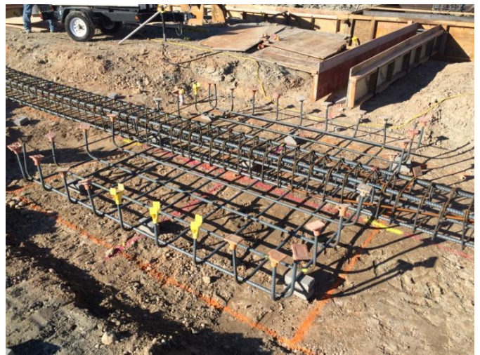
Grade beam rebar going through footing Wednesday, December 10 th , 2014 1:52 pm
