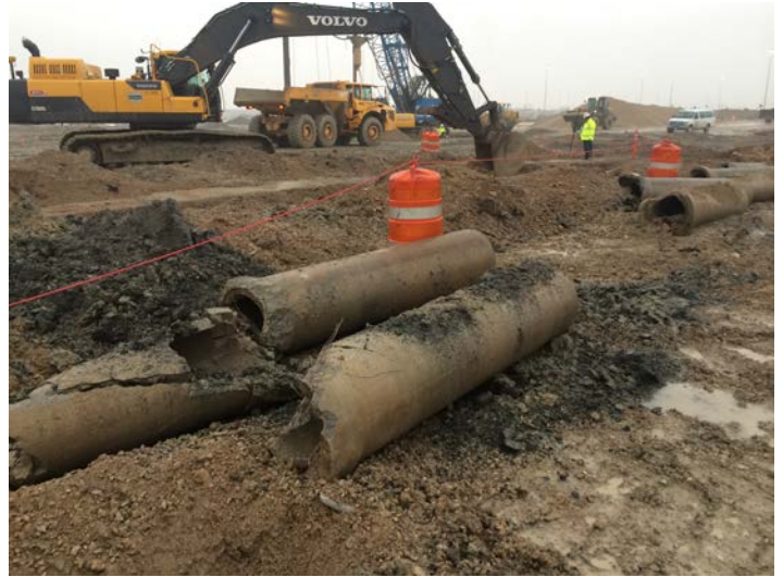
Old storm drain line removed in northeast quadrant Monday, January 12 th , 2015 9:57 am
