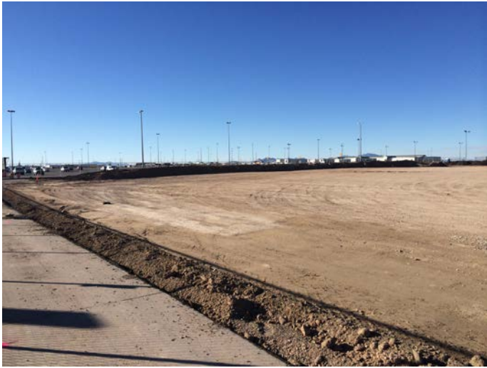
Grading of west half of site completed sw corner Tuesday, November 11 th , 2014 2:58 pm
