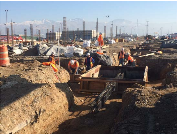
Formwork and rebar continues for footings and tie-beams Monday, January 26 th , 2015 10:39 am
