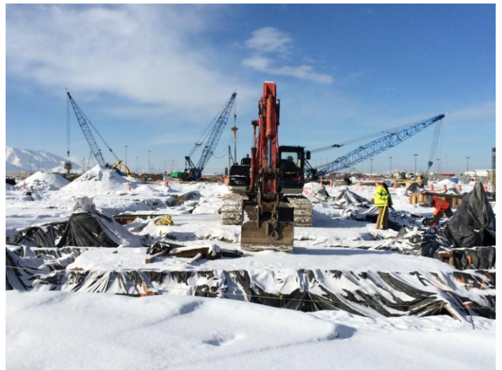
Wadsworth cutting out rebar to look for missing stone columns Tuesday, December 30 th , 2014 10:50 am
