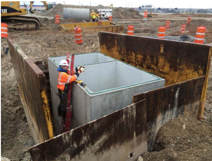
Oil/ Water Separator middle of east side of the QTA Wednesday, January 14 th , 2015 10:30 am
