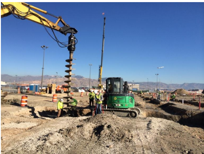
Stone column where the top had shifted being augered out to align with the bottom of the column so it can be re-built back up in the proper location Wednesday, December 10 th , 2014 1:58 pm
