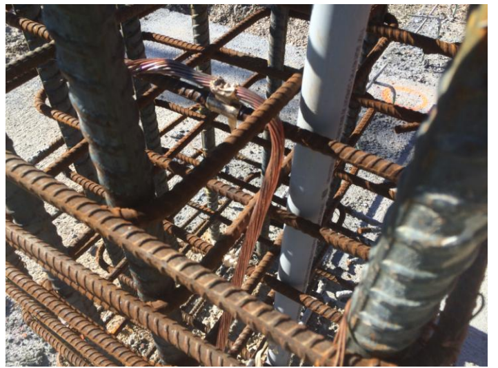
Grounding copper & lightning protection conduit Thursday, January 22 nd , 2015 11:50 am
