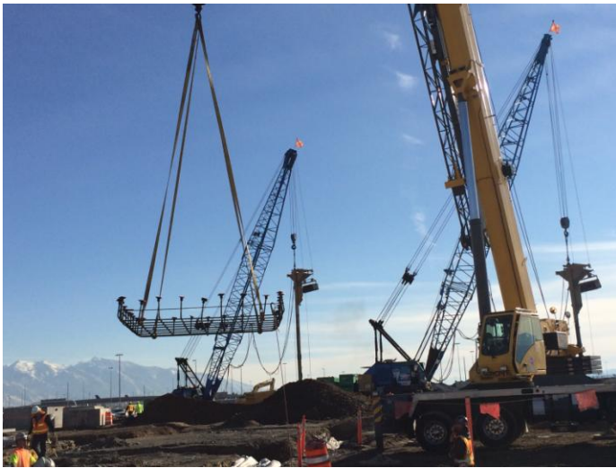
Rebar cage being lifted by the crane Monday, December 15 th , 2014 2:07
