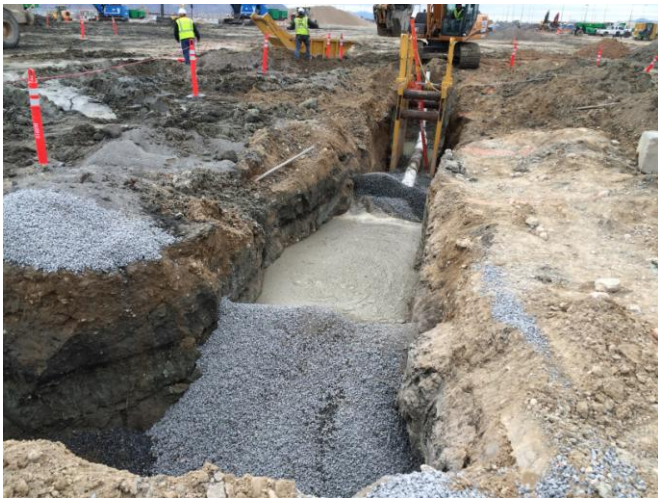
Flowable fill over drain pipe at NE corner Tuesday, November 24 th , 2014 2:54 pm
