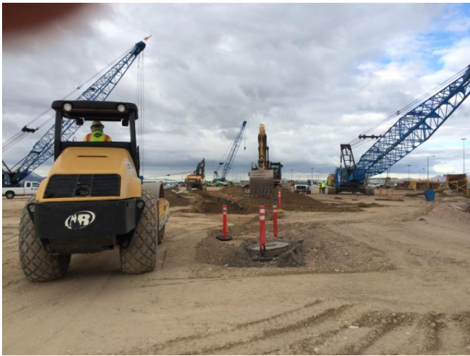
East/West ductbank removed & compacted Monday, November 3 rd , 2014 9:33 am
