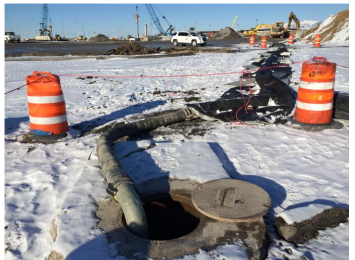
Routing the storm water around the hole for the new box Tuesday, December 30 th , 2014 3:00 pm
