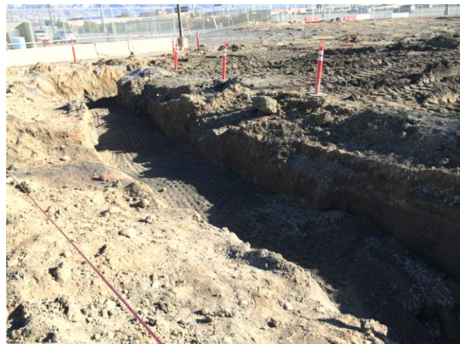
Storm drain pipe trench compacted at NE crnr of site Wednesday, November 26 th , 2014 2:00 pm
