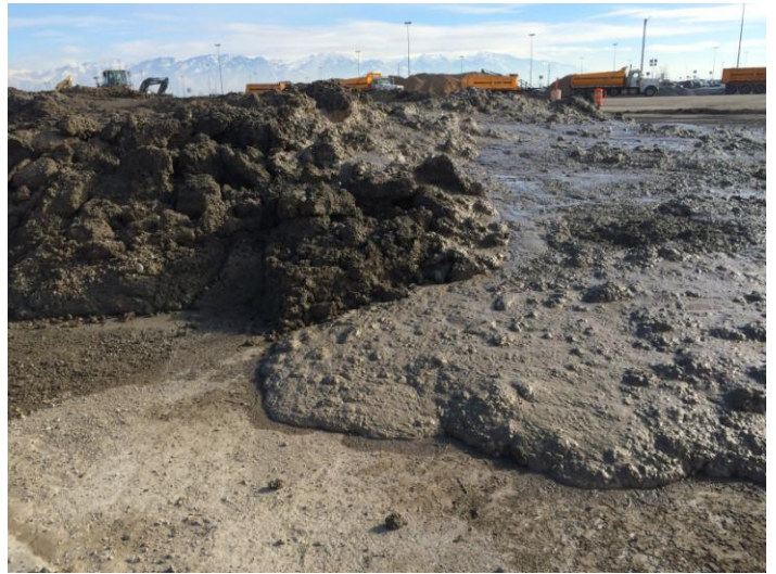
Mud from the holes for the stone columns Friday, January 23 rd , 2015 2:16 pm
