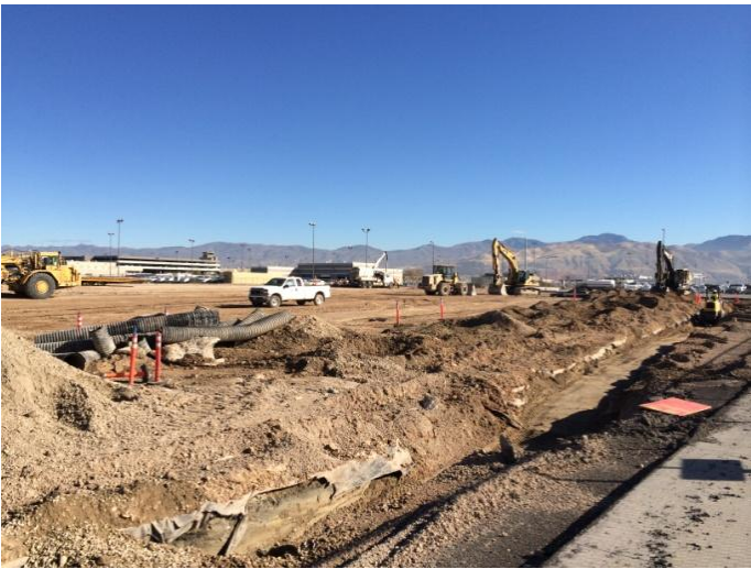
Corrugated Storm Drain Pipe removed and trench filled Wednesday, October 29 th , 2014 11:00 am
