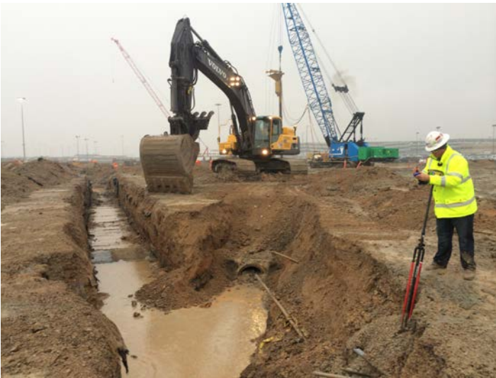
Storm drain line trench at the bottom of the "V" Monday, January 12 th , 2015 10:03 am
