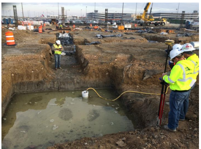
Checking a footing filled with rain & ground water day, December 9 th , 2014 8:59 am
