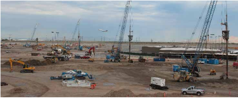
Cranes and crews worked over the summer to install 7,640 underground stone columns.
