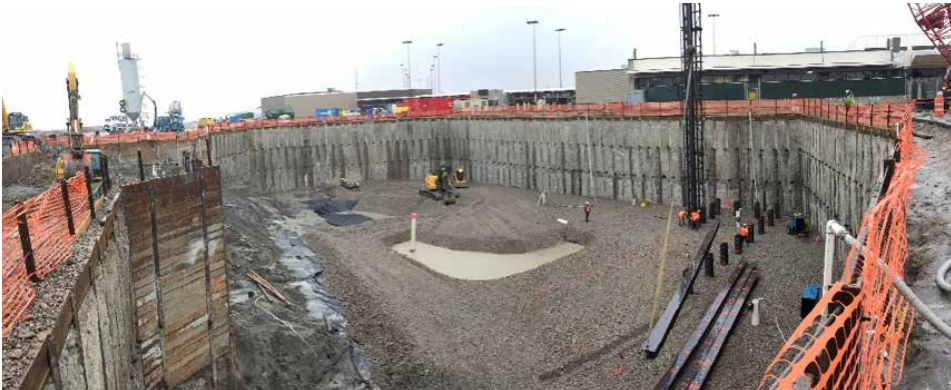
Construction crews work to drive the first steel pile in what will be the baggage processing tunnel.
