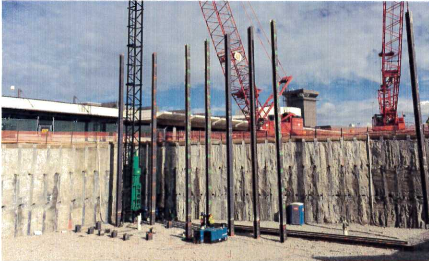
Driving Steel Piles for the Terminal Tunnel Deep Foundation.
