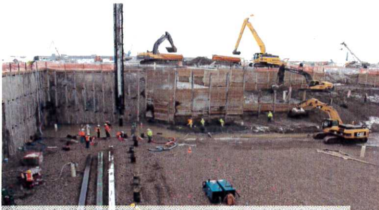
Working in the Hole
