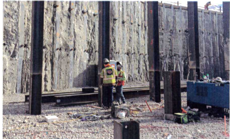
Foundation Piles are two 60' columns welded together driven to 120'
