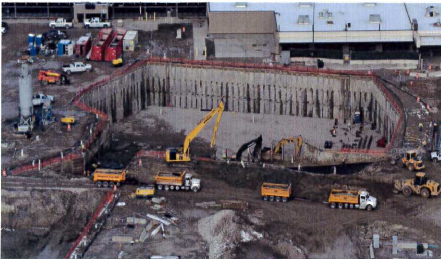
Terminal Tunnel Sequence 2 Area
