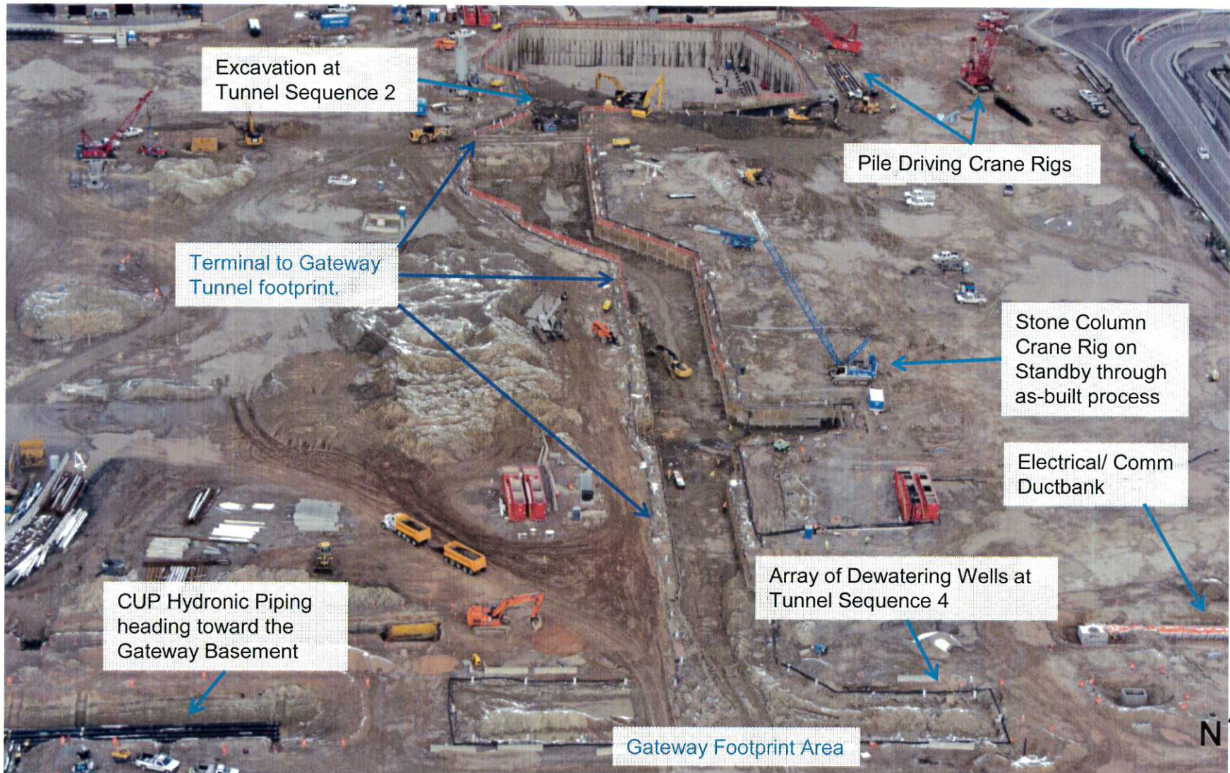
Terminal / Gateway Area
