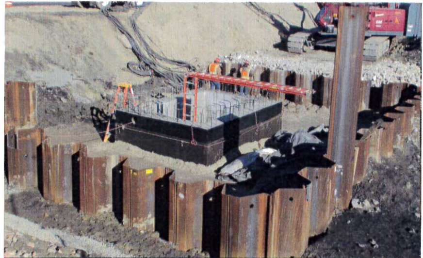
West Lift Station Wet Well poured and Waterproofed.
