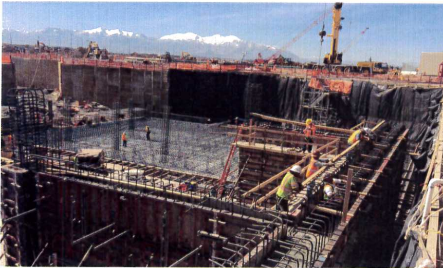
Final check atop the north wall form before concrete pumps.
