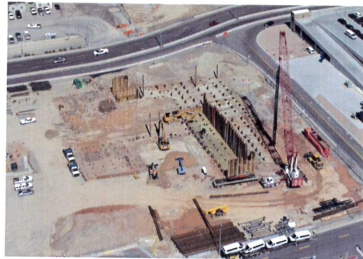
Central Utility Plant (CUP) Progress.
