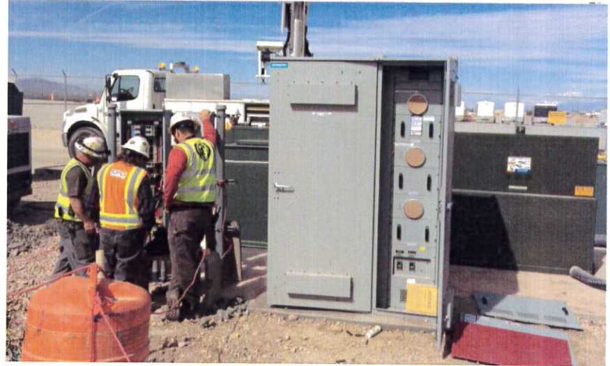
Power connection and meter installation for the West Lift Station.
