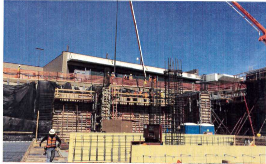
North wall pour in progress in the Terminal Basement.
