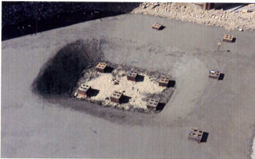
Piles and working surface mud slab in the Terminal Tunnel.
