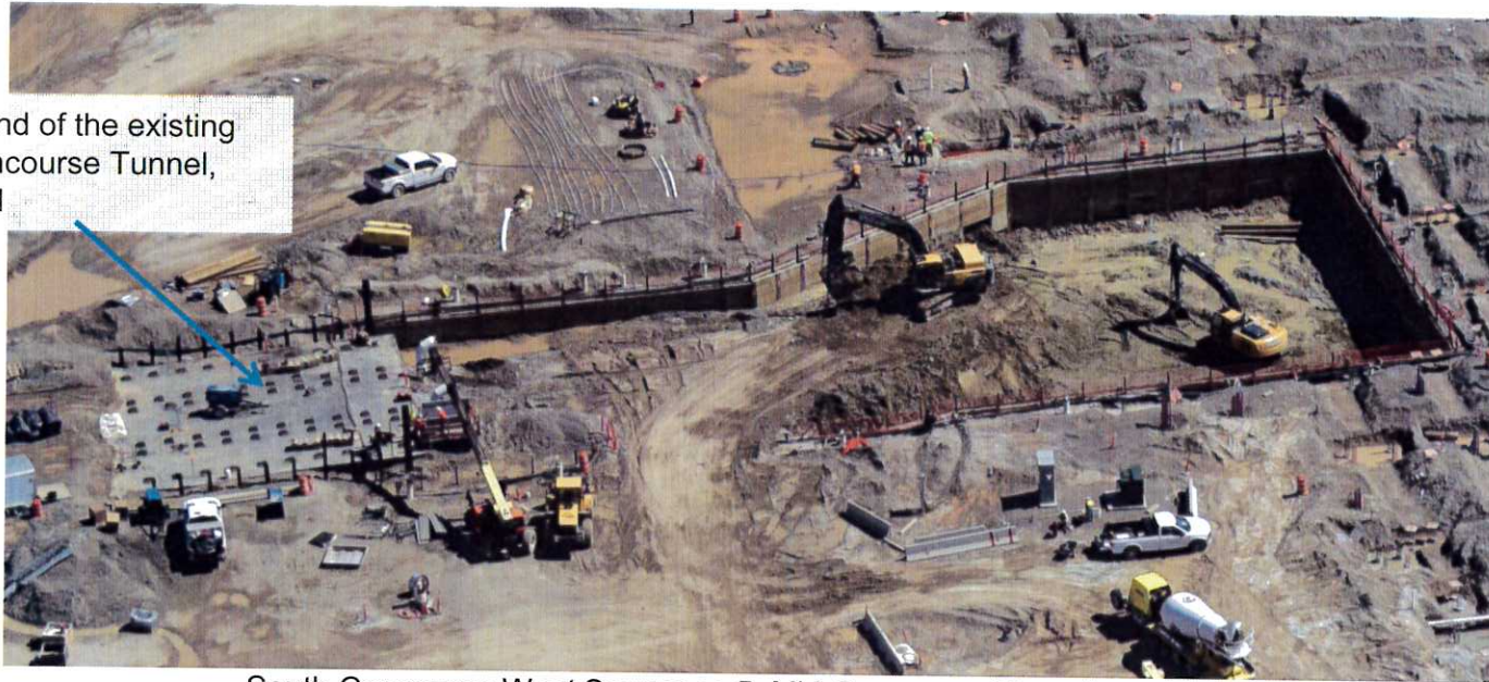
South Concourse West Sequence 5, Mid-Concourse Tunnel excavation
