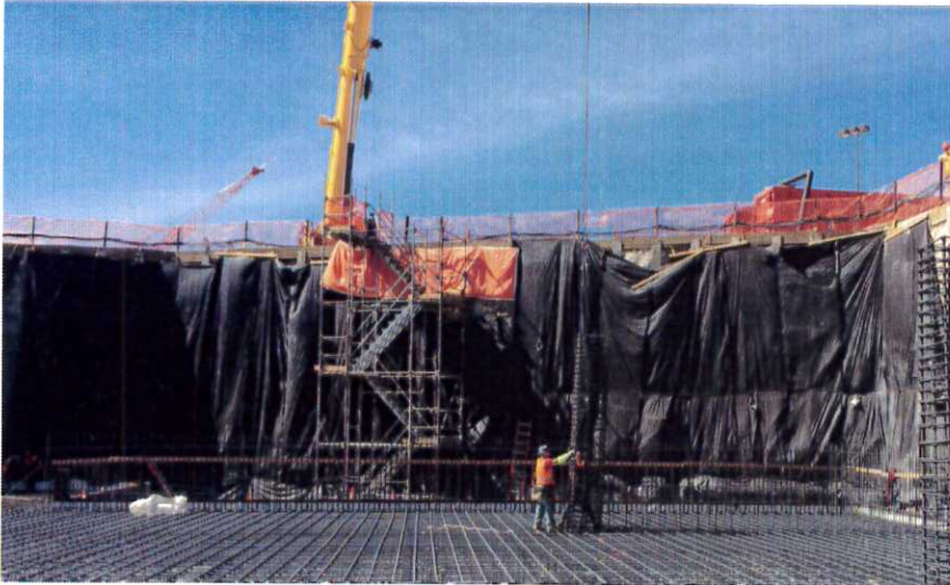
Setting column rebar on the Terminal Basement floor slab rebar.
