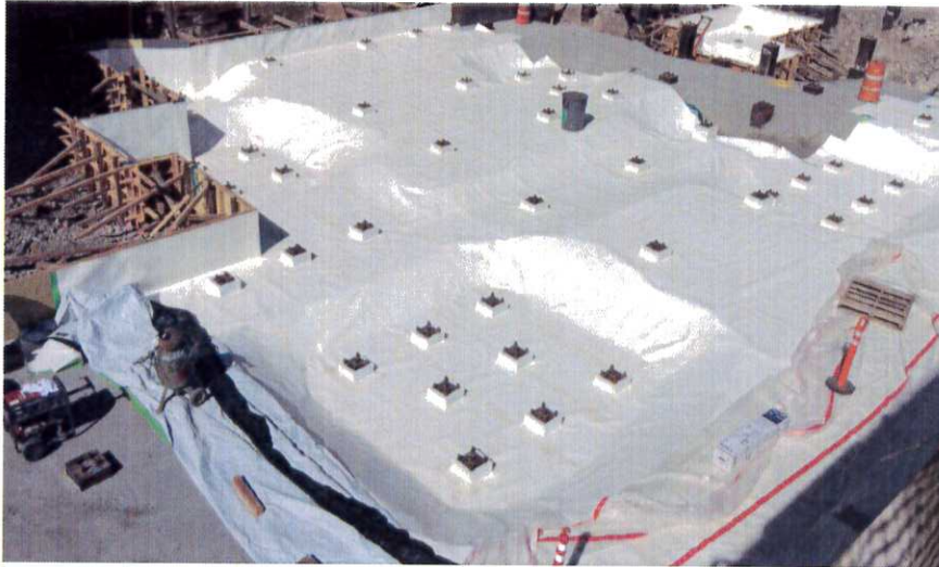
Waterproofing application in the Terminal Tunnel.
