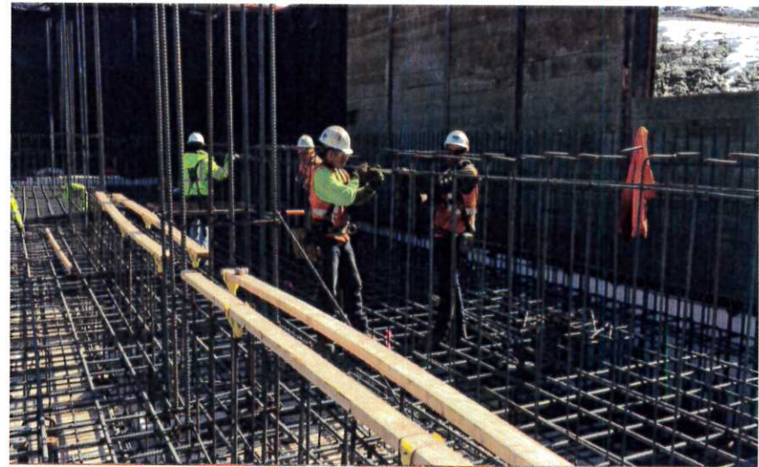
Tying rebar for Terminal Basement starter wall.
