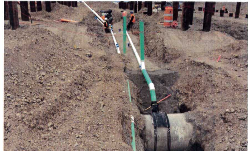
By now, underground utility installations can be measure in miles.
