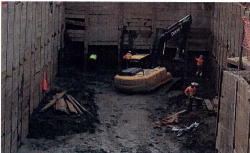
Excavation and lagging crew working their way out of Gateway Tunnel Sequence.
