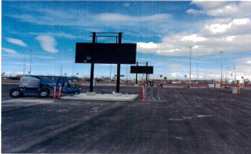
FIDS installed at Park and Wait Lot.
