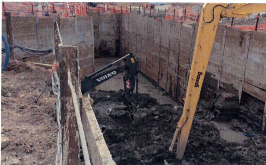
Excavation and wall lagging nears completion in Tunnel Sequence 4.
