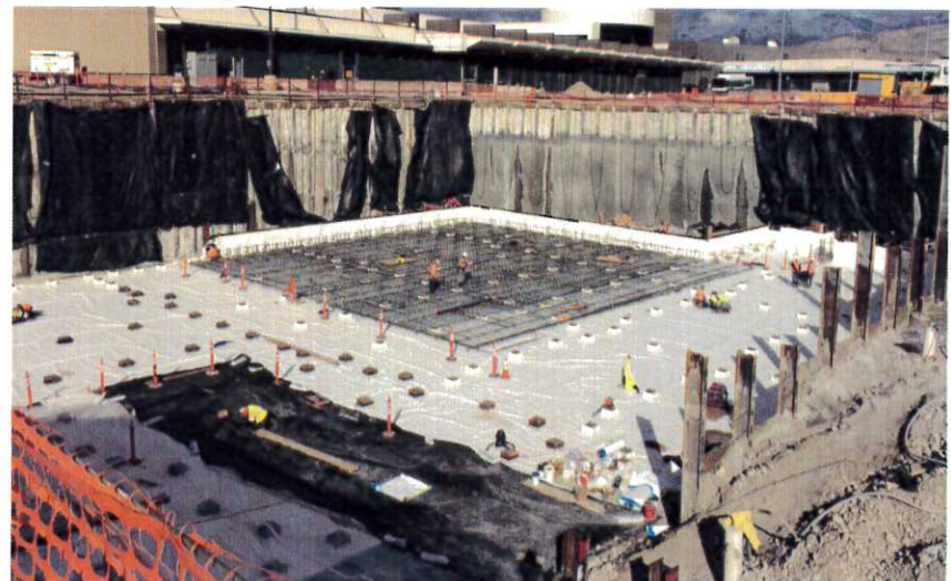
Placing the first course of rebar on waterproofing for the Terminal Tunnel mat slab pour.
