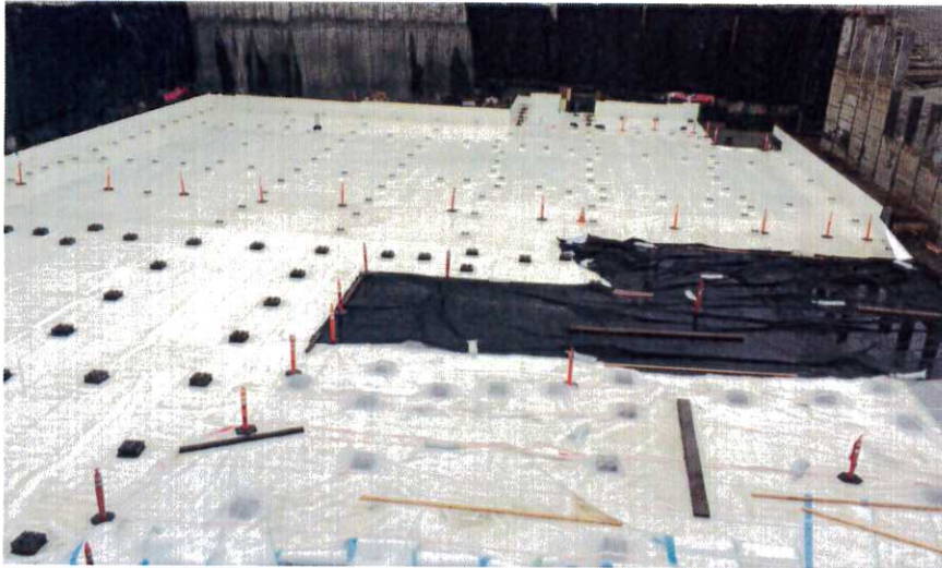
Waterproofing application on the mud slab in the Terminal Tunnel.
