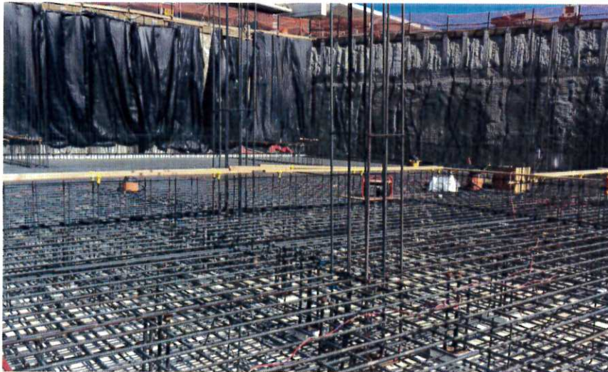
Rebar in progress for Terminal Basement floor slab pour.
