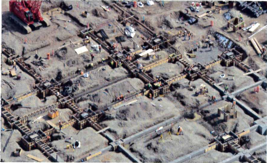
South Concourse West Foundation detail.
