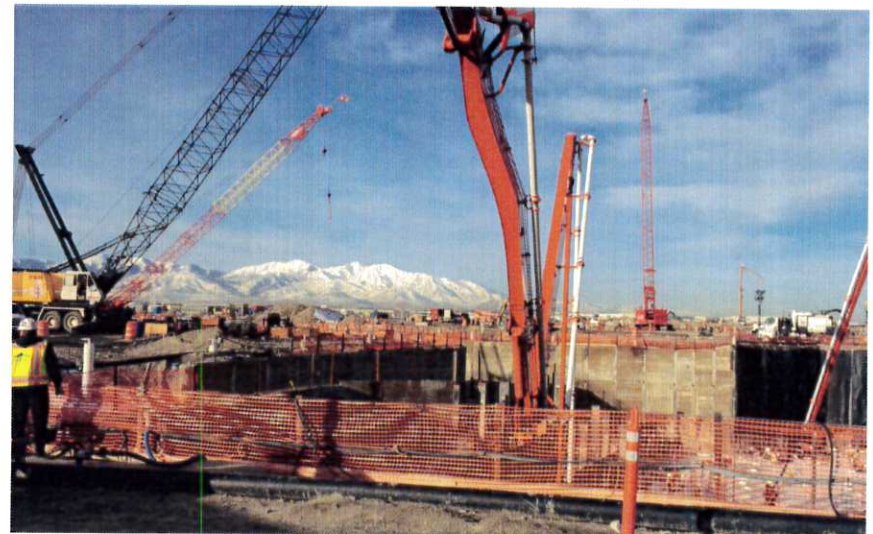
Cranes and concrete pumps at the Terminal Tunnel.
