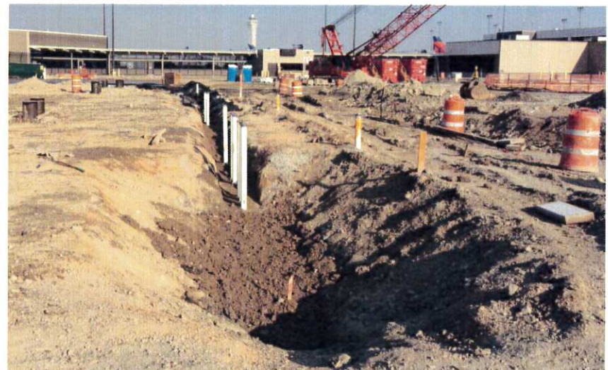
Under-slab piping installation at South Concourse West.
