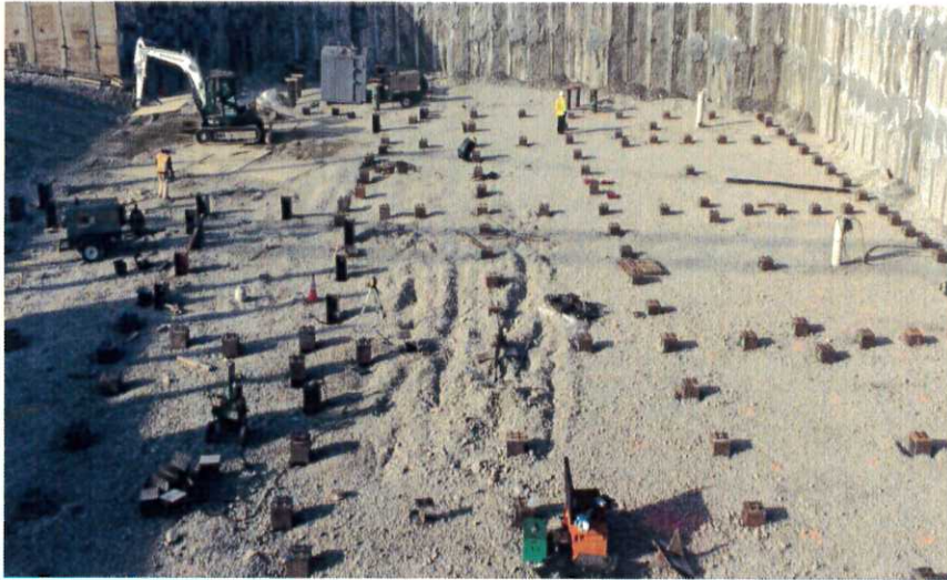
H-pile, many cut and capped, installed in the Terminal Basement.
