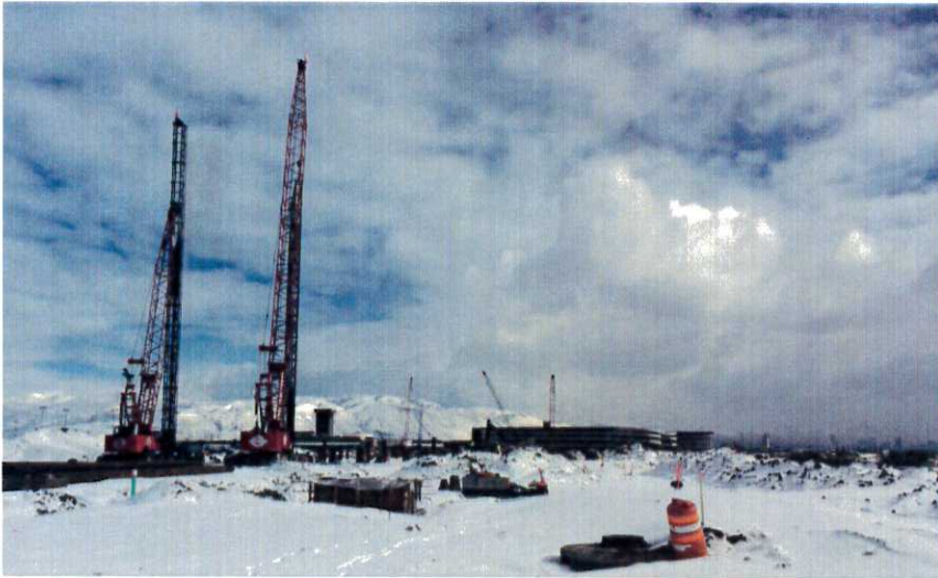
Cranes at work on the South Concourse West building pad.
