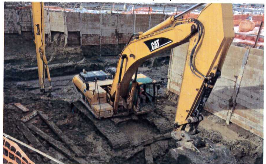
Terminal Tunnel excavation and lagging at Tunnel Sequence 1.
