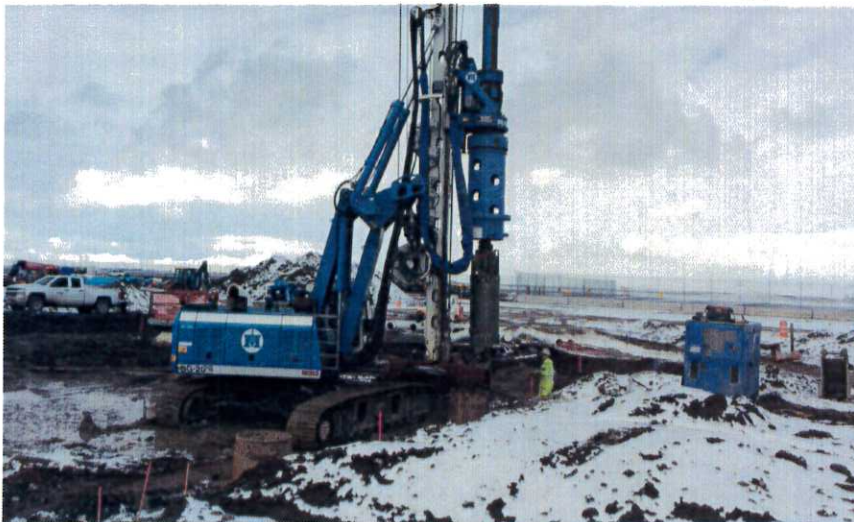
Drilling dewatering wells at existing Airfield Tunnel Sequence 5.
