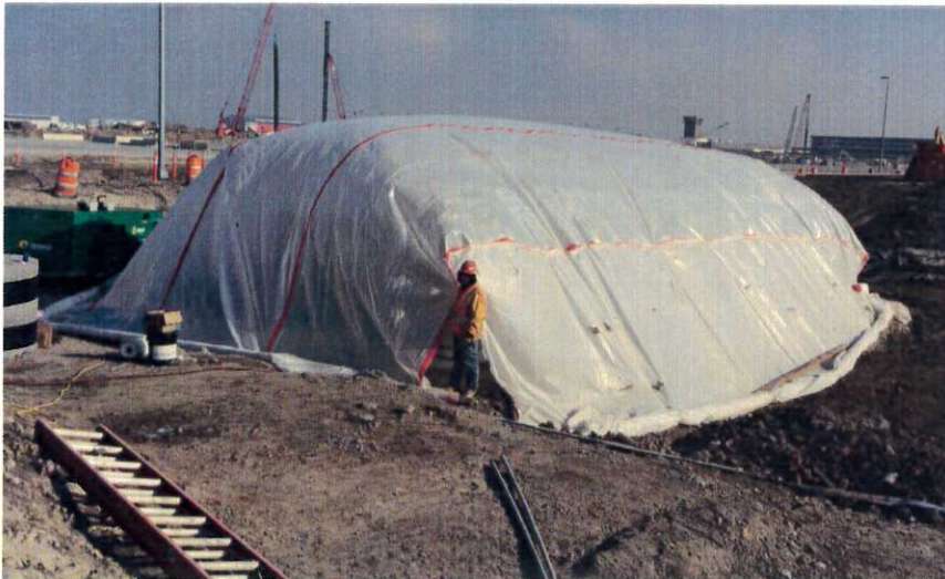
Heated shelter allowing West Lift Station waterproofing application and curing.
