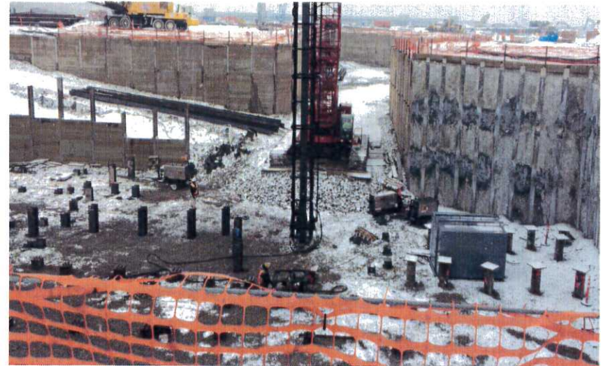
Pile driving crane rig working its way out of Tunnel Sequence 2
