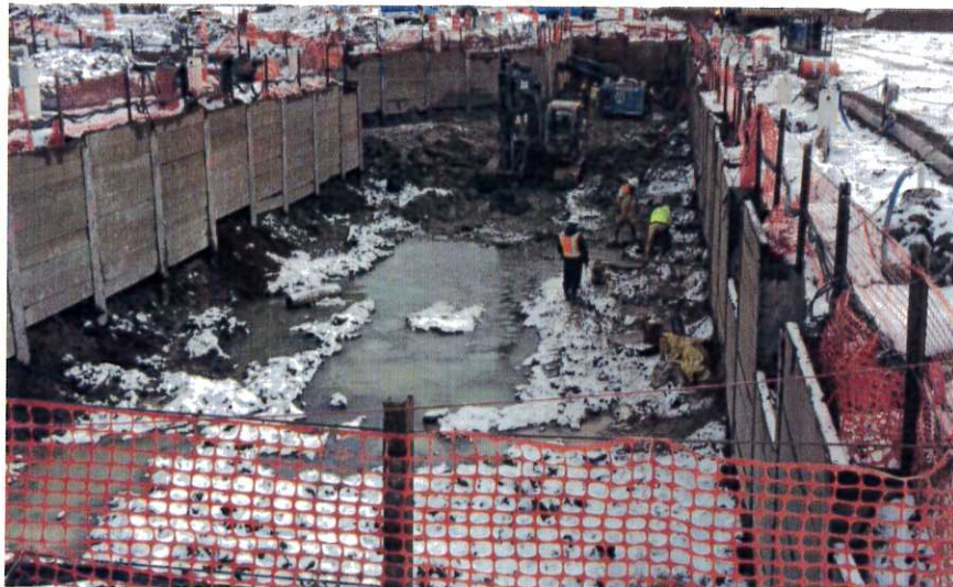
Excavation and wall tie-backs continue in Tunnel Sequence 4.
