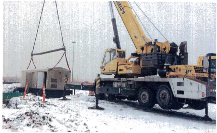
Setting West Lift Station and pumps on structure.
