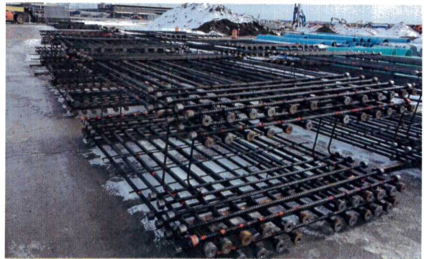
Pre-tied rebar for South Concourse West pile caps
