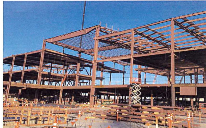
Erecting Terminal Roof Trusses at Canyon.
