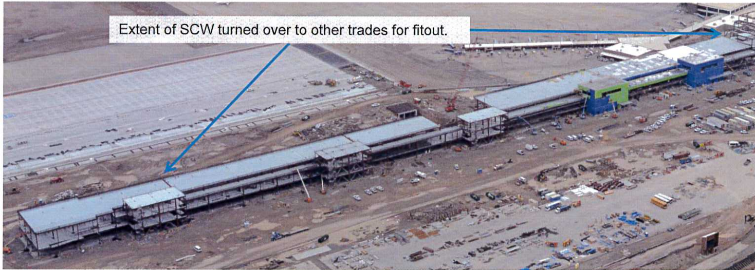
SCW construction progress
