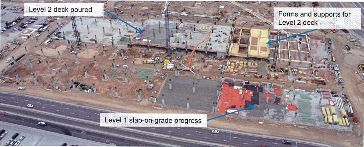
Parking Garage progress
