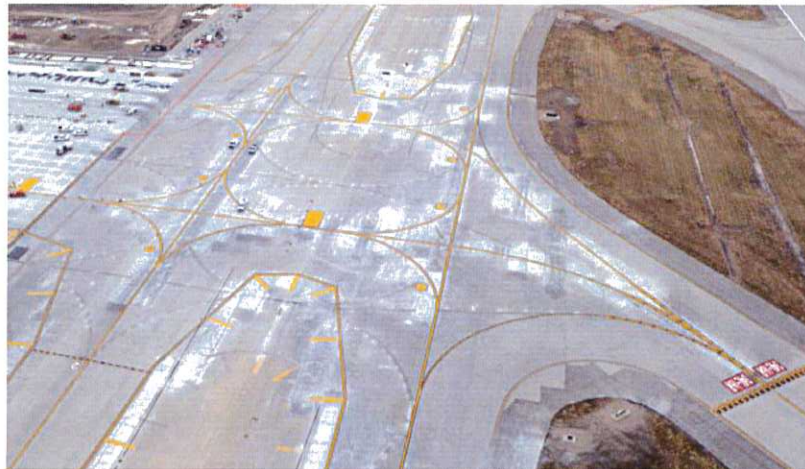
New striping at Taxiways A and B, and Ramp A5.
