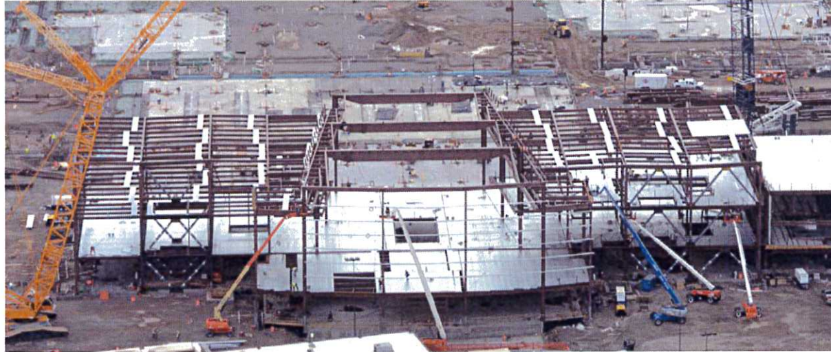
Terminal steel and metal deck progress, viewed from the north
