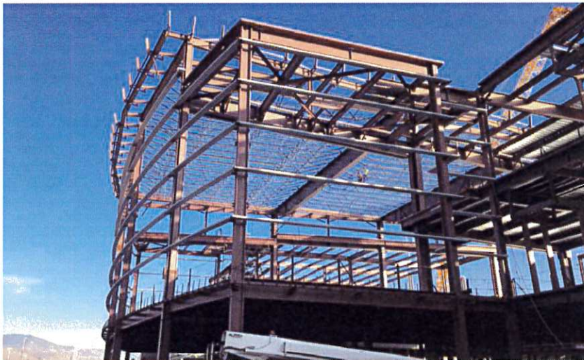
Erecting Terminal Roof Trusses at Canyon.
