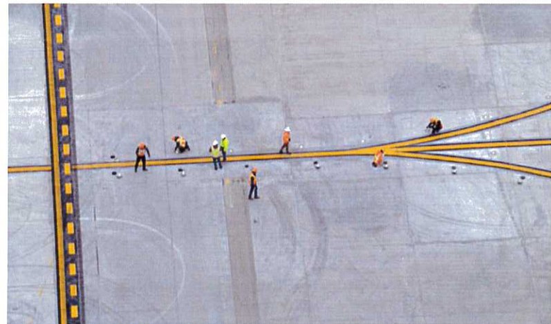
Electricians installing new LED centerline lighting.
