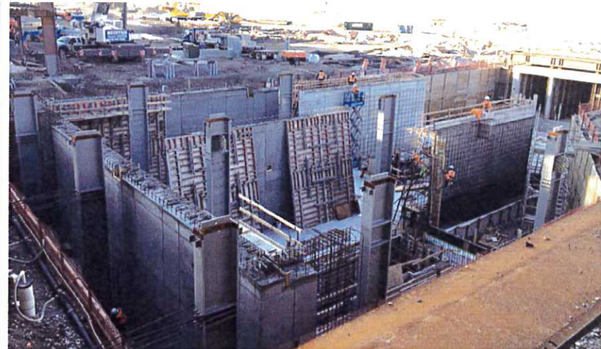
Slab and wall progress at Mid-Concourse Tunnel
