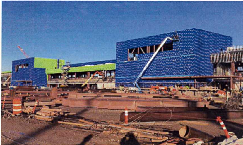
SCW exterior wall sheathing progress
