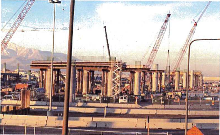
Elevated Roadway bent cap progress
