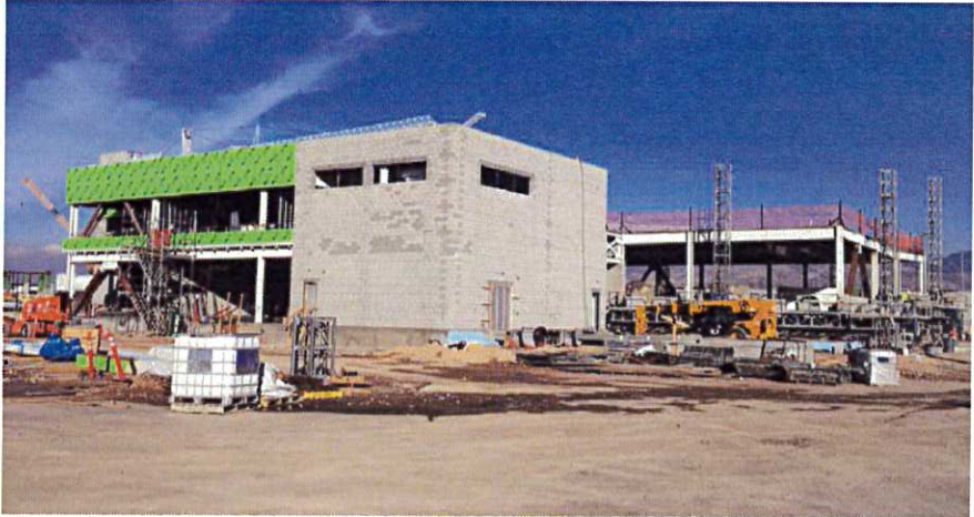
Central Utility Plant (CUP) building progress
