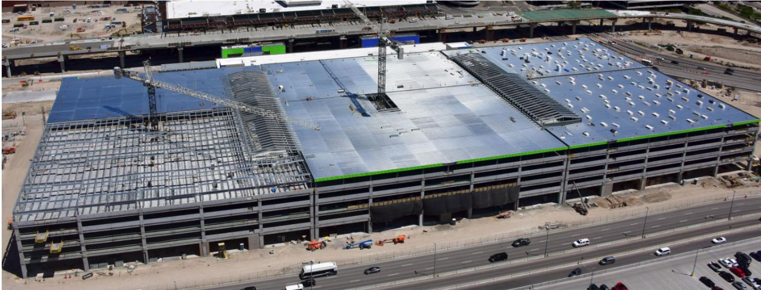
Parking Garage - looking north – Roof Steel Erection and Metal Decking
