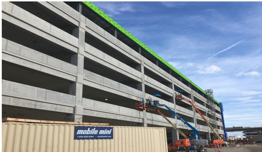
Parking Garage east face, rubbing concrete and removing forms
