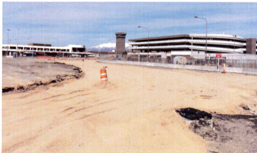
Terminal Exit Roadway Detour Construction
