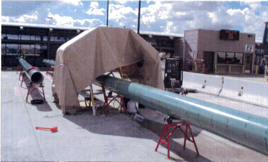
Fuel line weld x-ray test inspection set-up
