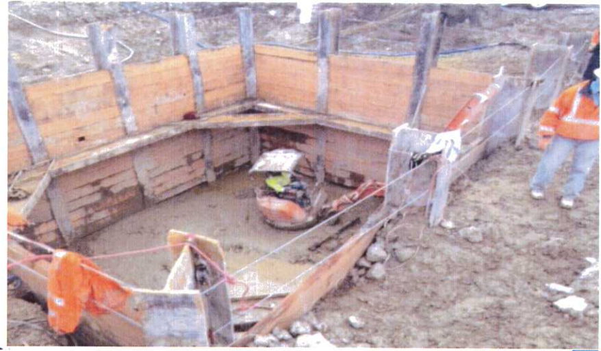
Aerial of East Lift Station Site
