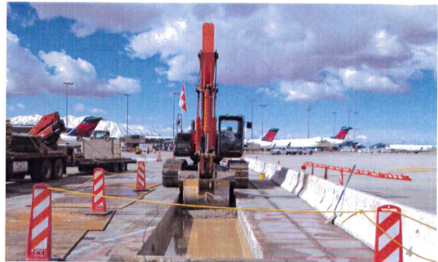
Airfield fuel line relocation trenching in progress at Gate D2
