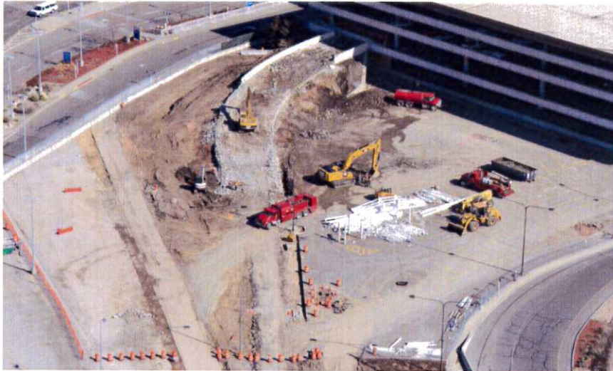
Demolition of the Parking Deck West Ramp
