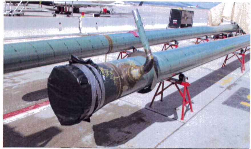
Close-up of fuel line pipe assembly
