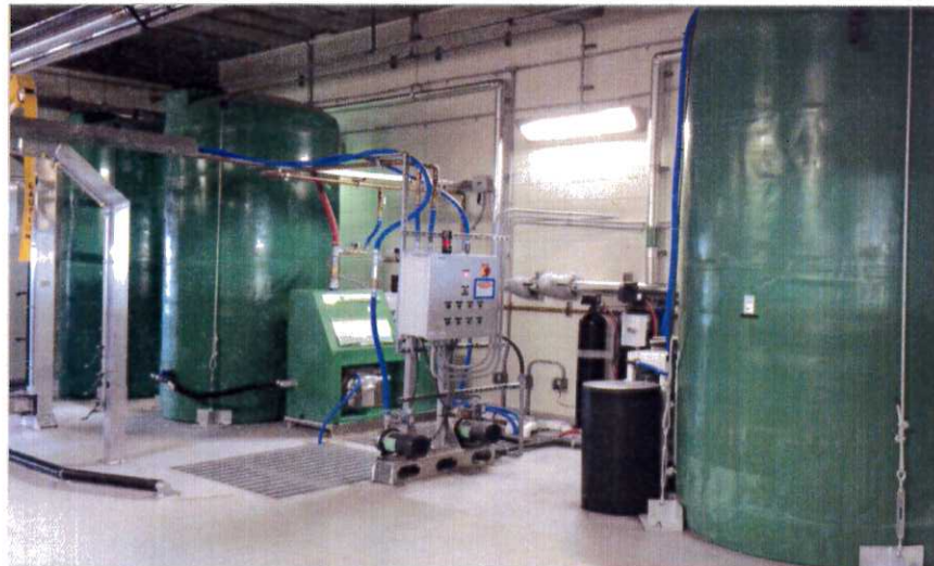
QTA car wash equipment installation
