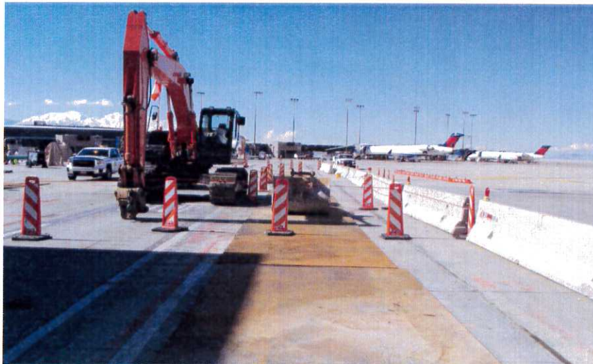
Airfield fuel line relocation trench covered during off hours
