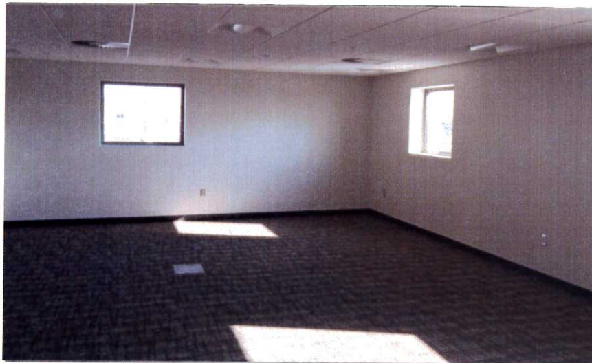
Interior Progress in RSS 'B'
