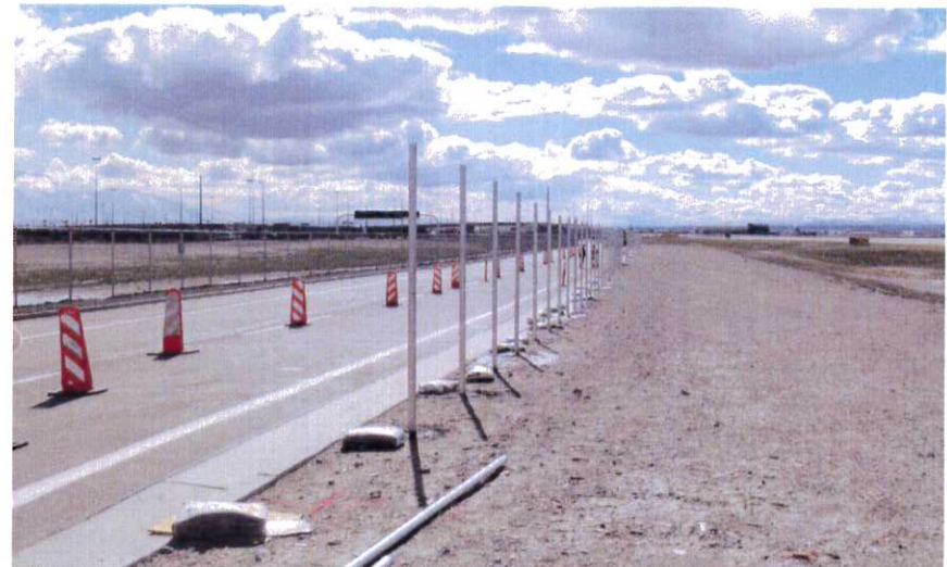
West Access Road temporary SIDA fence installation progress
