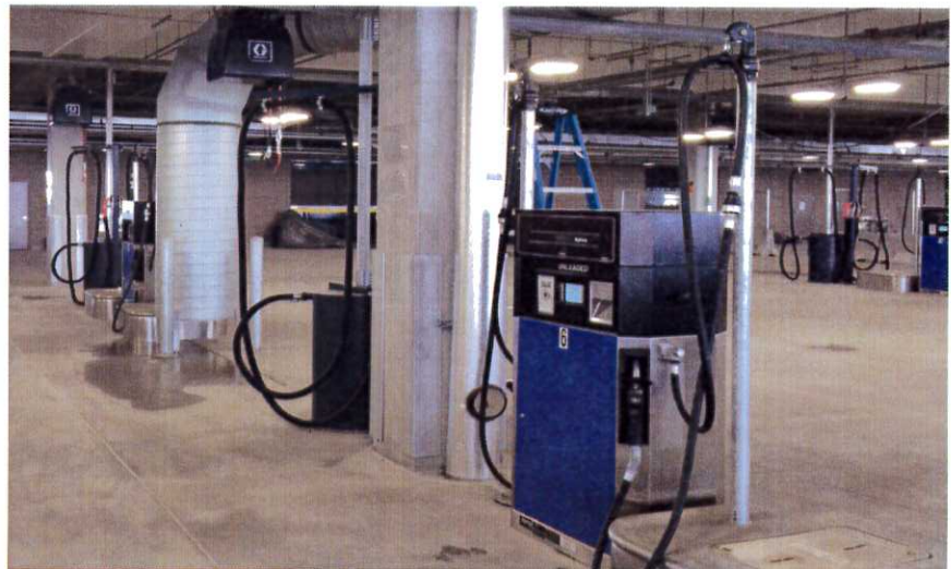
Typical QTA car care station. Fueling, vacuum system, and compressed air and wiper fluid from the hose reels
