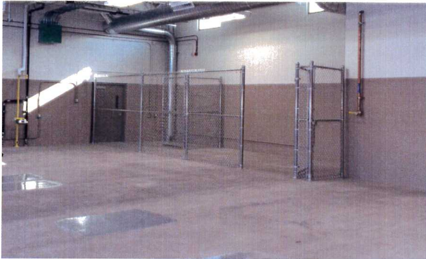
RSS 'C' Work Bay tenant parts storage cage
