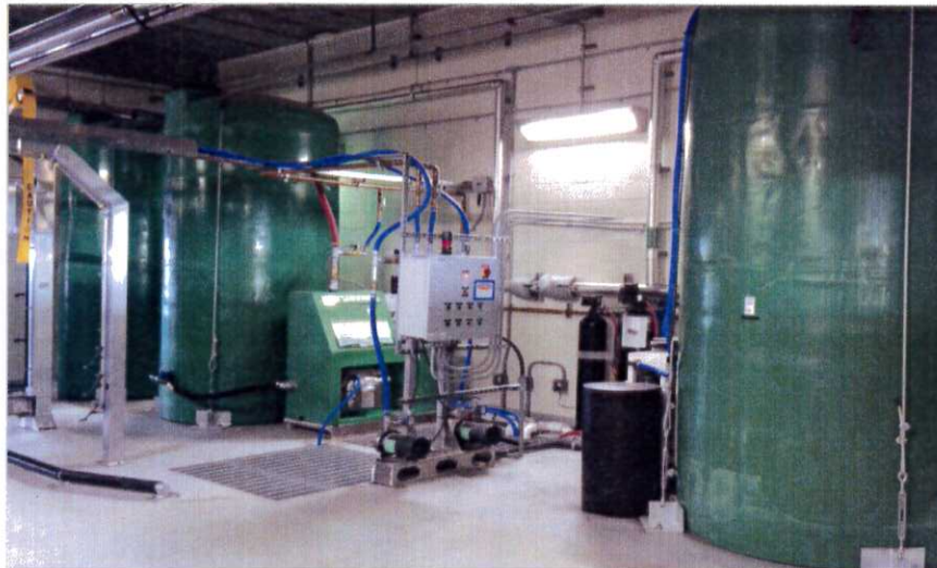
QTA car wash equipment installation
