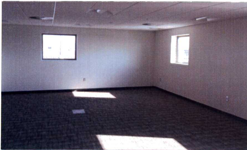
Interior Progress in RSS 'B'
