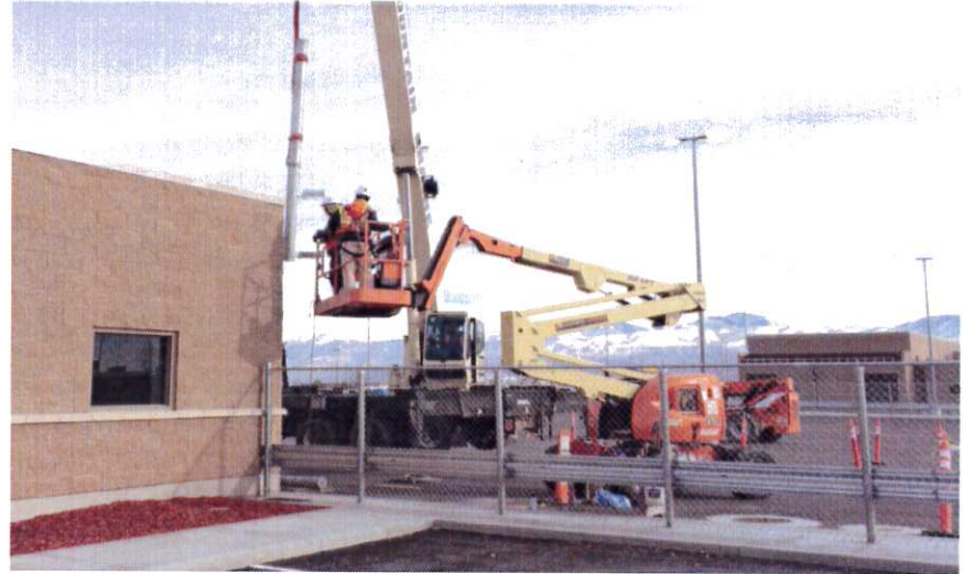
Mounting corner camera pole at RSS 'B'
