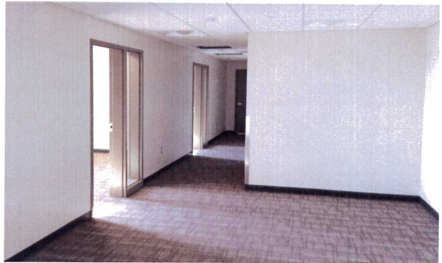
Admin Area Progress in RSS 'C'
