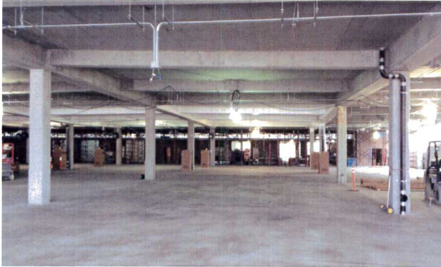
QTA west side stacking area looking toward the fueling area
