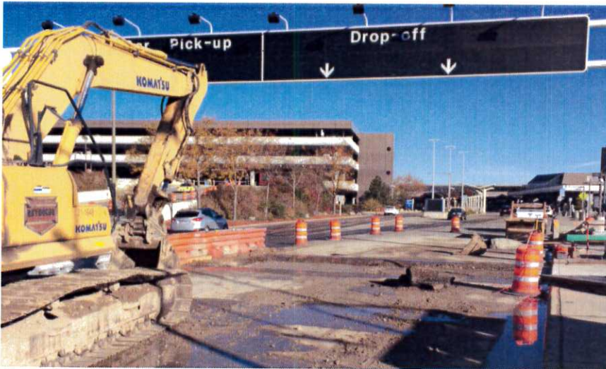
Sanitary line for new East Lift station crossing Main Entrance road
