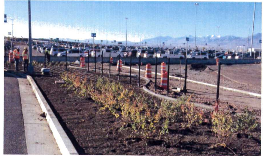
QTA/RSS road landscaping, irrigation and fence installation
