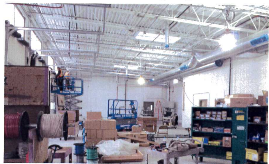
HVAC and Electrical installation progress in RSS 'C' Work Bay
