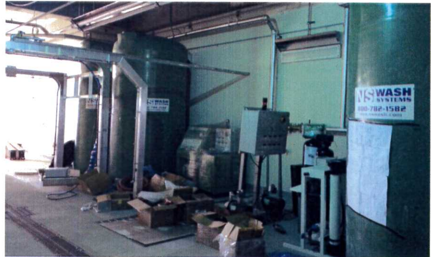
Start of QTA carwash equipment Installation
