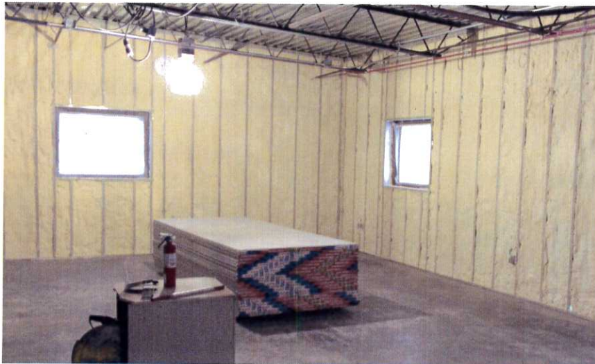
RSS 'B' Admin area build-out, exterior wall insulated, sheetrock ready
