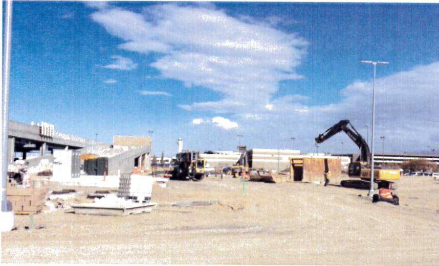
Significant amount of sitework in progress at QTA-east side
