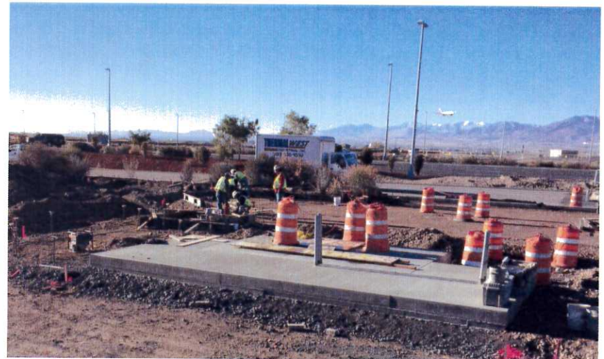
South Lift Station wet well poured, forming generator slab and curb
