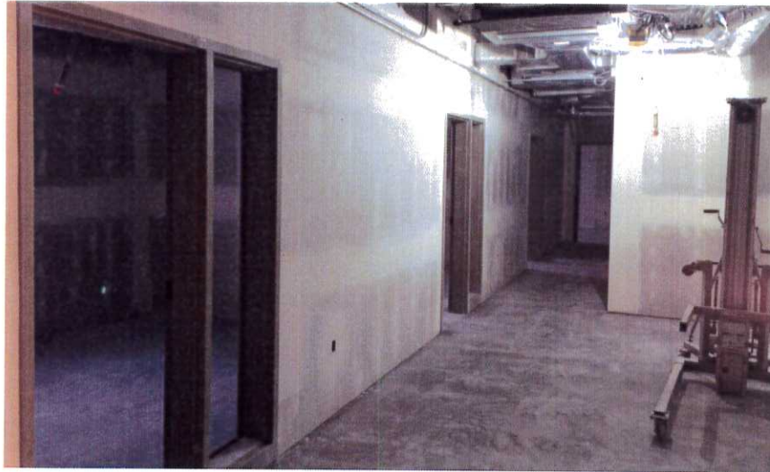
RSS 'A' Admin Area, walls taped & sanded, frames primed
