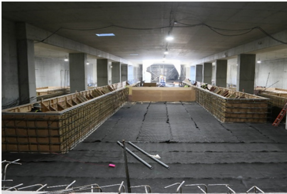
Passenger circulation cell in the Central Tunnel taking shape.
