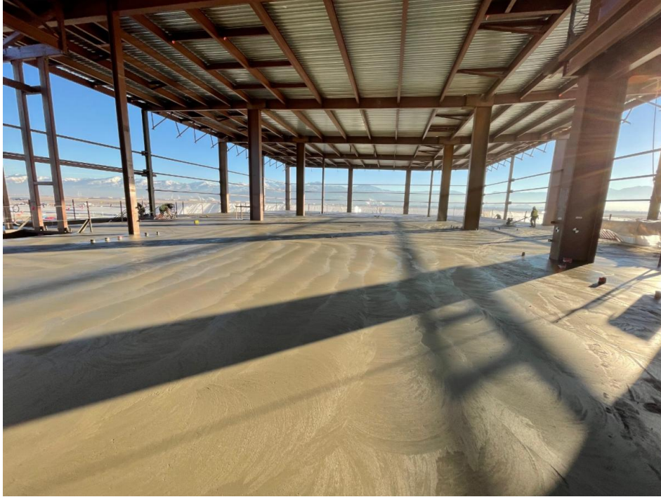
Final concrete pour on level two of Concourse A-east.
