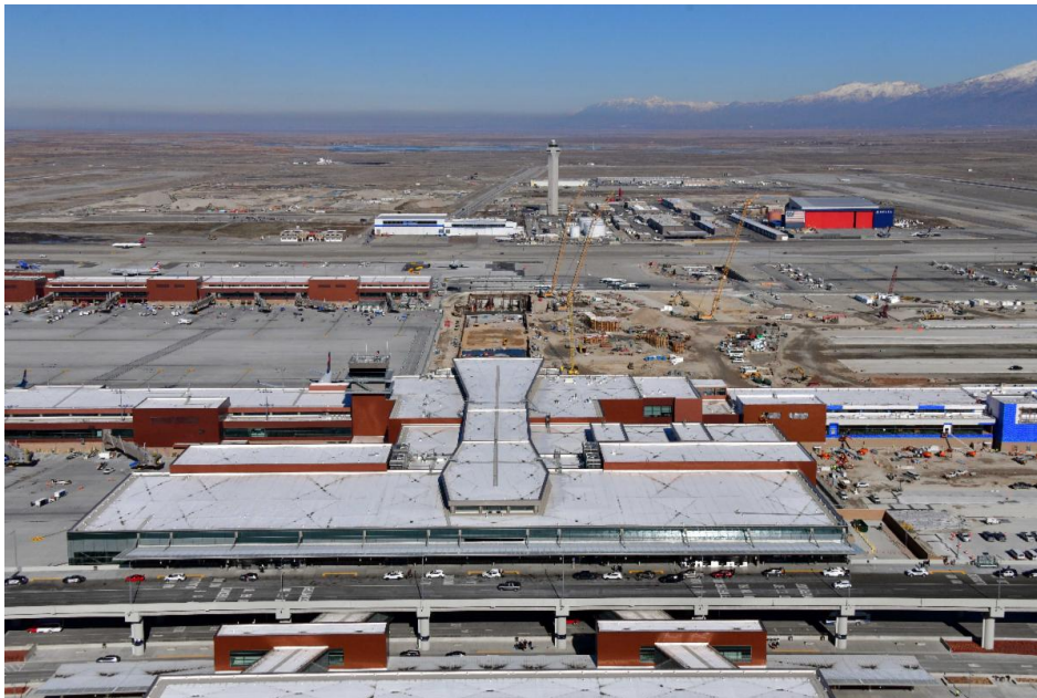
Aerial view of the terminal and central tunnel, looking north.
