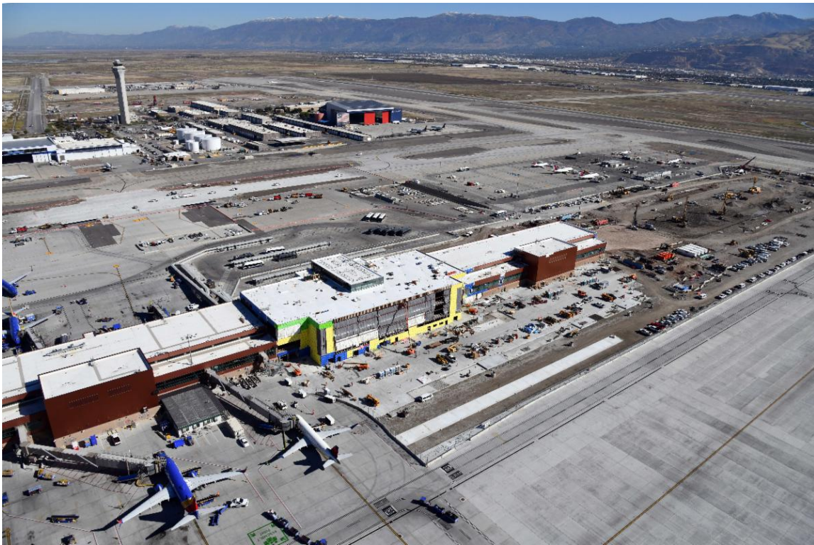
Aerial photo showing the construction of Concourse B-east, looking northeast.
