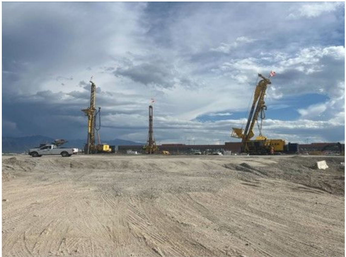
Started installing stone columns for Phase 4
