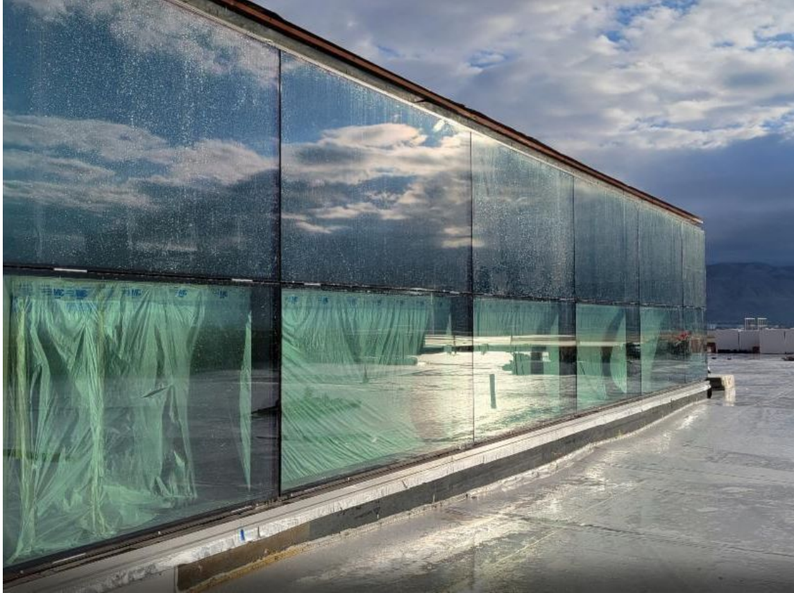
The clearstory penthouse on Concourse B-east, following glass installation.
