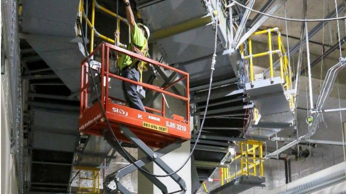
Installing the baggage handling system catwalk in the Central Tunnel
