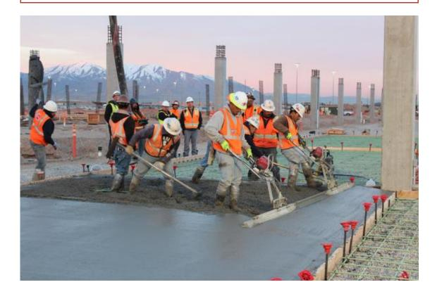
The Quick-Turn-Around (QTA) facility that car rental companies use to clean, refuel and circulate cars remains the construction focus of the Terminal Redevelopment Program. In the area south of the parking garage, crews are now pouring the concrete floor. Relocation of the QTA is one of the enabling projects that will prepare the site to accommodate the new terminal anticipated to be finished in 2019.
